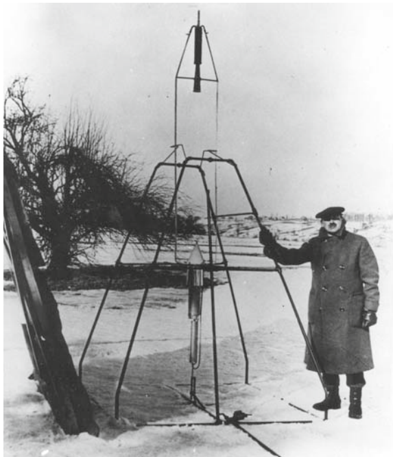
Fig. 1.5 Robert Goddard with the first successful liquid-fueled rocket, March 16, 1926. The device used gasoline and liquid oxygen propellants (courtesy NASA)
