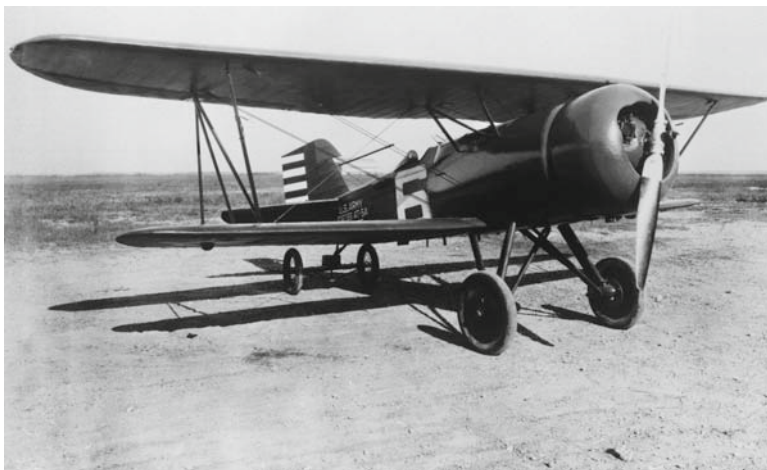
Fig. 7.1 Early airplanes used performance-enhancement devices such as multiple wings to increase lift and aerodynamic cowlings to decrease drag. This is the Curtiss Hawk with NACA cowling (courtesy NASA)
