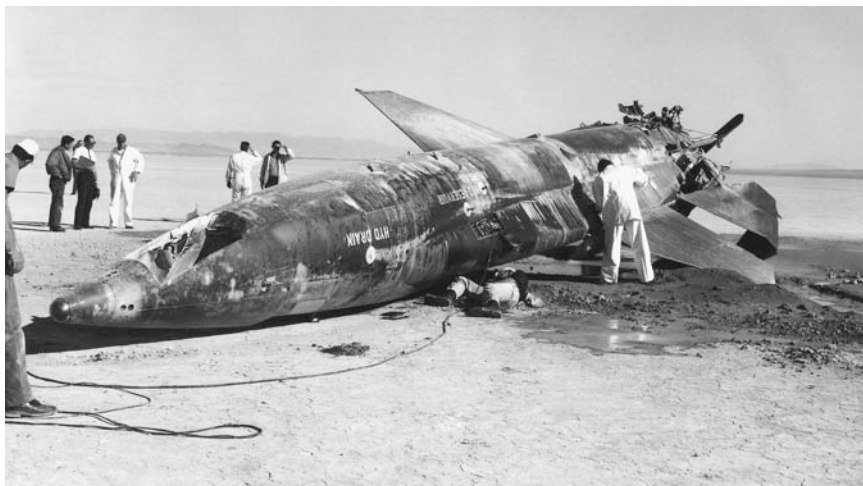
Fig. 5.7 On November 9, 1962, X-15 pilot Jack McKay experienced multiple vehicle failures, forcing a crash landing. After the engine became stuck at 35%, the planned flight test was aborted. Landing flaps then failed to extend, resulting in a higher than normal-speed approach, and the left skid failed on touchdown, causing the vehicle to tumble. Yet because this vehicle had wings and direct human control, both plane and pilot flew again (courtesy NASA)
