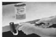
4. After strip is positioned, apply pressure immediately with J-roller. Be careful near the ends so you don't break the laminate.
