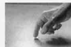
9. A surface is ready for bonding when adhesive does not transfer to your fingertip.
