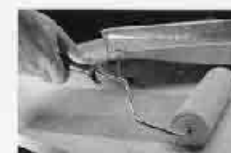
8. Next, apply adhesive to the core (particleboard or old surface) with roller. Make sure both surfaces are free of dirt.
