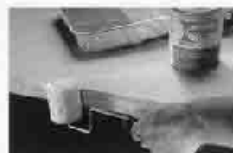
2. Next, apply two coats of adhesive to core edge of countertop.
