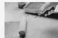
7. Apply adhesive to the back of the laminate with a roller. Follow adhesive instructions.
