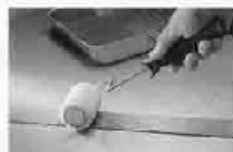
1. Start with the self-edge. Apply Formica brand #100 adhesive (or equivalent) to the laminate edge strip with small roller or brush.
