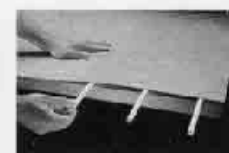
10. Position dowel rods approximately 6" apart to support laminate and keep it off the core as you align. Slide rods out after laminate is positioned over core material.
