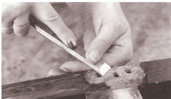
Fig 31 Hold the chisel steady, sliding it between index finger and thumb to stop it slipping
