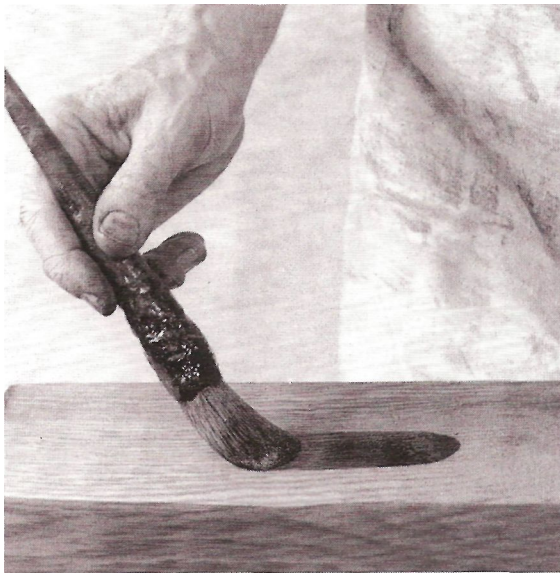
Fig 89 Coat colour evenly in strips across the full width
