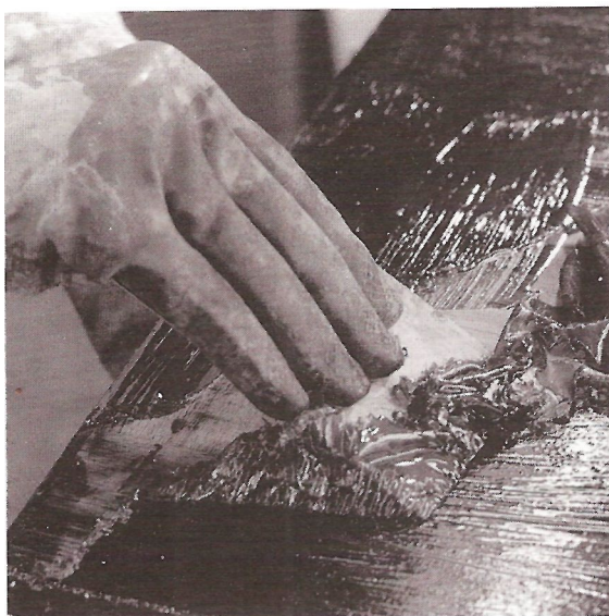
Fig 23 Use a sharp scraper to remove all the material
