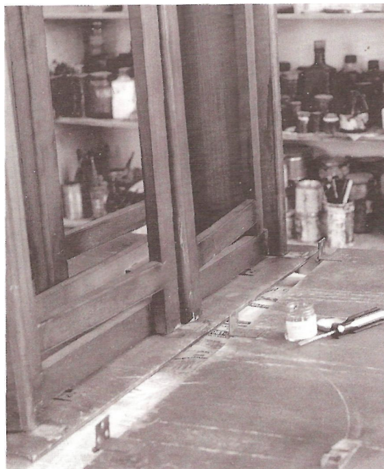
Fig 17 The hinges remain on the leaf and all the fittings are put into a labelled jar
