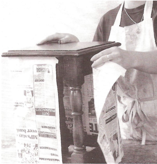
Fig 18 Masking up the base if you only want to strip the top
