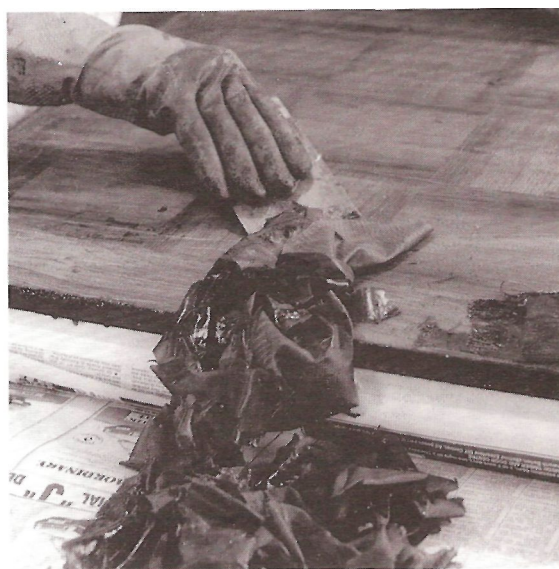
Fig 24 Scrape off onto a piece of paper which can be disposed of later
