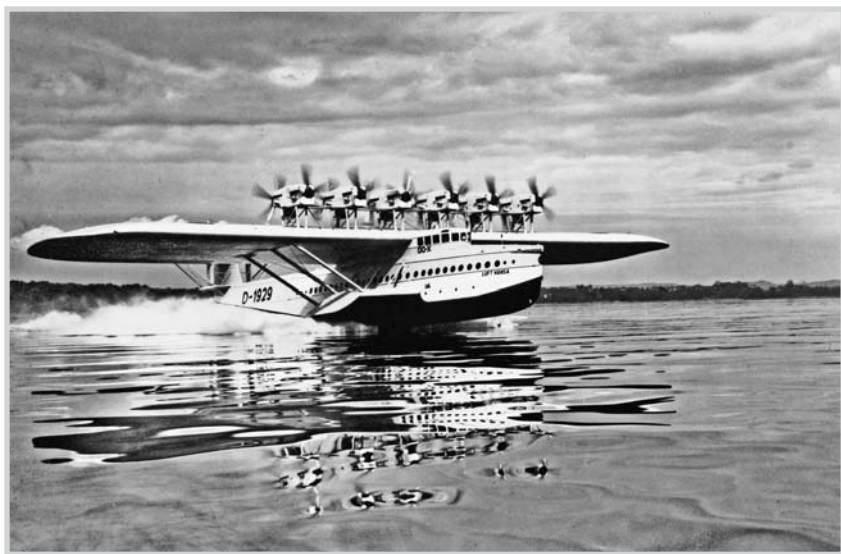
Too heavy, the Dornier Do X of 1929 performed poorly despite twelve engines.
