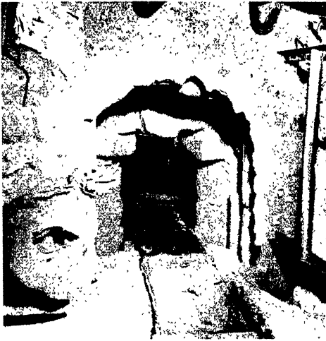
Three photographs of the great French chapel tunnel: (above) electric light was installed and (below) a cable system for transport of debris; the solidity of some of the masonry which had to be pierced is evident (left)
