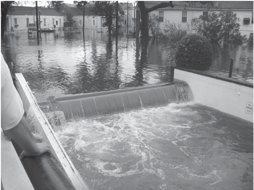
Like a waterfall, flood waters cascade over a barrier to the loading dock of Lindy Boggs Medical Center. The waters flooded the hospital basement, which housed supplies and equipment, the kitchen, the pharmacy, and the morgue. Photo by Pablo Moncada.
