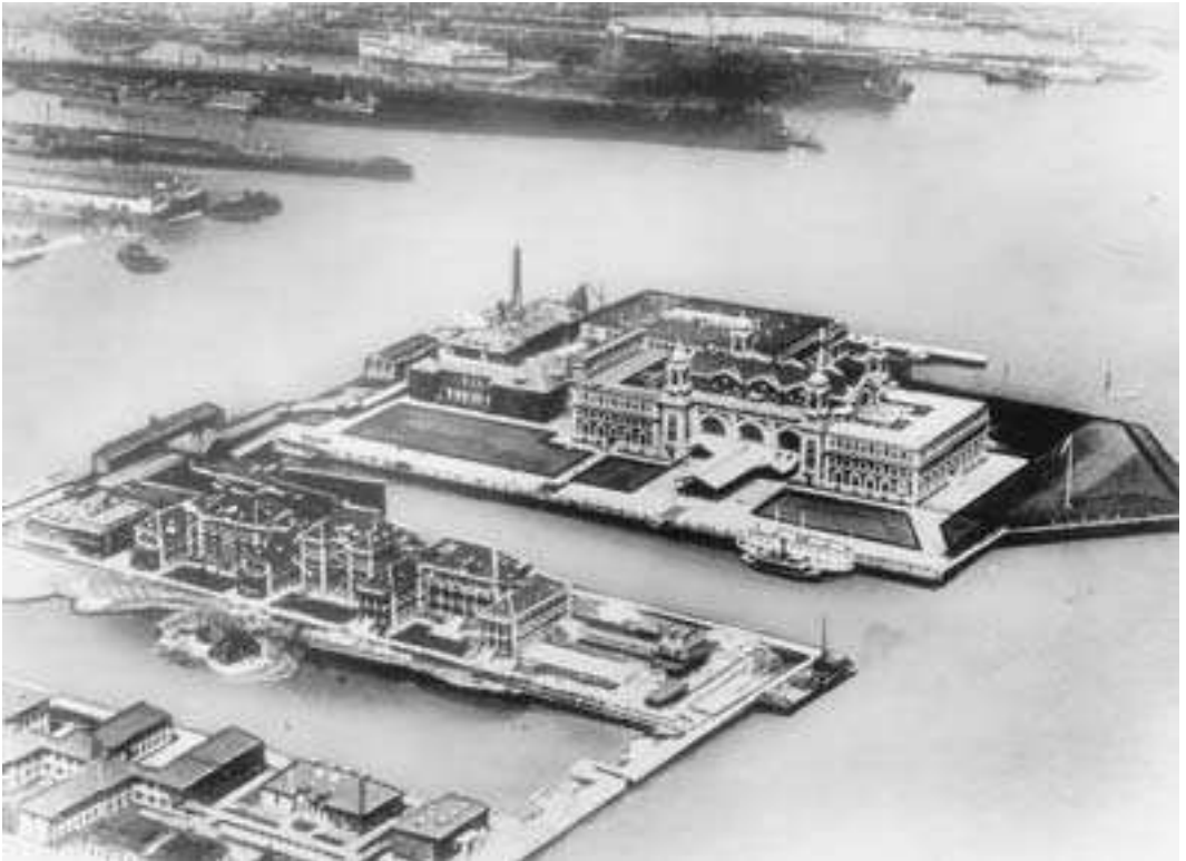
Aerial view shows the effects of landfilling at Ellis Island, ca 1915. Courtesy of the Ellis Island Immigration Museum.
