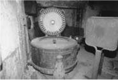
Laundry and Linen Exchange/Hospital Outbuilding interior today. Courtesy of the Ellis Island Immigration Museum.
