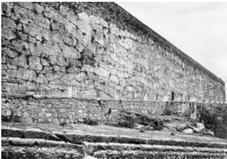
Figure 10.6: Polygonal walls of the Alatri Acropolis, Italy.
