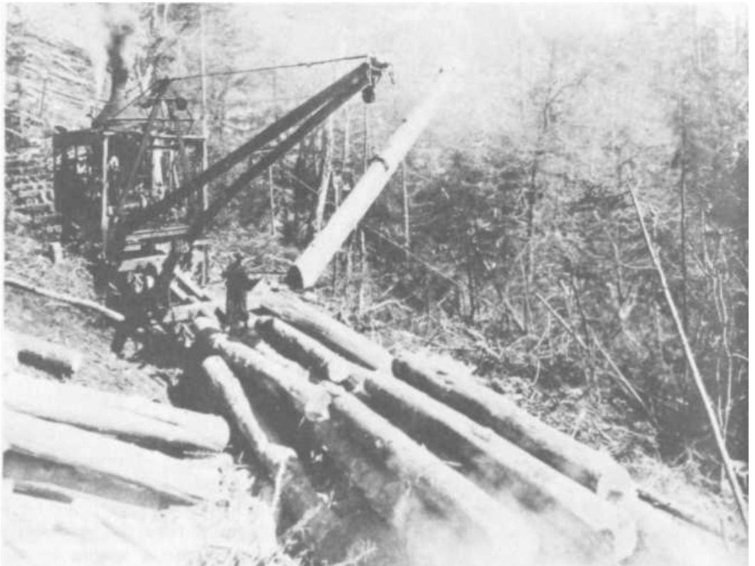
PLATE 278 A "stiff-necked" loader at work. The loaders were steam powered, and their boilers were often called "coffeepot boilers." (Photo courtesy of Champion Paper.)
