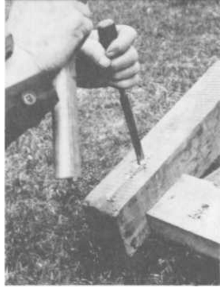
PLATE 169 After the bottoms of the pegs are sawed off flush, Tedra splits the bottom of each peg. Then he drives a wedge into the split to make the peg bind firmly in the hole.
