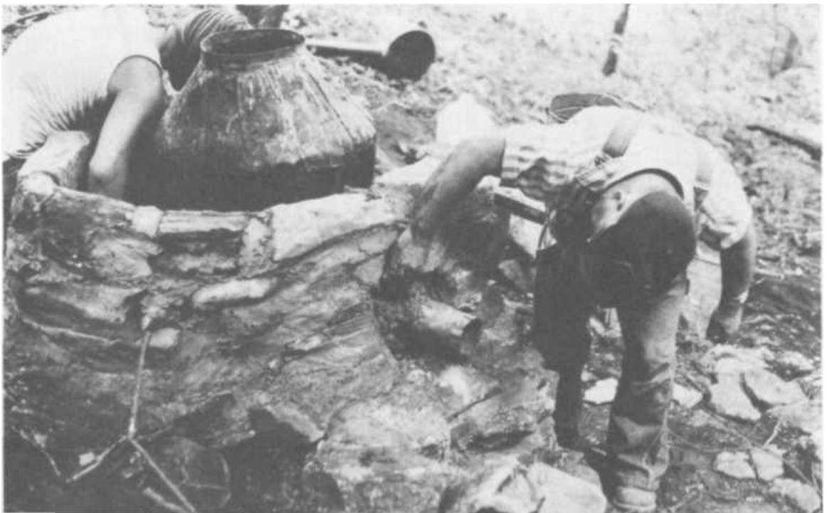
PLATE 437 Then he sealed the hole around the slop arm with red-clay mud while one of the students helped by lining the sloped inside back wall of the furnace with cement and smoothing it up.
