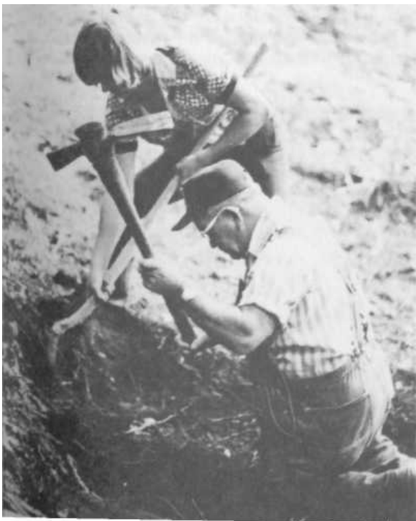
PLATE 426 The first step is to choose a suitable hillside hidden in the woods. Buck always sets his stills into a bank so that he can stand on the ground behind the still and get to it without using a ladder. The site selected, he and Joey Fountain, one of the Foxfire students, dug out the hole for the furnace.
