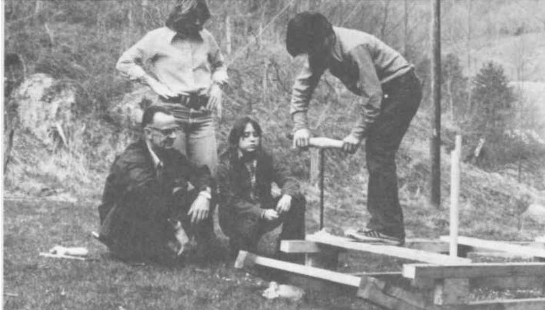
PLATE 172 With the 1" auger, Dwayne drills down through the oak crosspieces, the sills, blocks, and well into the runners. Long dowels driven into each of the six holes hold the sled together and keep such loads as logs from rolling off.
