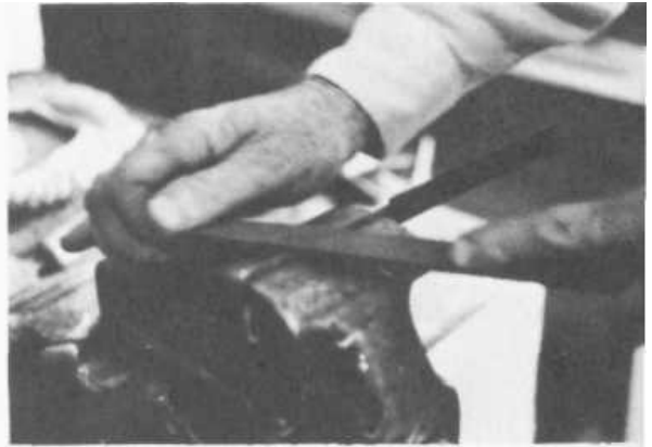
PLATE 15 Then he files the ragged edge smooth.
