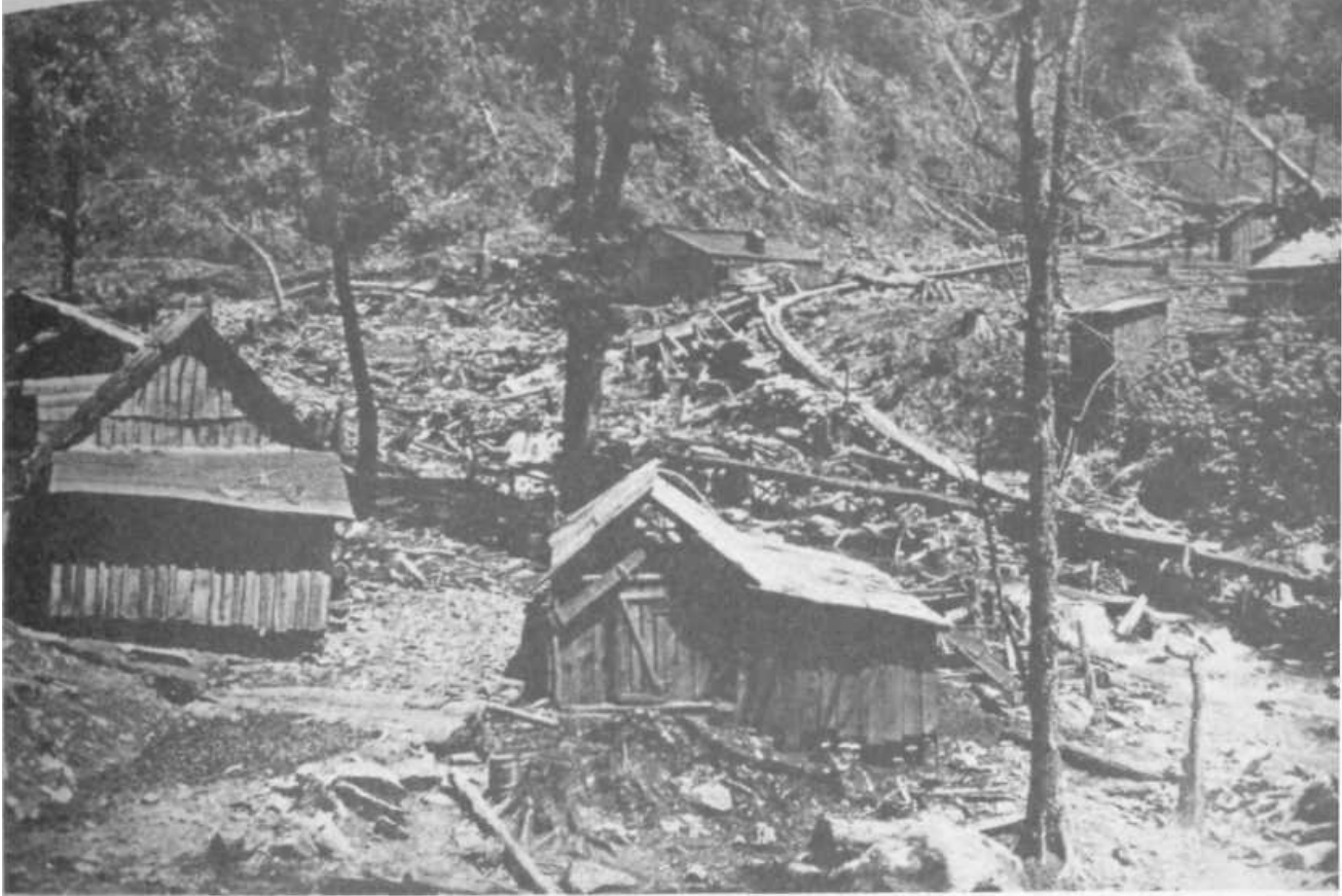
PLATE 286 A logging camp high in a watershed. The buildings would be family homes, stables, a dining hall, outdoor toilets, and so on. The flume through the middle of the camp indicates that this was one of Champion's acid wood operations. (Photo courtesy of Champion Paper.)
