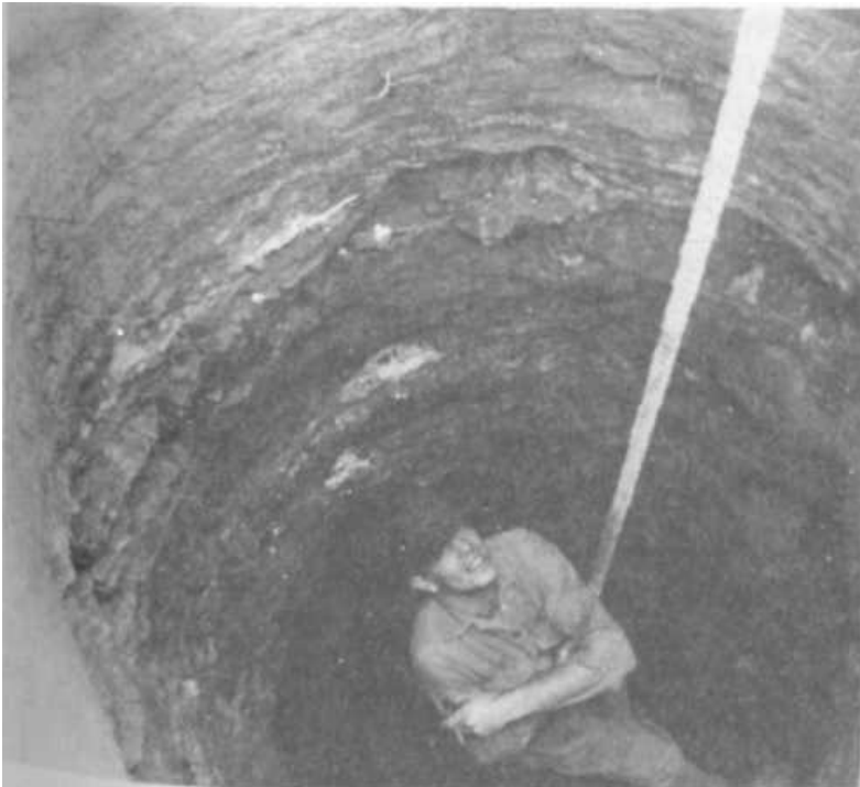
PLATE 353 Harold Embrey being lowered into the well to continue working. The Embrey/Ramey well is 52" at the top and tapers to 42" at the bottom. The first five feet were through dirt. Then they hit white flint rock and had to use a hammer and chisel. After four or five hours, they cut through that and had dirt again until they hit solid rock above the water level. They had to blast with dynamite twenty-five times to get through it. Below that level was water, running at a rate of five gallons a minute.
