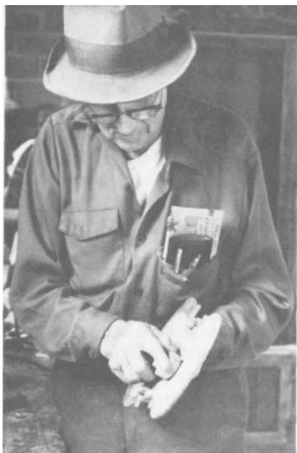
PLATE 113 With the plane, Harley shapes out the top and the back of the fiddle until they are about 1/8" thick.
