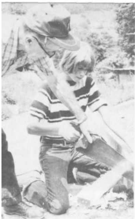
PLATE 175 Then he shows Ken how to cut a series of slots at the spot the pole must bend.
