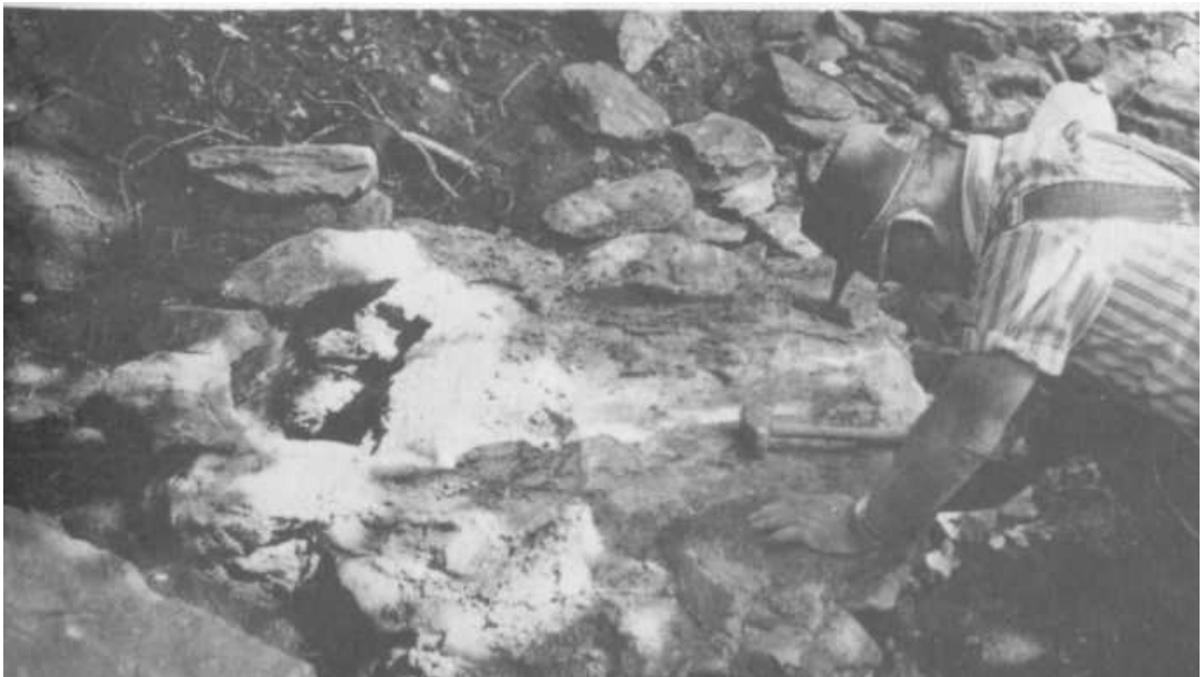
PLATE 430 The hole left at the back of the platform is for the flames, which will come up from the firebox below and wrap around the still, heating the contents to a boil.
