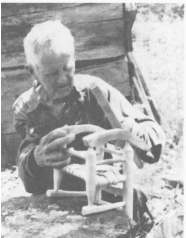
PLATE 75 Two holes are drilled into the top of each rocker, and the rockers are tapped into place.
