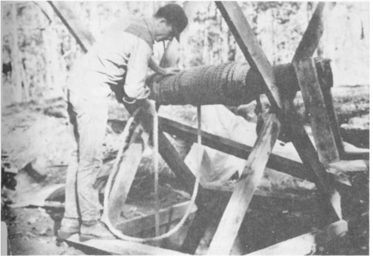
PLATE 352 We visited Harold Embrey and Tom Ramey who were digging a well in our county. They had hit water at forty feet by the time we got there and were finishing up. It took them six days to hit water with seven men digging off and on. Here, the bucket is being lowered into the hole to be loaded with dirt and rock.
