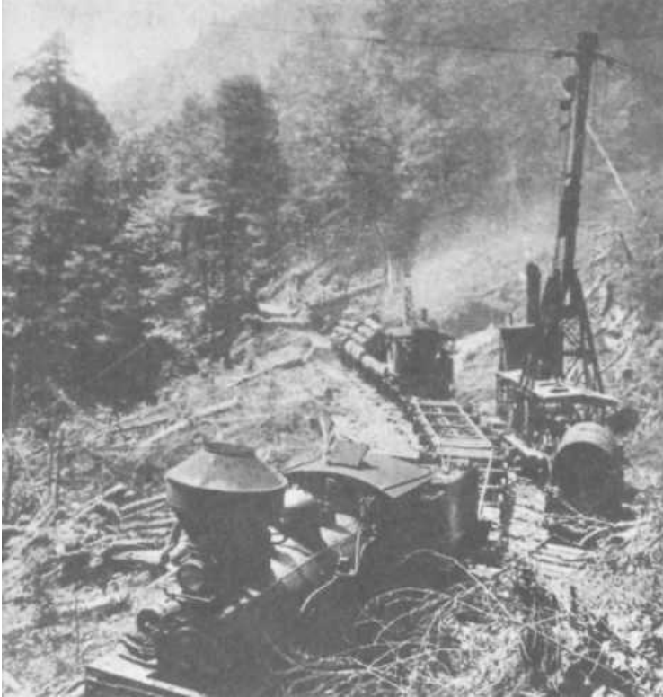
PLATE 277 At the head of the rail, road line, an overhead skidder (far right) powered by a steam boiler would be used to drag the logs out of the woods, where they had been cut, to the loading area. There a log loader (or "stiff-necked loader"), visible in this photograph on the tracks beyond the steam engine, would load the logs onto the railroad cars for the trip to the mill. When one car was filled, the loader would pull off the main track onto a short siding so that the engineer of the train could move another empty car into position to be loaded. (Photo courtesy of Champion Paper.)
