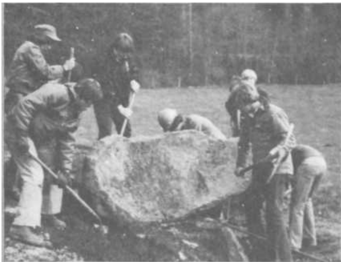
PLATE 251 To turn the rock over we dug the earth out from behind it and rolled it back using poles as levers.
