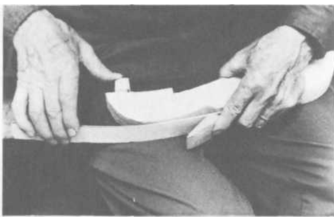
PLATES 133-134 The sides are clamped into forms as shown.
