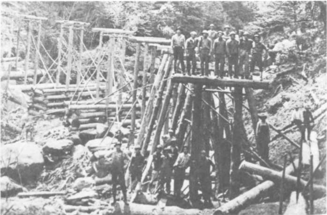
PLATE 274 Narrow-gauge railroads were also used for hauling large logs, surh as balsam, to the mill. Often trestles were required, and a man like Rube Mull and his crew would be railed in to build them. This trestle probably went up into Little East Fork, an area that is now the Pisgah National Forest. (Photo courtesy of Champion Paper.)
