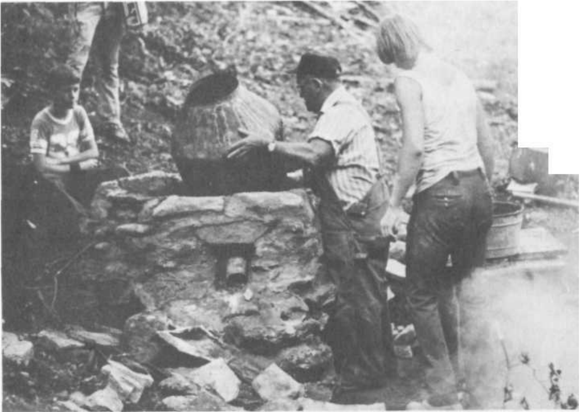
PLATE 436 When the rock sides were high enough to reach the cape of the still, Buck set it back into place.
