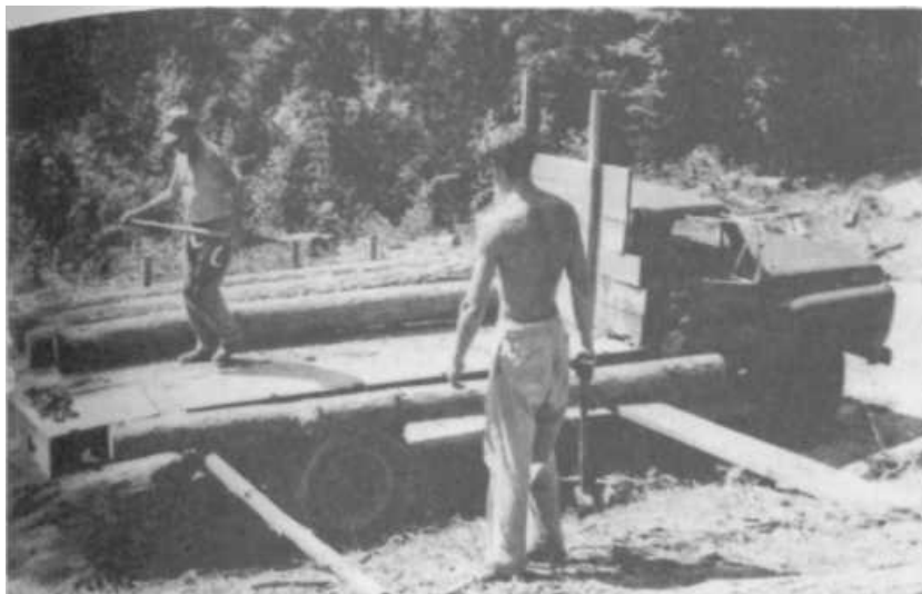
PLATE 268 At the truck, the logs are loaded by rolling them over skid poles onto the bed. They were often loaded onto wagons, years before, in the same manner.
