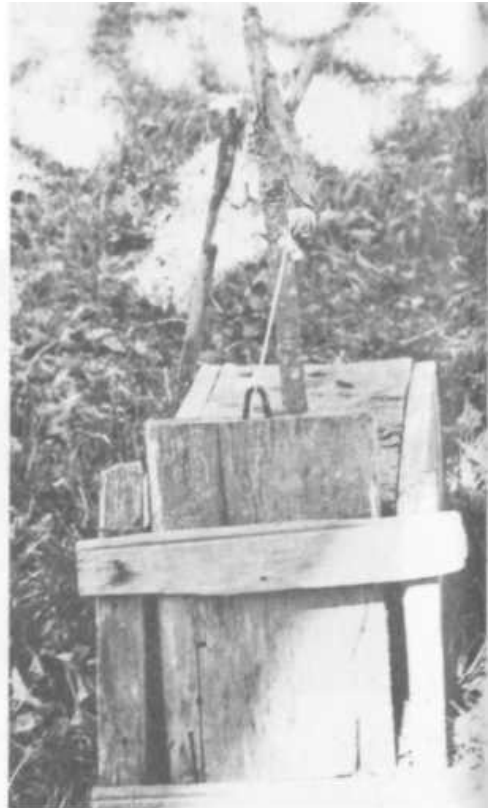
PLATE 232 The bait is placed behind the notched triggering stick. When the rabbit pushes against this, it is released . . .
