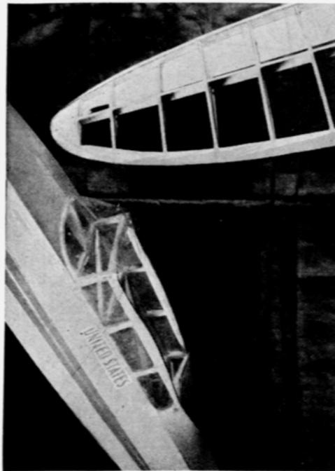
Here you see how the wing is constructed and details of the cabin construction
