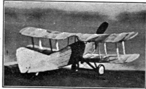
A small door is cut in the rear of the fuselage to allow rubber to be inserted. The rear hook is formed of .034 piano wire and attached in the body with several coats of cement.
