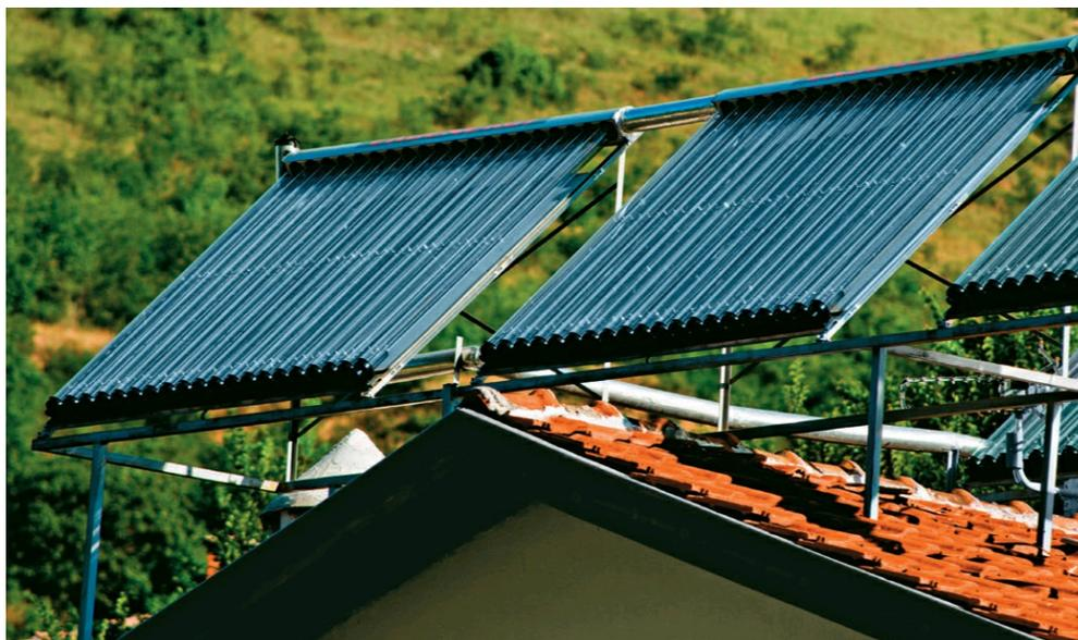
**The mounting system** used for this solar hot water collector straddles the ridge of the roof so that the panels will face due south even though the house faces east/west.
