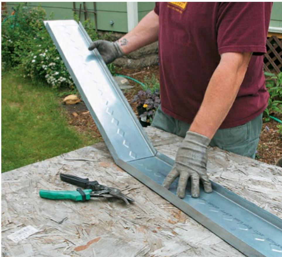
**1** Cut and bend the box frame pieces from  $2 \times 6$  steel studs. Each steel stud piece will wrap two sides of the panel with a  $90^\circ$  corner bend. Mark the bend location on both steel studs. Cut a relief into the 6" side of the stud with aviation snips at this mark. Bend the stud to an L-shape and use a square to ensure that the corner forms a true  $90^\circ$  angle.
