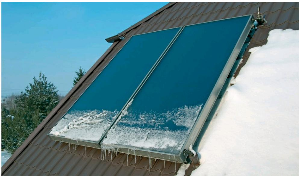
**Drainback solar hot water systems** are safe for year-round use, even in cold climates. Water is pumped to the collectors only when the temperature in the collector is higher than the temperature in the storage tank, so there's no danger of freezing pipes.
