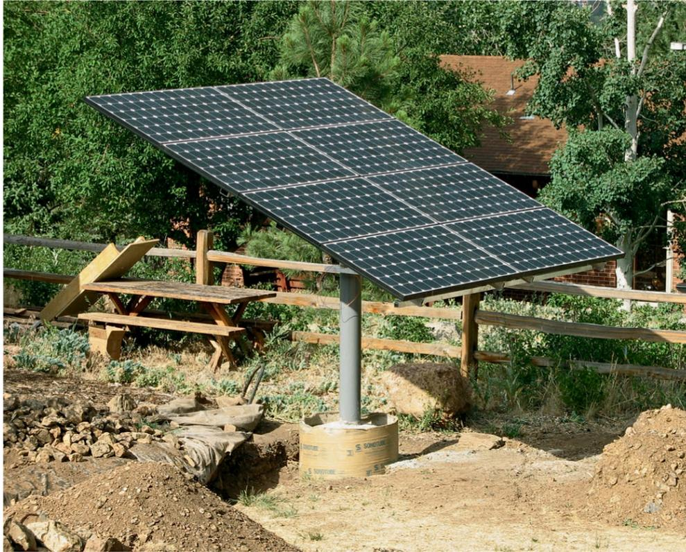
**Mounting solar arrays on the ground** offers greater flexibility in placement when rooftop installation is impractical, or is prohibited by local building codes or homeowners associations.
