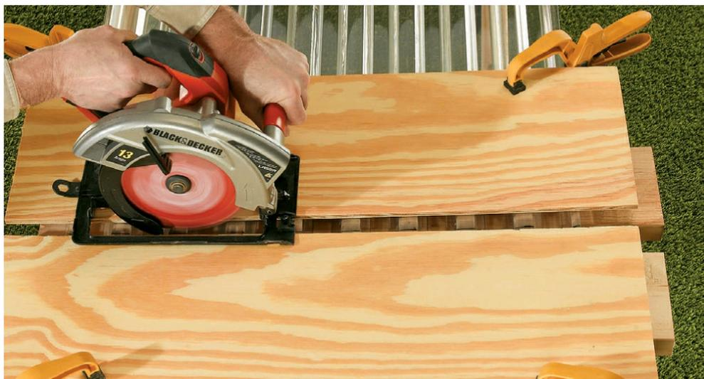
**20** Align the four polycarbonate panels, then clamp the ends with spring clamps and mark the cut line. Place 2 × 4s under both sides of the cut, then place cardboard or plywood on top, under the circular saw, so the panel doesn't get scratched. Use a sharp plywood-cutting blade (or whatever blade the panel instructions recommend) to cut the panels.
