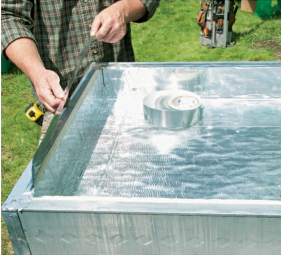
**6 Seal the insulation edges.** Place a bead of silicone around the inside corner where the insulation strips and backing panel meet, and then seal with foil tape. Flip the panel over. Place a bead of silicone on the intersection of the 2 × 6 stud flange and the back of the insulation, and seal with foil tape. Conceal any exposed insulation edges with foil tape.
