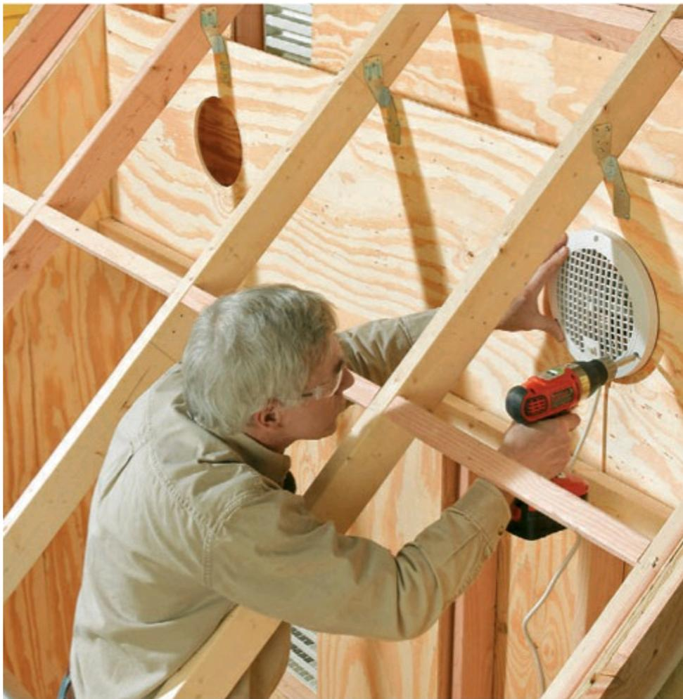
**17 Fasten the fans** to the shroud. The fans are turned on during the day to circulate the air, then turned off at night so the wood doesn't dry too quickly, so they should be plugged into a timer.
