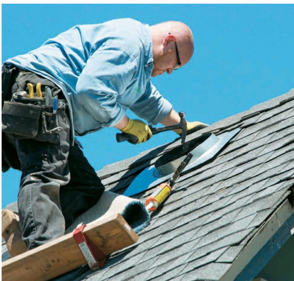
**15** Use a **roof jack** or Cone-jack to form an 8"-dia. opening. Apply a heavy double bead of roofing cement along the top and sides of the roof jack. Nail the perimeter of the flange using rubber gasket nails. Cut and install shingles with roofing cement to fit over the flashing so they lie flat against the flange.
