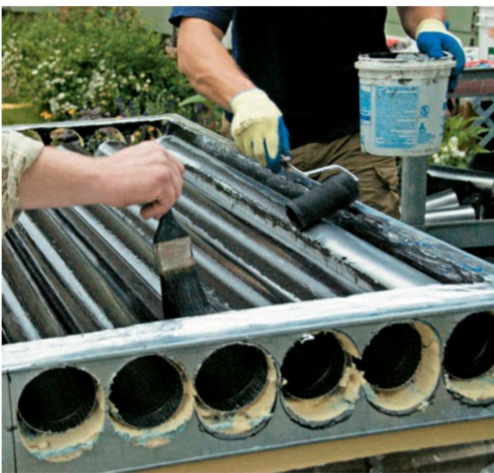
**11** Paint the last section of ductwork and touch up around the interior of the box so all exposed surfaces are black.
