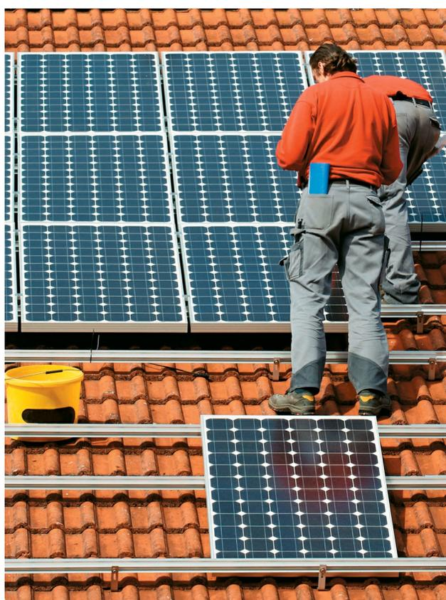
**The large surface** area of solar panels means that they must be very securely mounted to resist the force of the wind.
