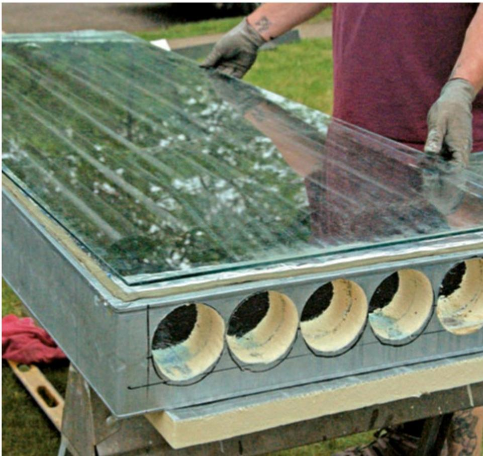
**12** Affix the glass top. First, double-check that all openings in the panel are adequately sealed and insulated. Then, line the tops of the steel stud frame with foam closed-cell gasket tape. Carefully position the glass on top of the gasket tape, lined up 1/2" from the outside of
