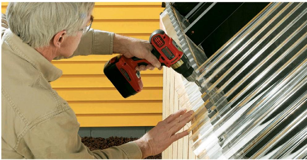
**21** Set the panels in position over the foam closure strips, then predrill the holes on the crowns. Use a sharp bit 1/8" bigger than the diameter of the neoprene screw to allow for movement. Don't overtighten the screws—they should be tight against the panel, but should not distort it.
