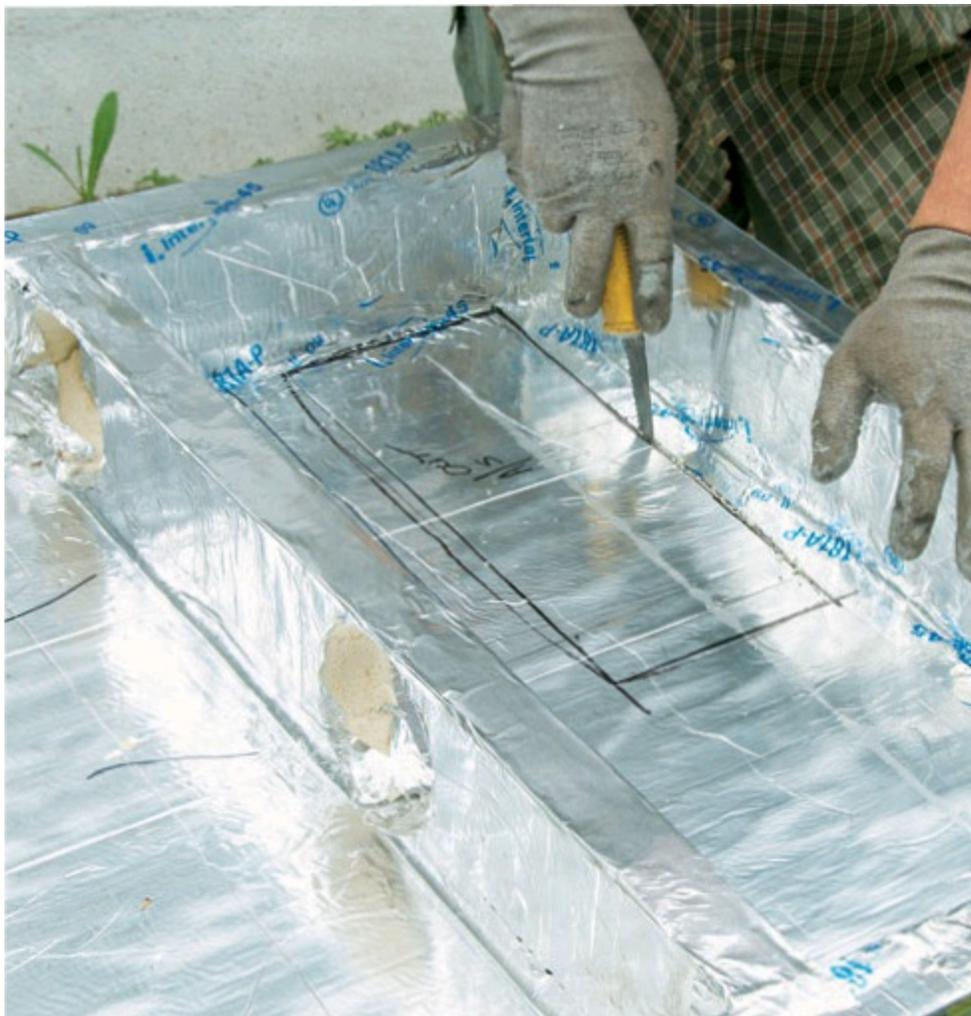
**8** Install a **compartment separator** in the first and last panels with a piece of foil insulation set on edge. Cut ductwork access holes in the separator. Then, cut out holes for the ductwork that will pass through the separator. Also cut a plenum opening in the separated compartment in the first and last unit.
