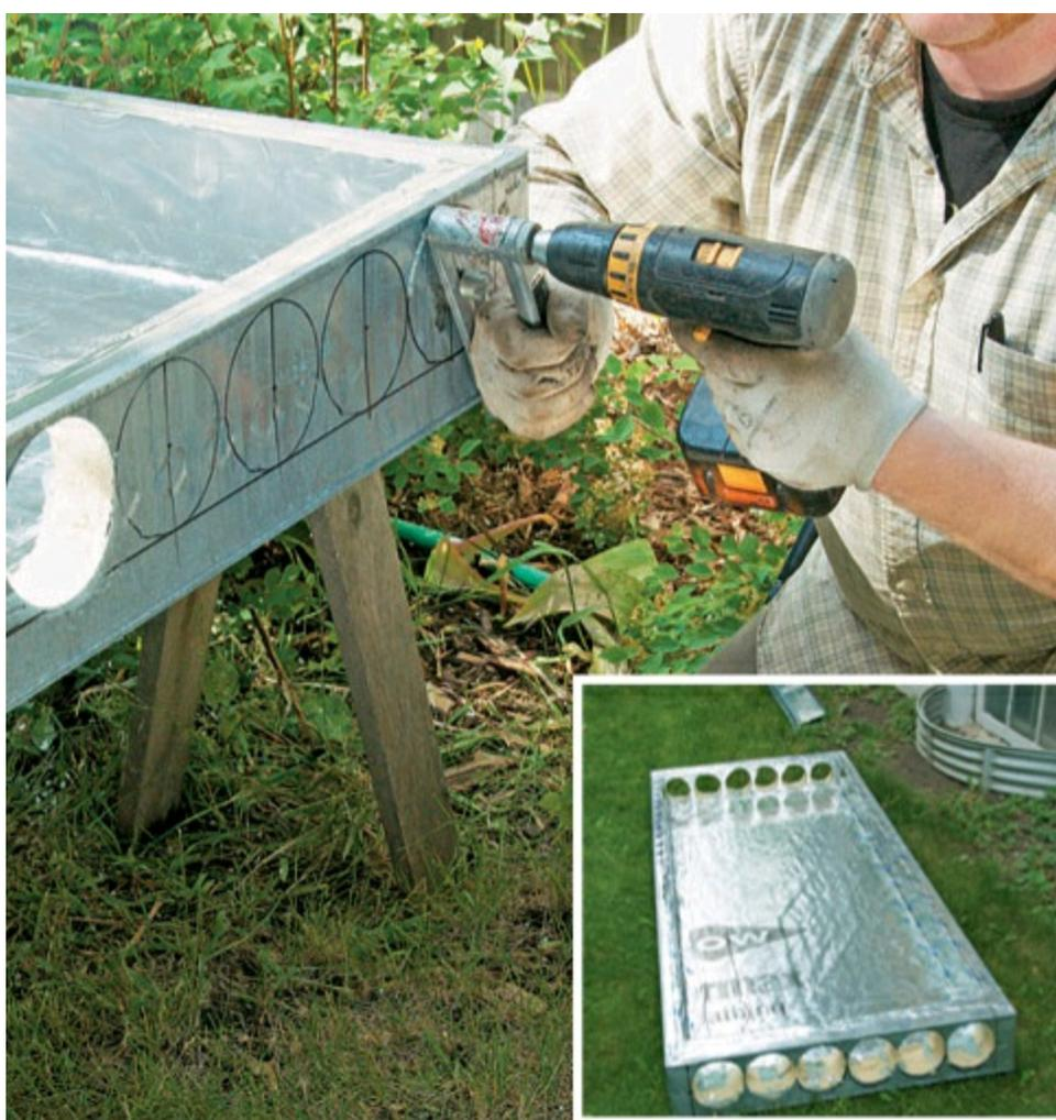
**7** Create **inlet and outlet holes** in the walls with a hole saw or circle cutter. The number and location of the ductwork holes depends on where each panel fits into the overall array (presuming you are making and installing multiple panels). The first and last panels in the series will each have one end wall that is uncut, while intermediate panels will have duct holes on each end wall (inset).
