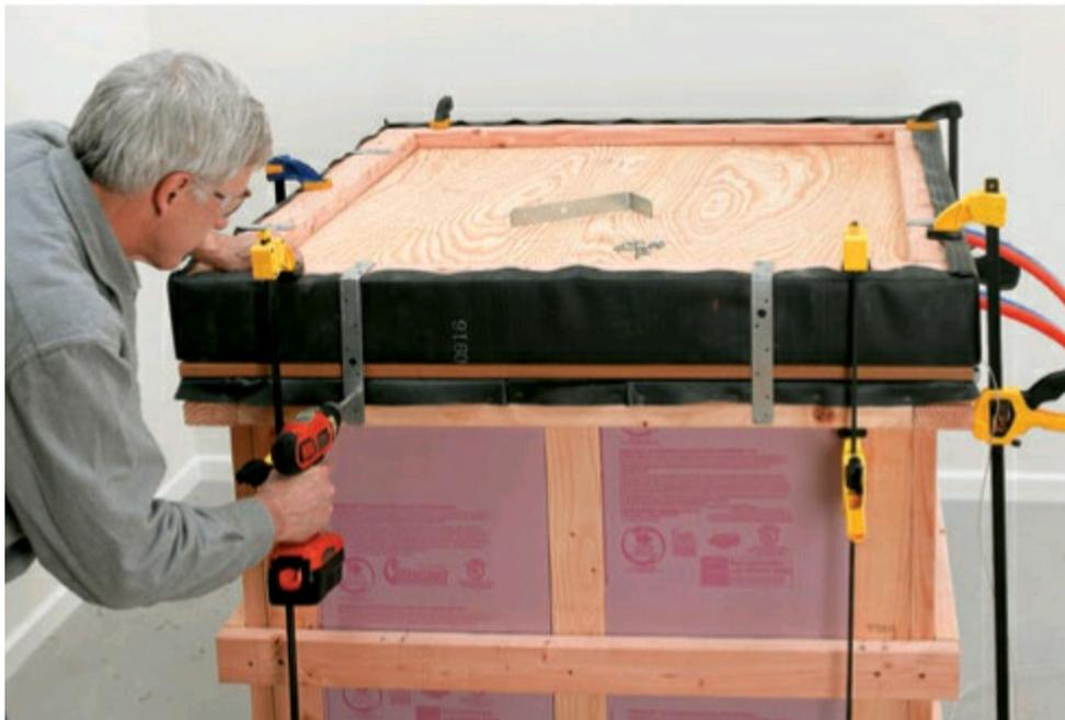
**17** Complete the plumbing connections inside the tank, fill gaps around the pipes on the ledge with silicone, then clamp the top down tightly to seal the edges. Fasten the top to the base with galvanized strap and deck screws.
