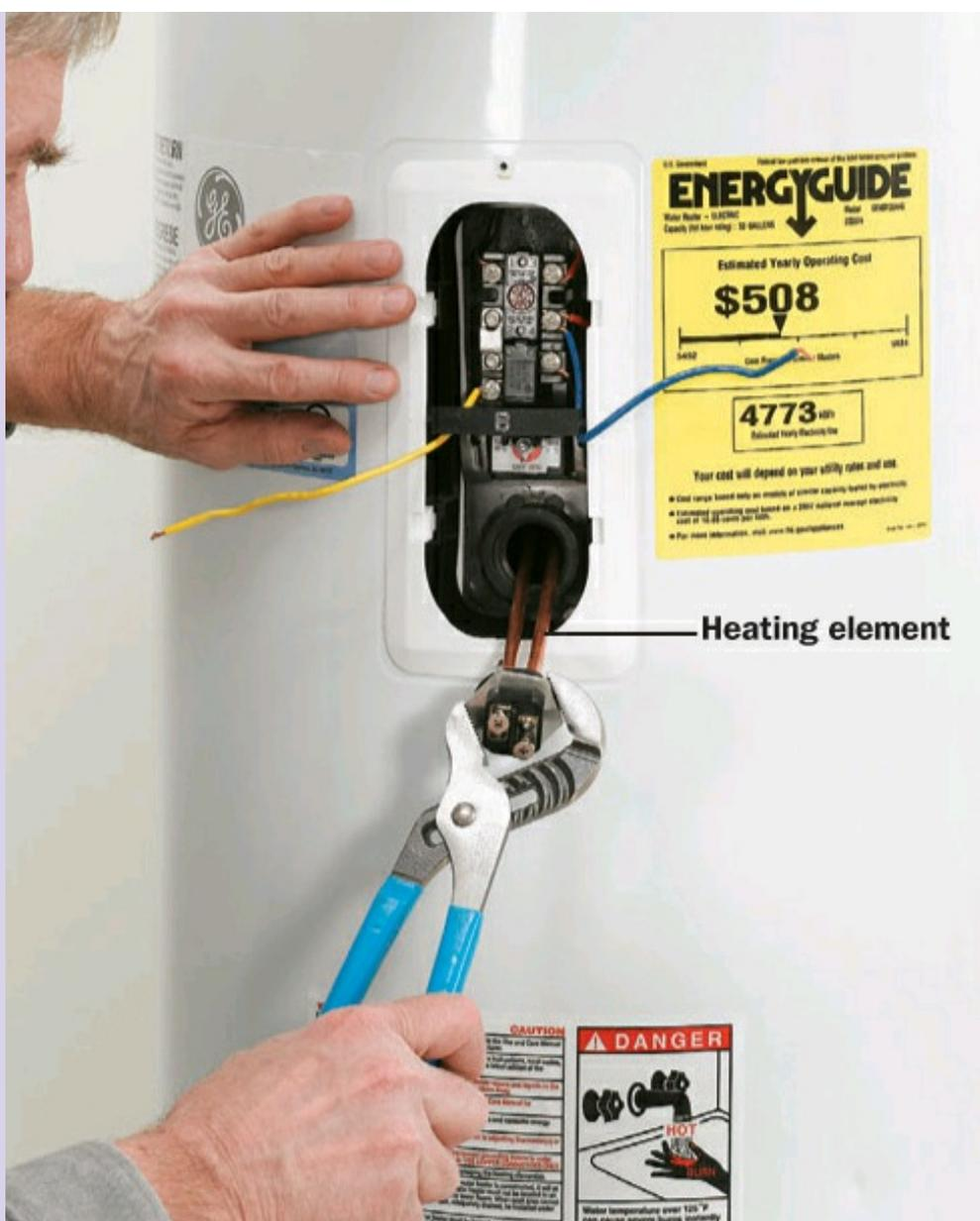
**Turn off and disconnect** any wiring to the heater you'll be converting to a storage tank. Remove the covers over the heating elements, cut away the wiring, then turn out both heating elements with a socket wrench or a channel lock wrench.
