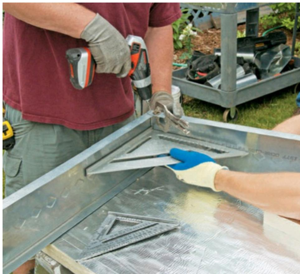
**2** Drill 1/8"-dia. holes in the overlapping top and bottom flanges. Clamp the corners together before drilling, using a square to make sure the corner forms a 90° angle.
