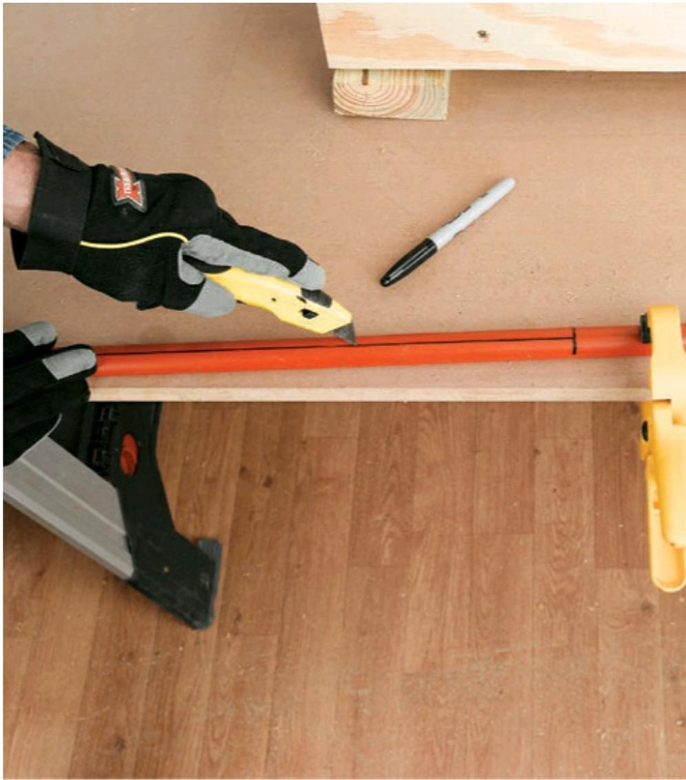
**9** Mark the first 19" of PEX , then cut it in half with a utility knife. Score it lightly at first to establish the cut lines.
