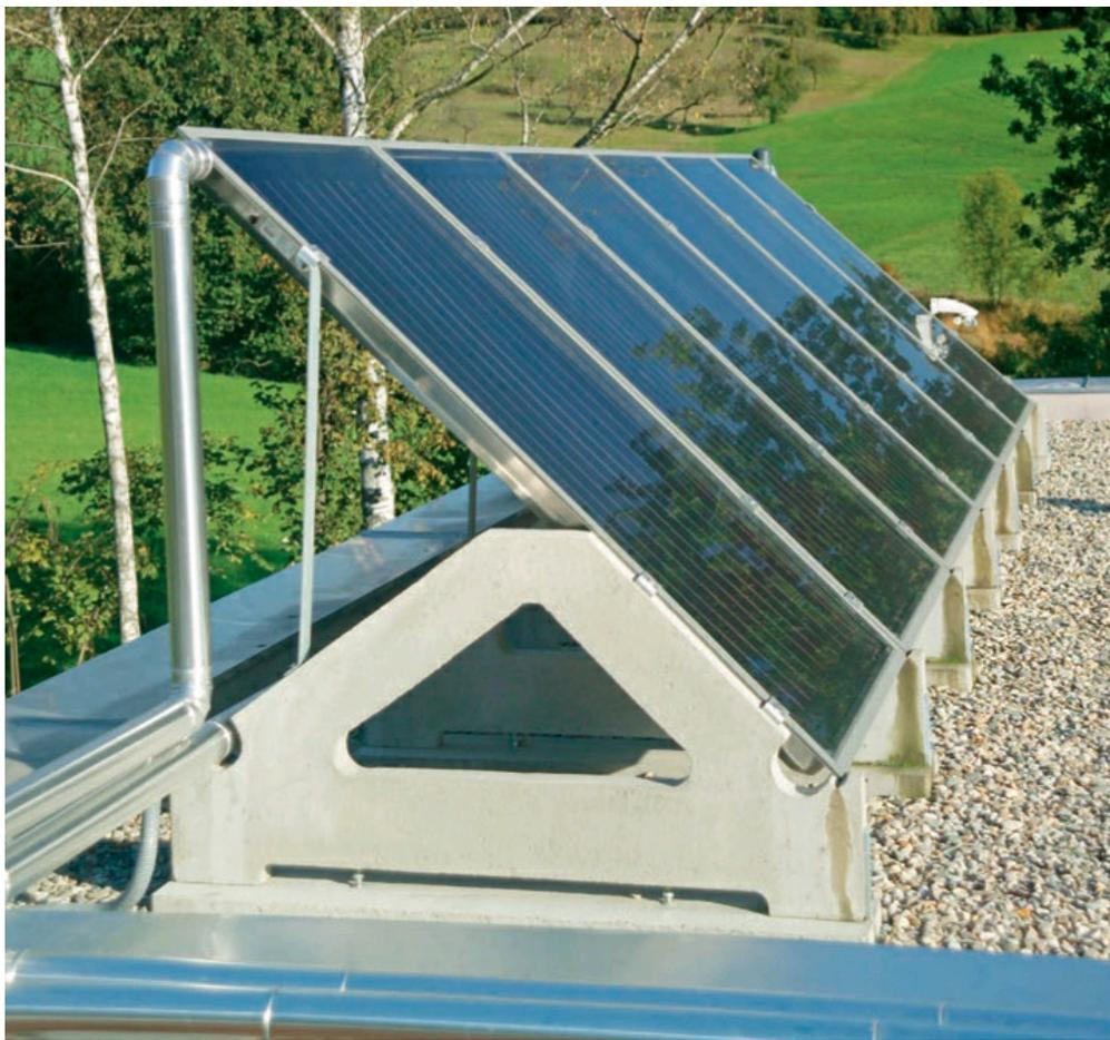
**These molded supports** for solar hot water panels are set at 45°-a safe, compromise angle for year-round use in most of the country. The wide base of the supports distributes the weight of the panels evenly on the flat roof.
