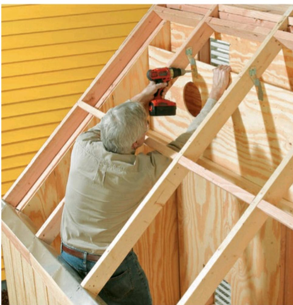
**16** Cut the shroud that the fans are attached to from 3/8" or 1/2" plywood. Attach 2 × 4 nailers to the sides (hidden behind the shroud in this photo), and screw a 2 × 4 across the bottom. Make cutouts for the fans you buy, then hang the shroud from the rafters with hurricane ties and screw the 2 × 4 to the side walls. (Fans can be any inexpensive type, 8" to 14" round or square, as long as you can find a way to fasten them.)
