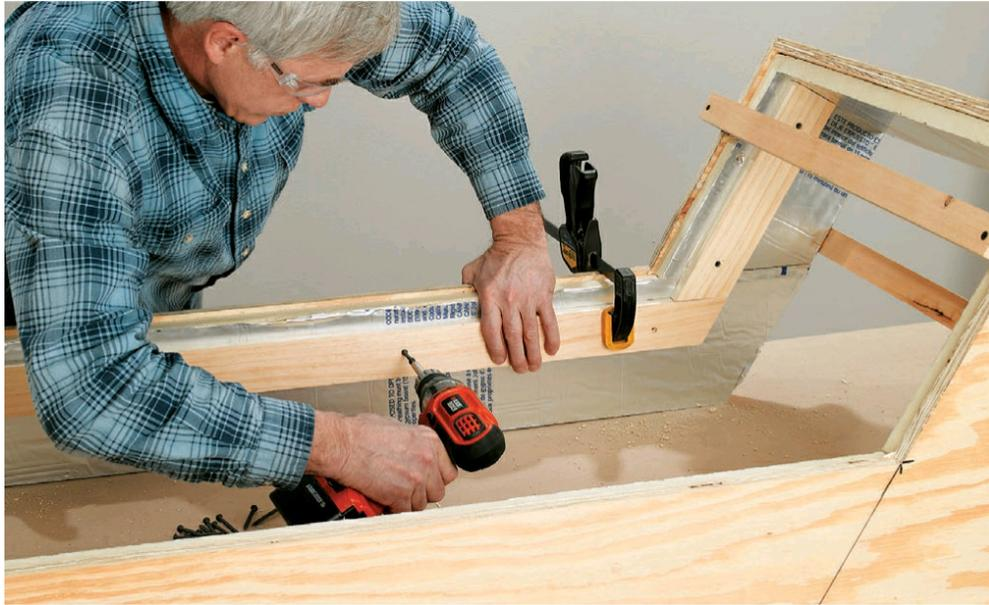
**5** Screw the 1 × 3 nailers to the sides of both the long and short pieces using 2-1/4" screws. Place the nailers 1-1/4" from the bottom edge to leave room for 1" insulation and 1/4" plywood.
