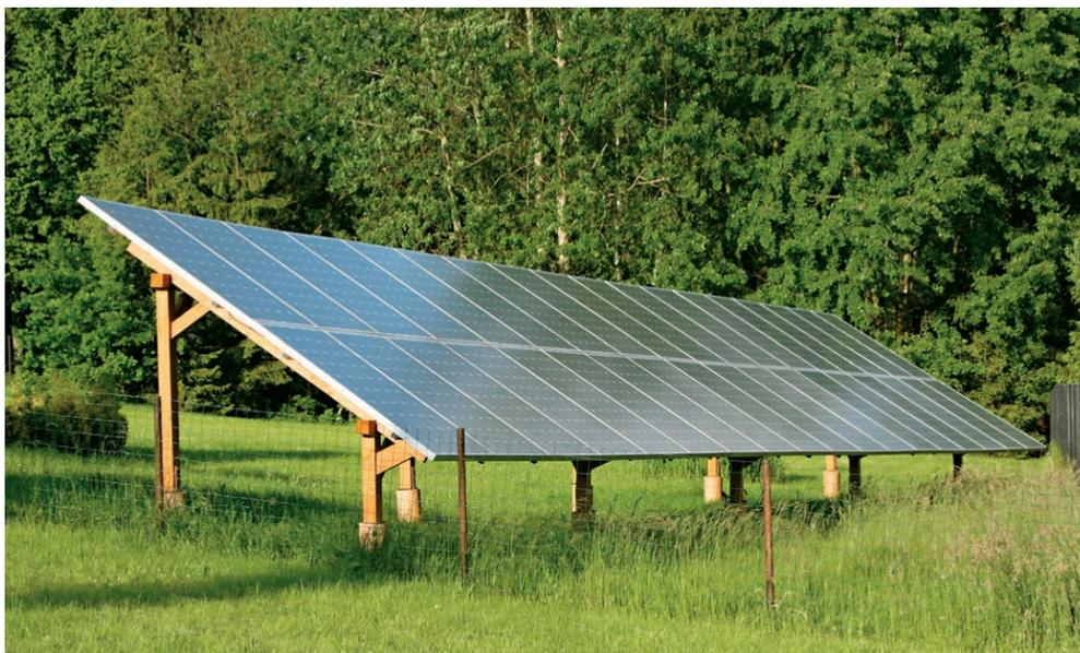
**To protect them** against damage due to frost heave and ground movement, solar arrays must be set on posts that go down to frost-footing depth, or at least 2 ft. When using treated lumber, let it dry out for several weeks before using it so it doesn't warp or shrink under the panel.
