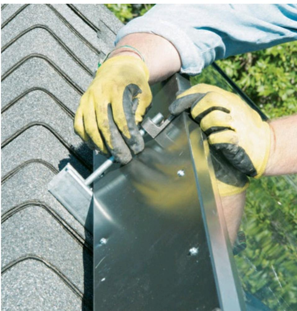
**19** Connect the panels to the Unistrut with 3/8" threaded rod attached at the top and bottom of the panel on the outside. Cut threaded rod to size, then attach to the Unistrut with Unistrut nuts. Attach the top clip to the top of the rod and the front face of the panel. Tighten the assembly to compress the panel down to the Unistrut for a tight hold.
