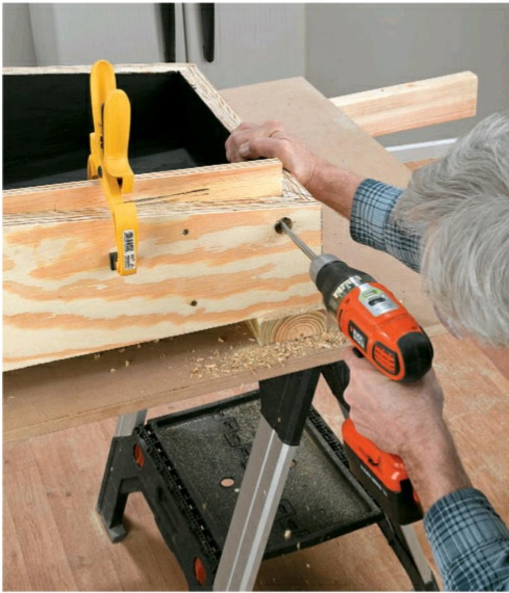
**8 Drill a hole** for the PEX drain. The top of the PEX is 1/2" down from the top edge. Clamp a scrap piece to the inside so the drill bit doesn't splinter the wood when it goes through.
