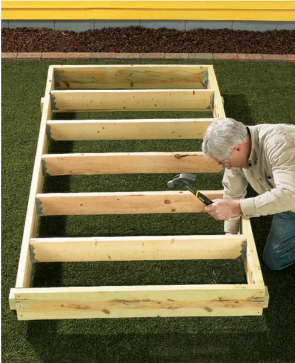
**1** Level a base of treated wood or concrete blocks at the kiln location, then build the frame for the floor on top of them. The kiln should be built in a south-facing location that gets at least 5 to 6 hours of direct sunlight.
