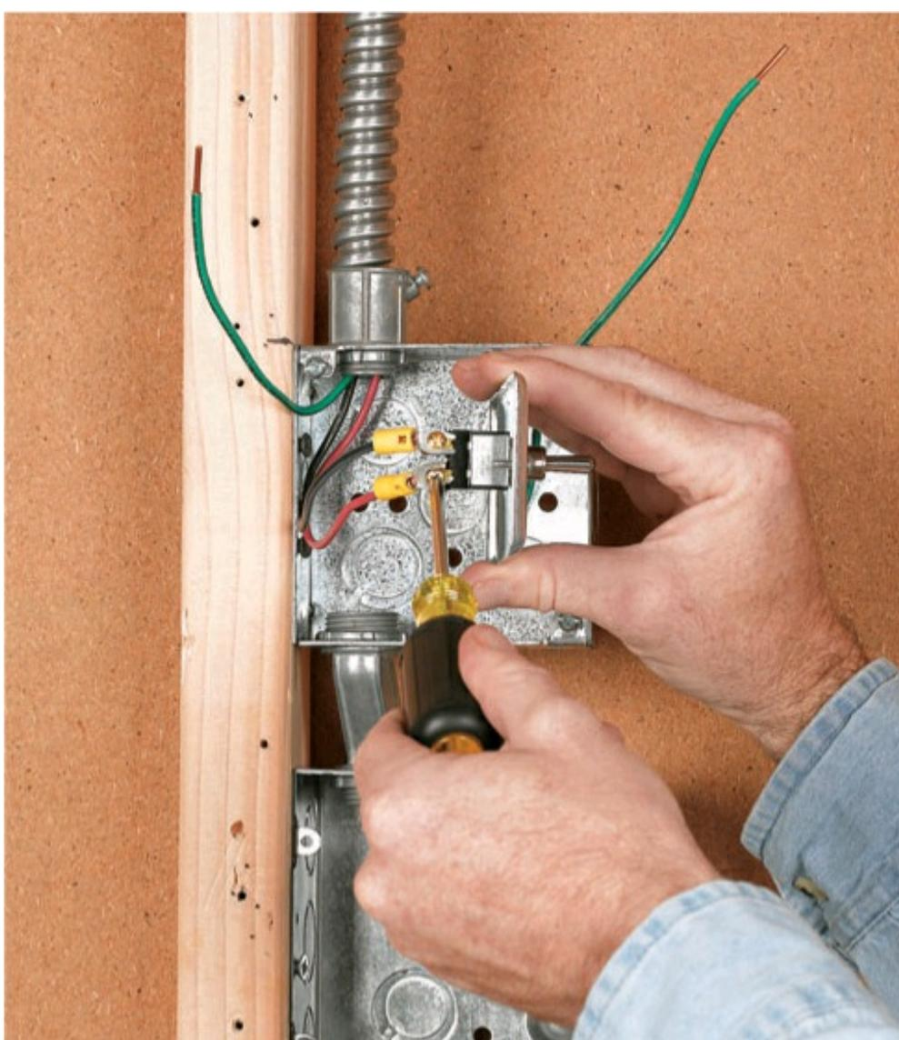
**6** Attach the DC disconnect switch to the wire leads from the power source.
