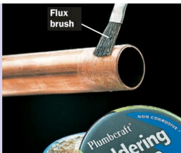
**Apply a thin layer** of soldering paste (flux) to end of each pipe, using a flux brush. Soldering paste should cover about 1" of pipe end.
