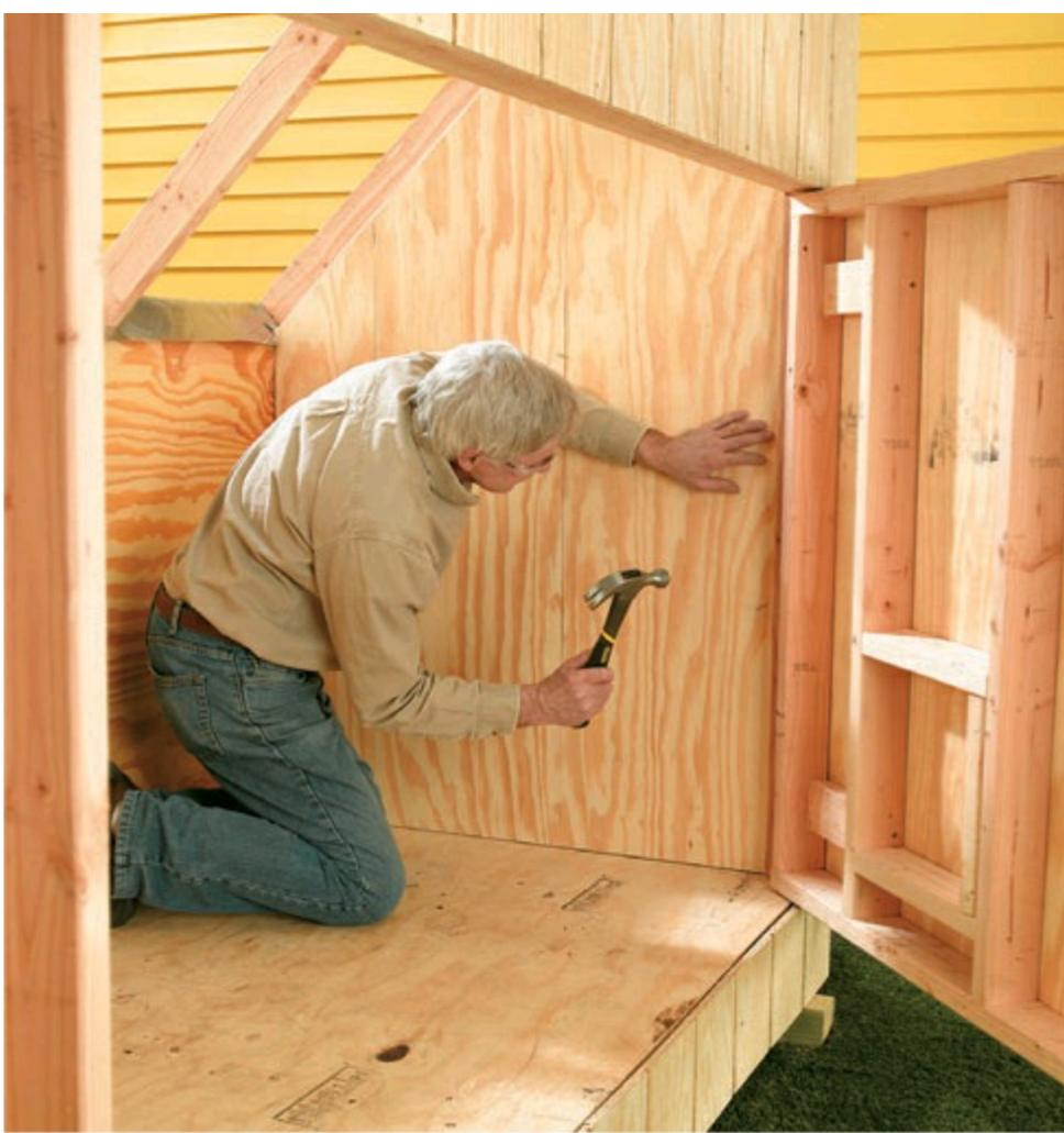
**14** Add insulation to the walls and doors, staple on the vapor barrier, then nail on the interior plywood siding.
