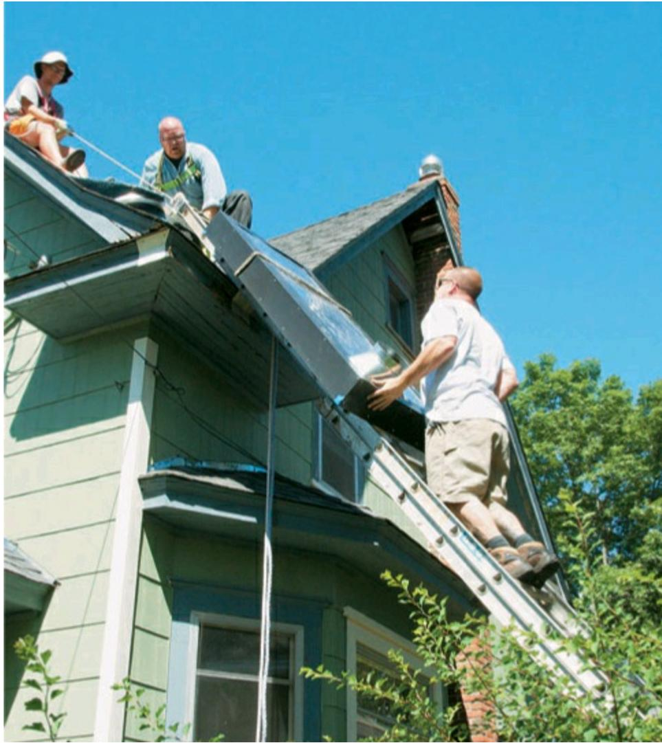
**17** Hoist the panels into position. Carefully follow safety regulations and use scaffolding, ladders, ropes, and lots of helpers to hoist the panels onto the roof. Wear fall-arresting gear and take care not to allow the plenum ductwork to be damaged.
