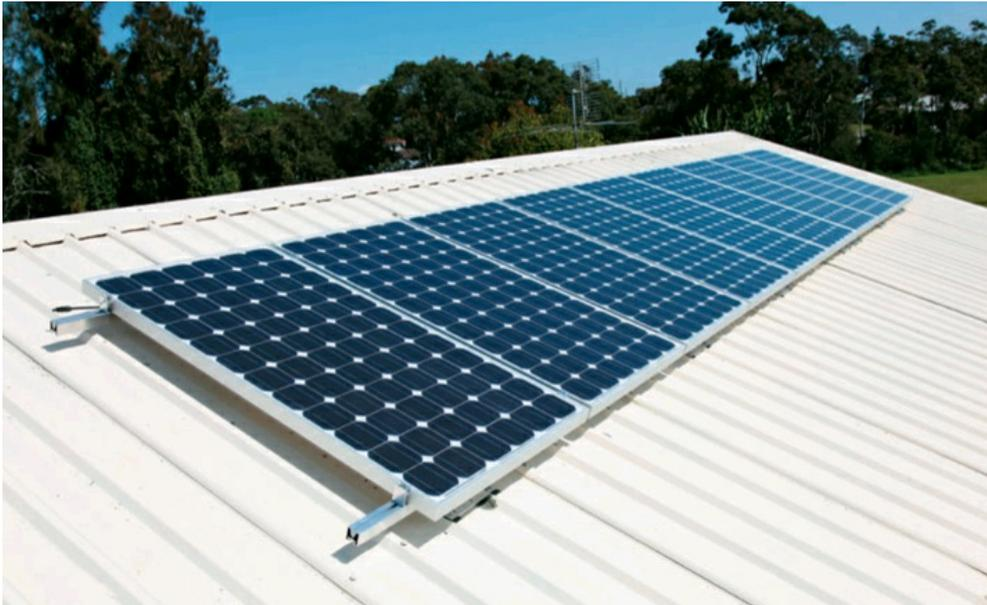
**Two elements of an energy-efficient house:** The photovoltaic panels provide most of the electricity, while the white roof reflects the sunlight and keeps the house cooler, substantially reducing energy demand.
