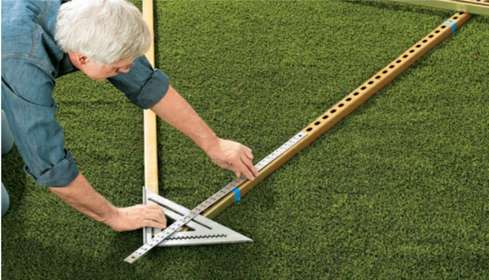
**1** The easiest way to figure out the strut lengths is to lay the three pieces on the ground, move the support piece to the proper angle using the angle markings on the speed square as a guide, then mark the cuts. Use tape to mark the location of the solar collector or panels and the points where the adjustable support leg will be attached.
