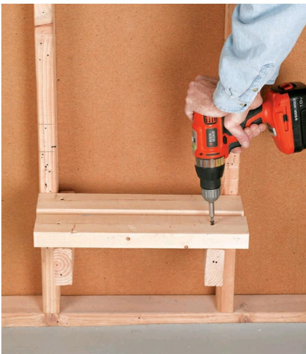
**9** Build a support shelf for the battery using  $2 \times 4$ s. The shelf should be at least 18" above ground. Set the battery on the shelf in a sturdy plastic case.
