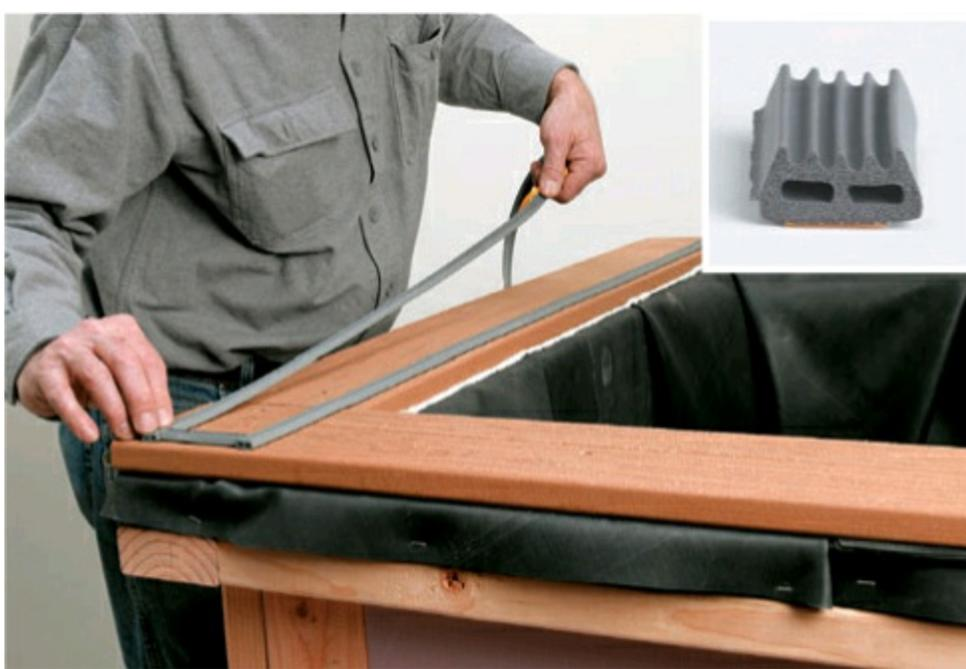
**16** Add two strips of weatherseal on the ledge about 2" apart. Use a soft foam type that compresses easily and fills voids, like this.
