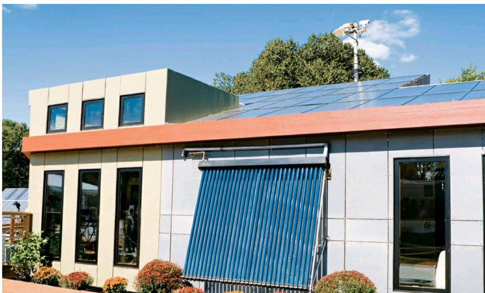
**Hot water collectors** are often mounted almost vertically to capture more of the winter sun and less of the summer. Collectors can actually get too hot if the water sits for a long period. The PV panels on the roof, however, need all the sun they can get.
