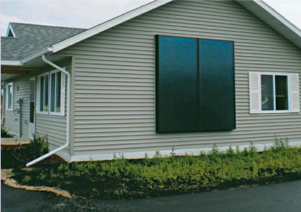
A **solar air heater** was built into the framing of the wall, with the siding trimmed around it (see Resources, p.152).
