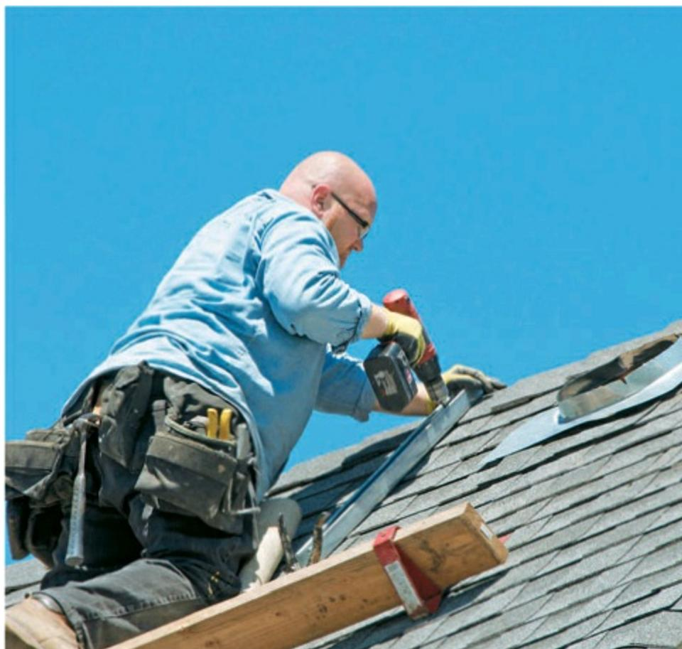
**16** Attach Unistrut mounting U-channel bars to the roof for each panel. Use the chalklines on the roof to determine the position of the Unistrut, and attach to the roof trusses with Unistrut connectors.
