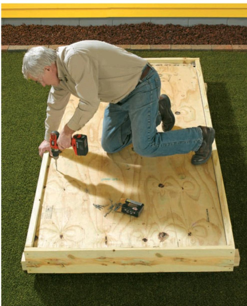
**2 Flip the framework over**, then screw 1/2" treated plywood to the underside of the frame. Caulk all the edges to prevent ants and other insects from colonizing the base.
