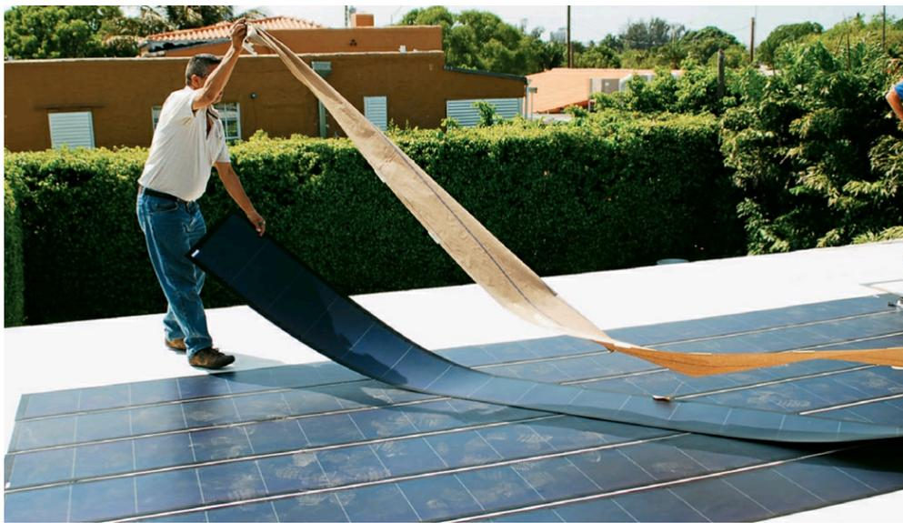
**Mounting thin-film solar** panels can sometimes be as simple as gluing them to a metal roof. Thin-film solar panels aren't as efficient as standard solar panels in full light, but they perform better in low-light conditions. They're also flexible, cheaper to manufacture and more versatile.
