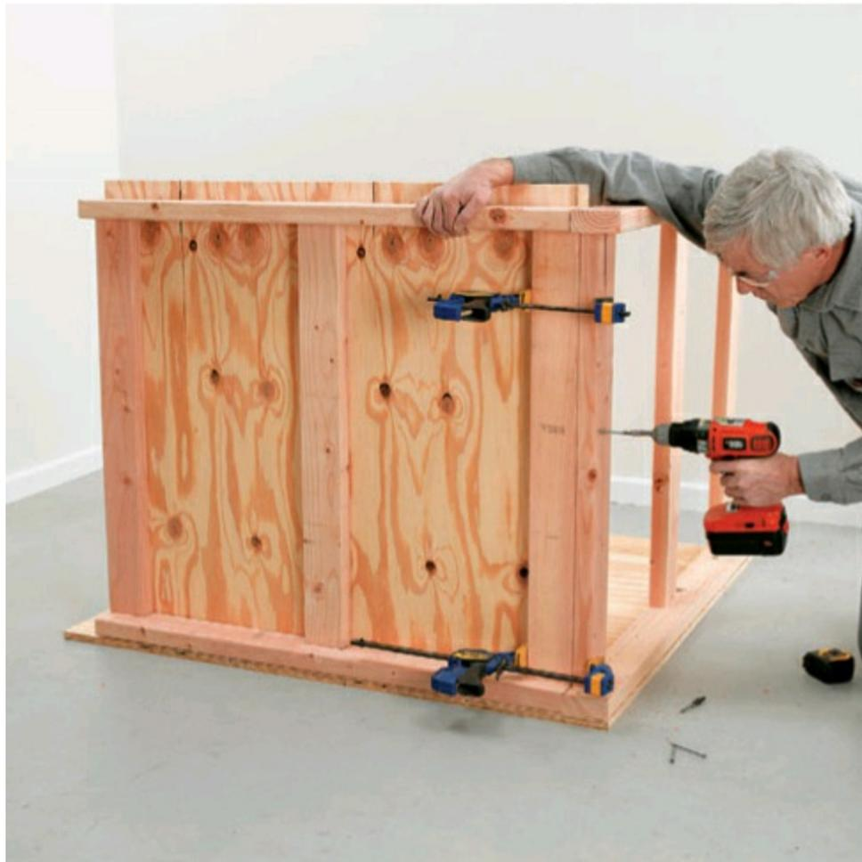
**3** Place the 3/4" plywood base at the tank location, then assemble the short sides to the long sides, fastening the overlapping corner 2 × 4s together with the long deck screws.
