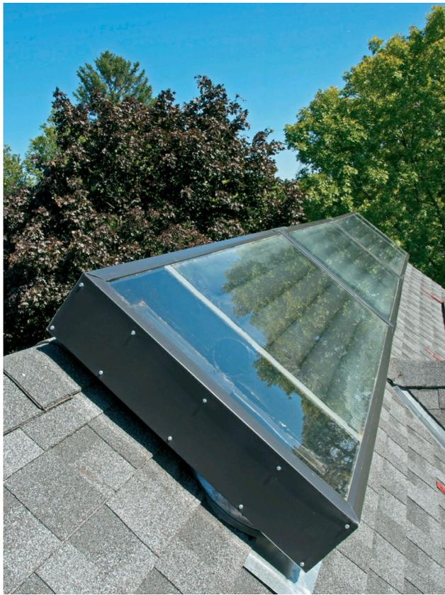
**When combined**, these three DIY “hotboxes” introduce enough hot air into this home to carry 30 to 40% of the home heating load.
