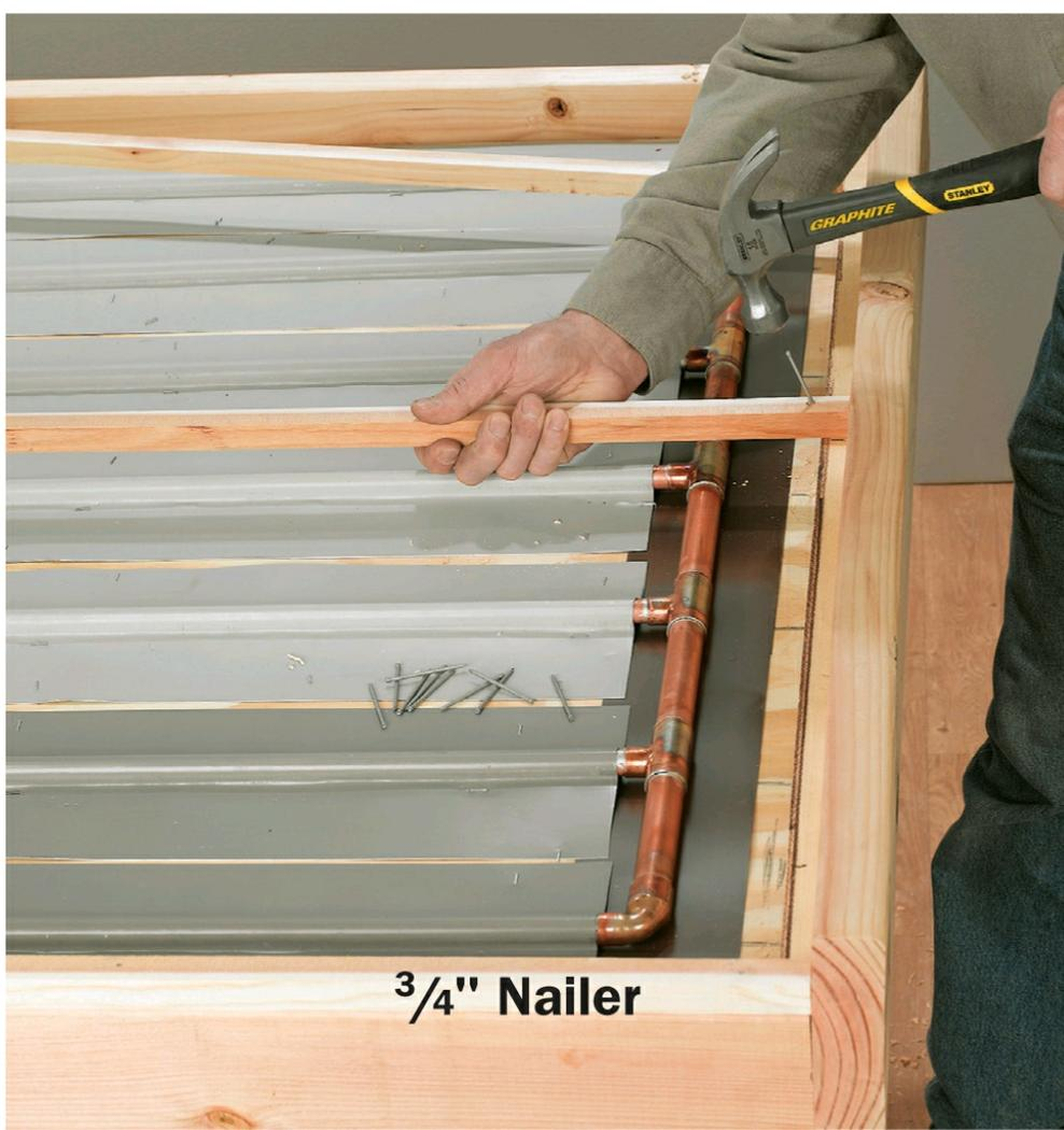
**13** Lay the glazing on top of the box and mark the spots for 3/4" nailers at the sides and the center overlap. Fasten the strips with 6d galv. casing nails.
