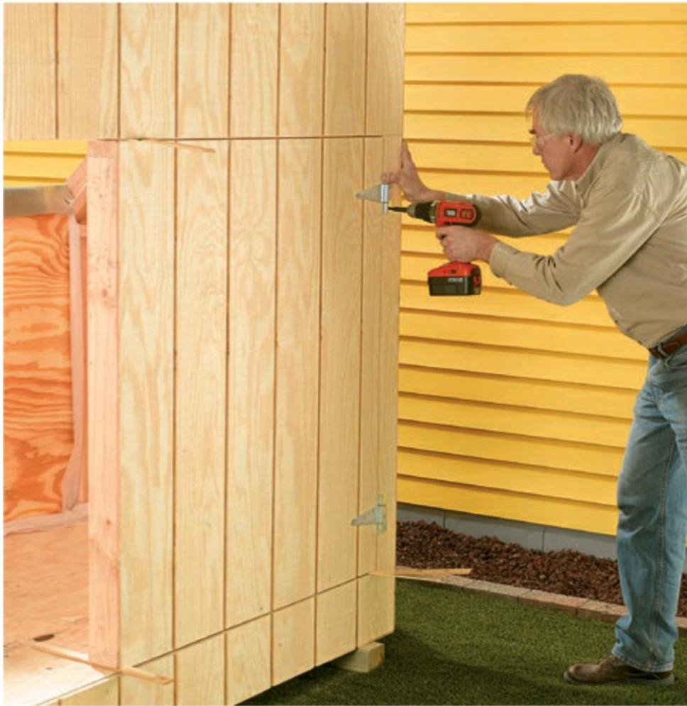
**13** Screw the strap hinges to the doors at the 2 × 4 backer locations. Shim the doors so they're tight and evenly spaced in the opening, with the door against the frame, then screw the hinges to the frame. Drive just one screw into each hinge at first, then remove the shims and check the fit. Adjust if necessary when you drive the rest of the screws in.
