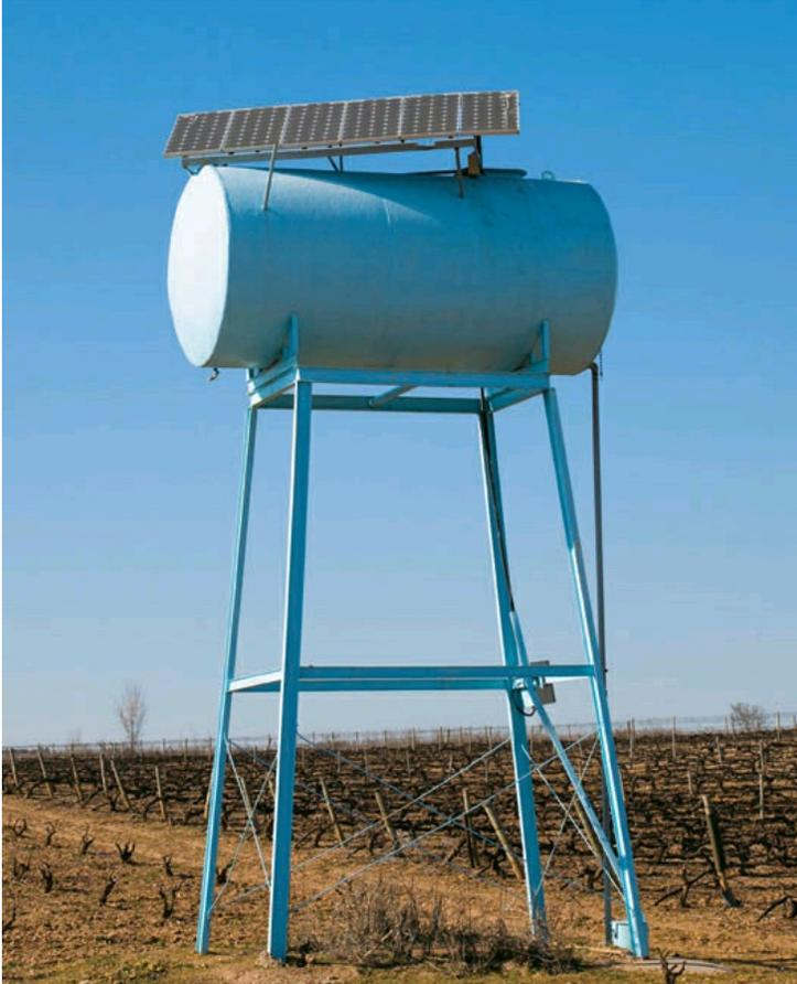
**Water for irrigation** is continuously pumped from a deep aquifer up to this storage tank during the day as long as the sun is shining.
