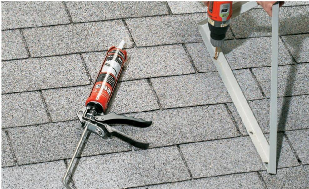
**1 Locate the roof rafters**, either by using a stud finder or by lifting up shingle tabs and tapping in finish nails. You must plan to fasten at least one of the angled mounting brackets to a rafter. If the other doesn't fall on a rafter, plan to attach it with toggle bolt anchors.
