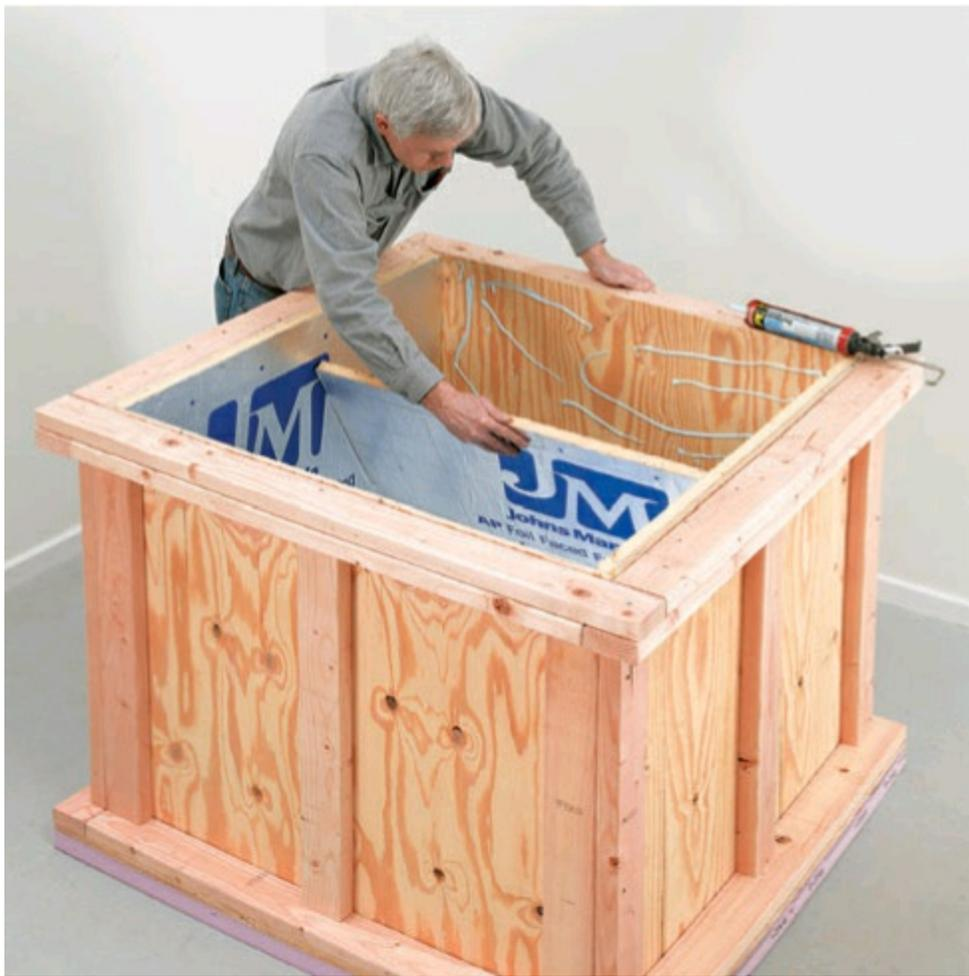
**7 Place the insulation** inside the box, using the foamboard adhesive to attach it. You don't need much; the water will hold the insulation in place. Add the second layer, then seal all the corners on the bottom and sides with silicone caulk.
