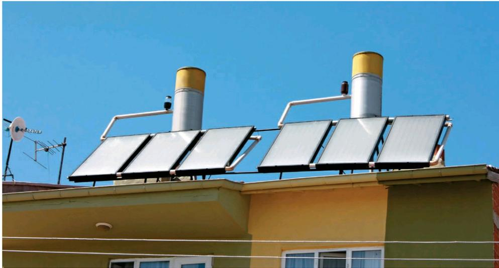
**Thermosyphon hot water heaters** work without pumps or controls. Heated water flows into the upper part of the storage tank, which draws cooler water from the bottom of the storage tank into the bottom inlet of the storage collector. The water is part of the house system, so whenever the hot water faucet is turned on, hot water flows out of the storage tank and fresh cold water flows in.
