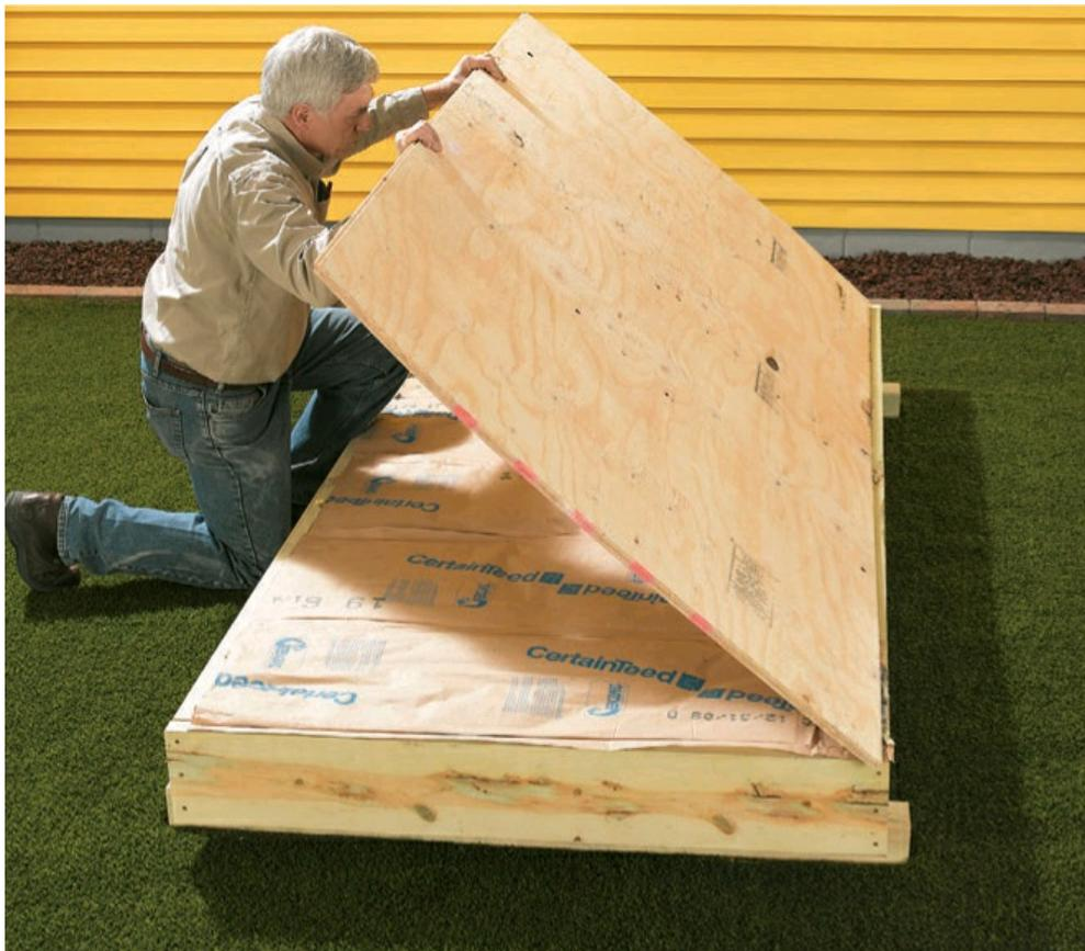
**3** Turn the frame right-side up again. Fill the cavities with insulation (use kraftfaced or add a vapor barrier). Screw the 3/4" plywood to the joists with 15/8" deck screws.
