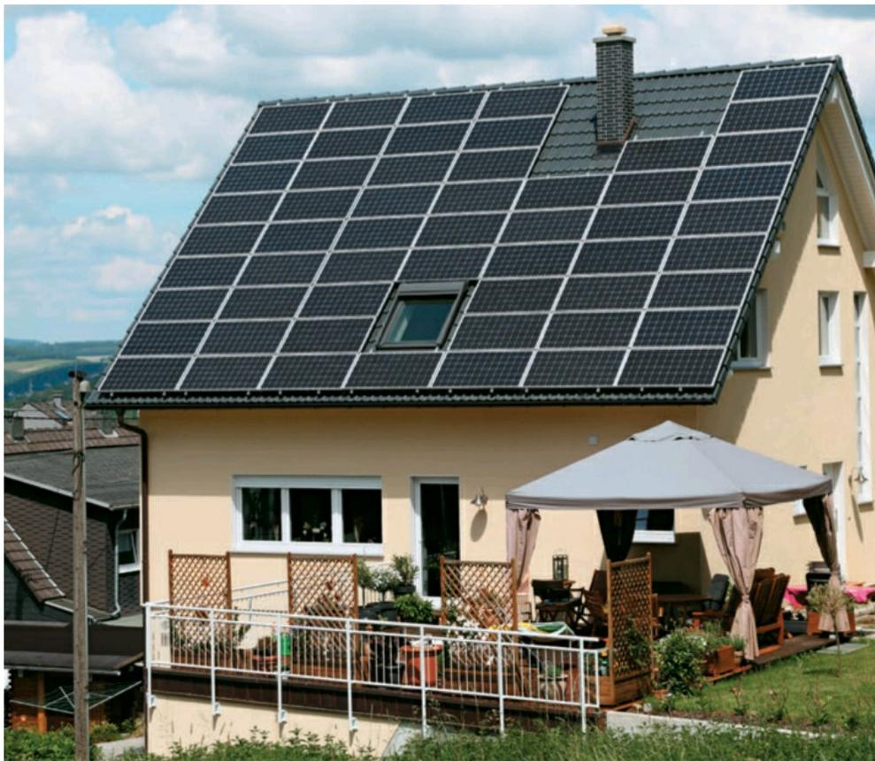
**This house is still connected** to the electrical grid, but with the entire south side of the roof covered with solar panels, the homeowner generates enough electricity on sunny days to earn money back from the utility company.
