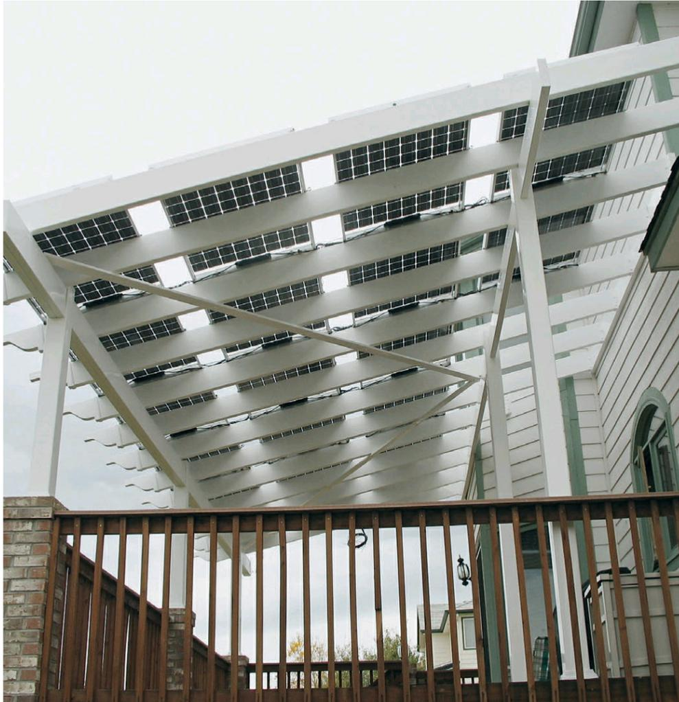
**Installing solar panels over an arbor, pergola, or other overhead structure can create a unique architectural element. Here, panels over an arbor provide shade for a patio space while generating electricity for the house.**
