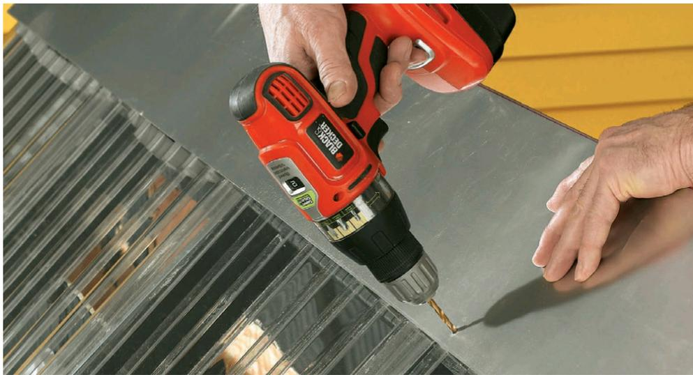
**22** Cut a 14"-wide piece of sheet-metal or aluminum coil stock slightly longer than the roof, then bend it at the center to create a cap for the roof. Drill holes through the metal, polycarbonate and closure strips in the front, then fasten with neoprene screws into the blocking. Screw the metal to the 1 × 6 in back.
