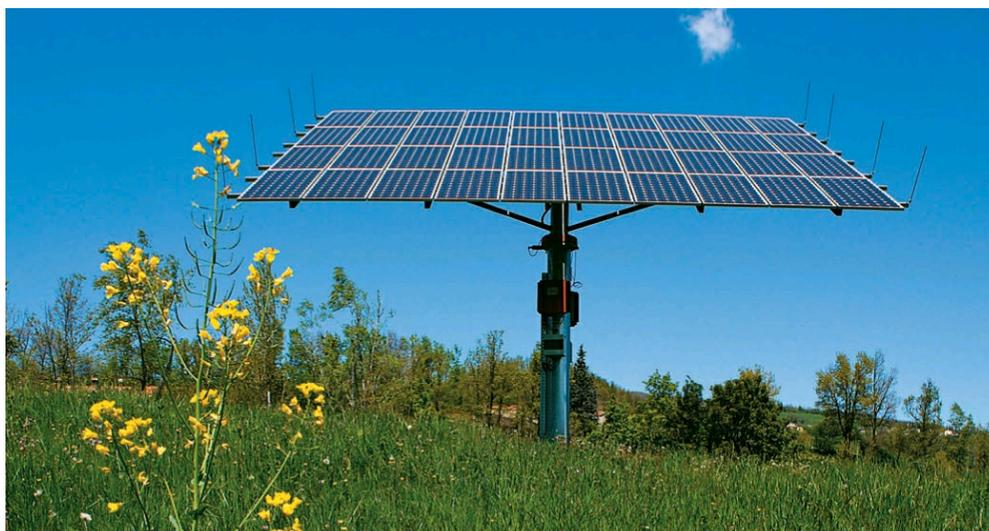
**PV panels** are often installed on heavy metal pole mounts, embedded in a cylinder of concrete and buried deep in the ground. The size and depth of the post mount for a PV panel is based on the square footage of the panel or panels, the height above the ground and local soil and wind conditions. You also need to take into account snow levels and the furthest reach of shadows cast by nearby trees and buildings throughout the year.
