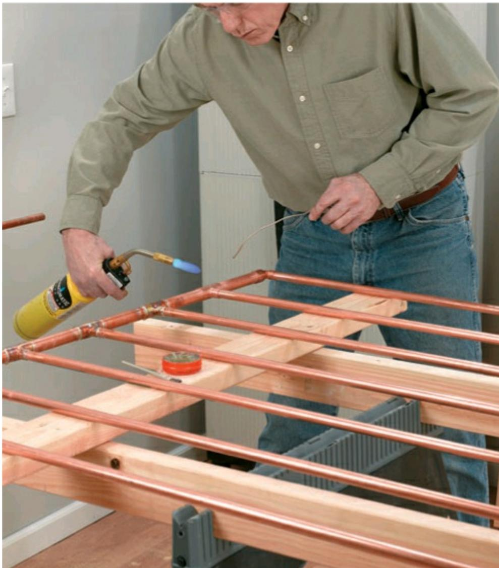
**6** Solder all the pieces together. Protect the floor from drips of solder and flux with a dropcloth. Wait at least 5 minutes to touch the
