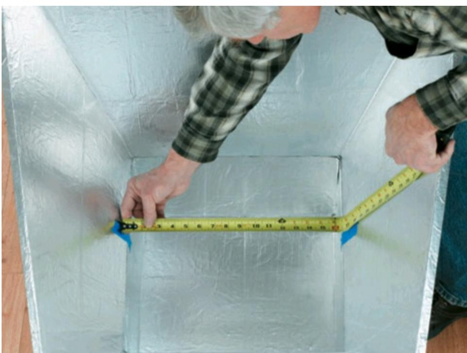
**2** Take measurements to double-check the glass lid size. Ideally, the lid will fit in so it comes to rest about 1" above the top opening of the box. As shown here, a  $1/4 \times 17 \times 17$ " piece of tempered glass fits just right. Be sure to order glass with polished edges. You can also just use a clear plastic oven bag instead of the glass. Either will trap heat and speed up the cooking.
