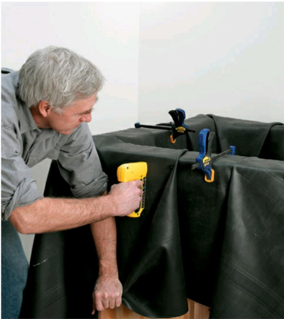
**10** Staple the rubber around the outside edge of the top  $2 \times 4$  ledge.
