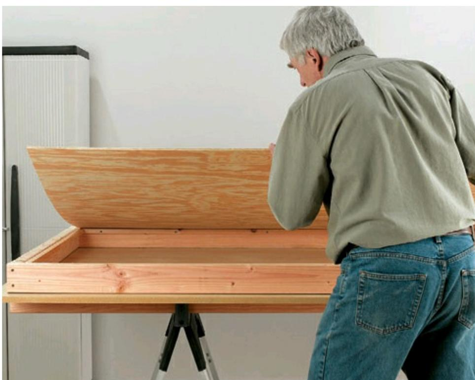
**3 Flip the frame over** and set the 1/4" plywood back into the frame against the nailers. Screw the plywood in place with 3/4" machine screws driven through the back panel into the nailers.
