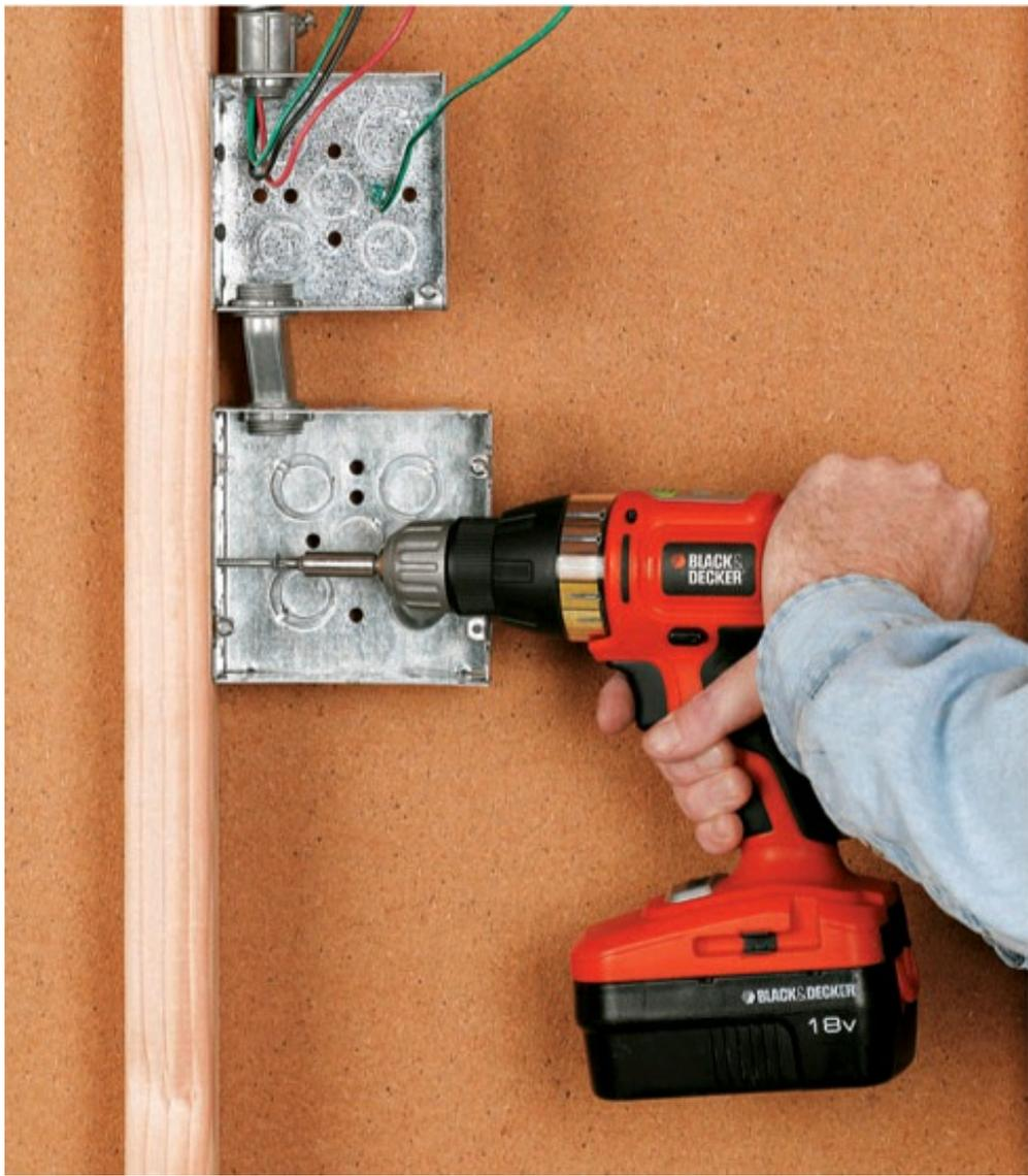
**5** Attach a double-gang metal junction box to the building's frame beneath the DC disconnect box to enclose the charge controller.
