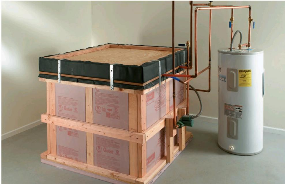
You can save money on a solar hot water system by making your own storage tank from wood, insulation and an EPDM rubber liner.
