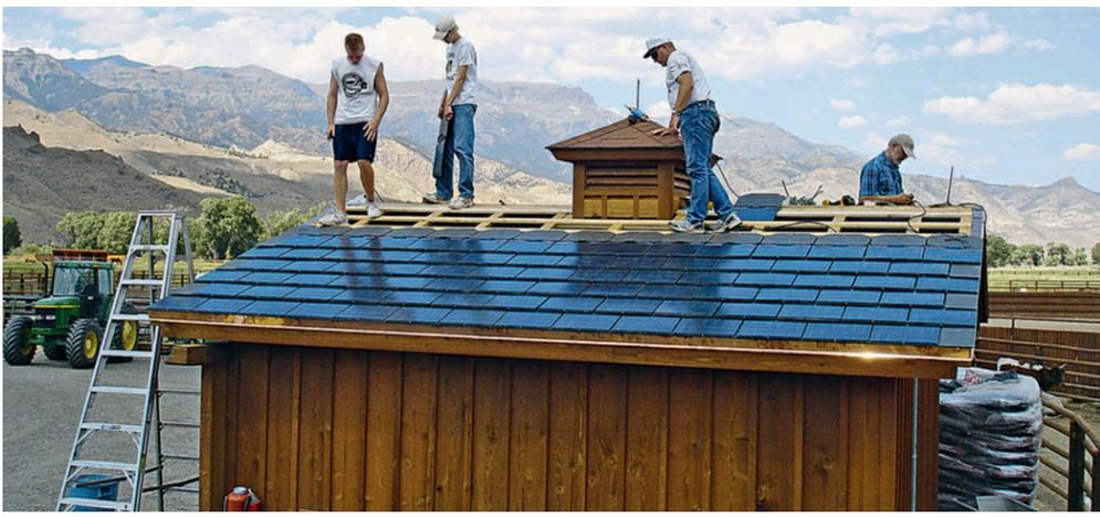
**This fiber-cement shingle roof** features an integrated array of shingles laminated with thin-film PV modules.
