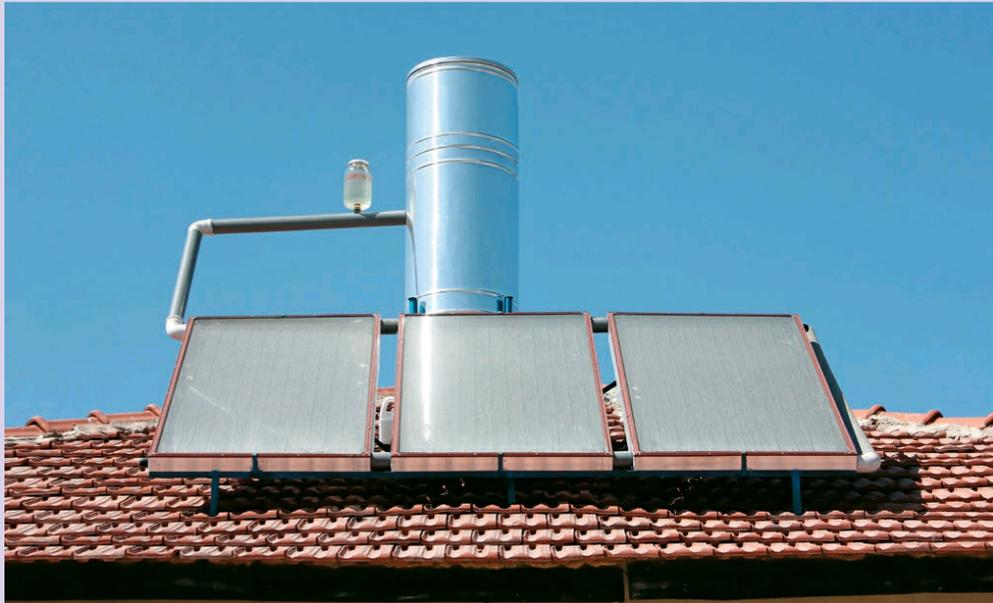
**Thermosyphon tanks must** be above the level of the collector in order for the movement of water by thermosyphoning to occur.
