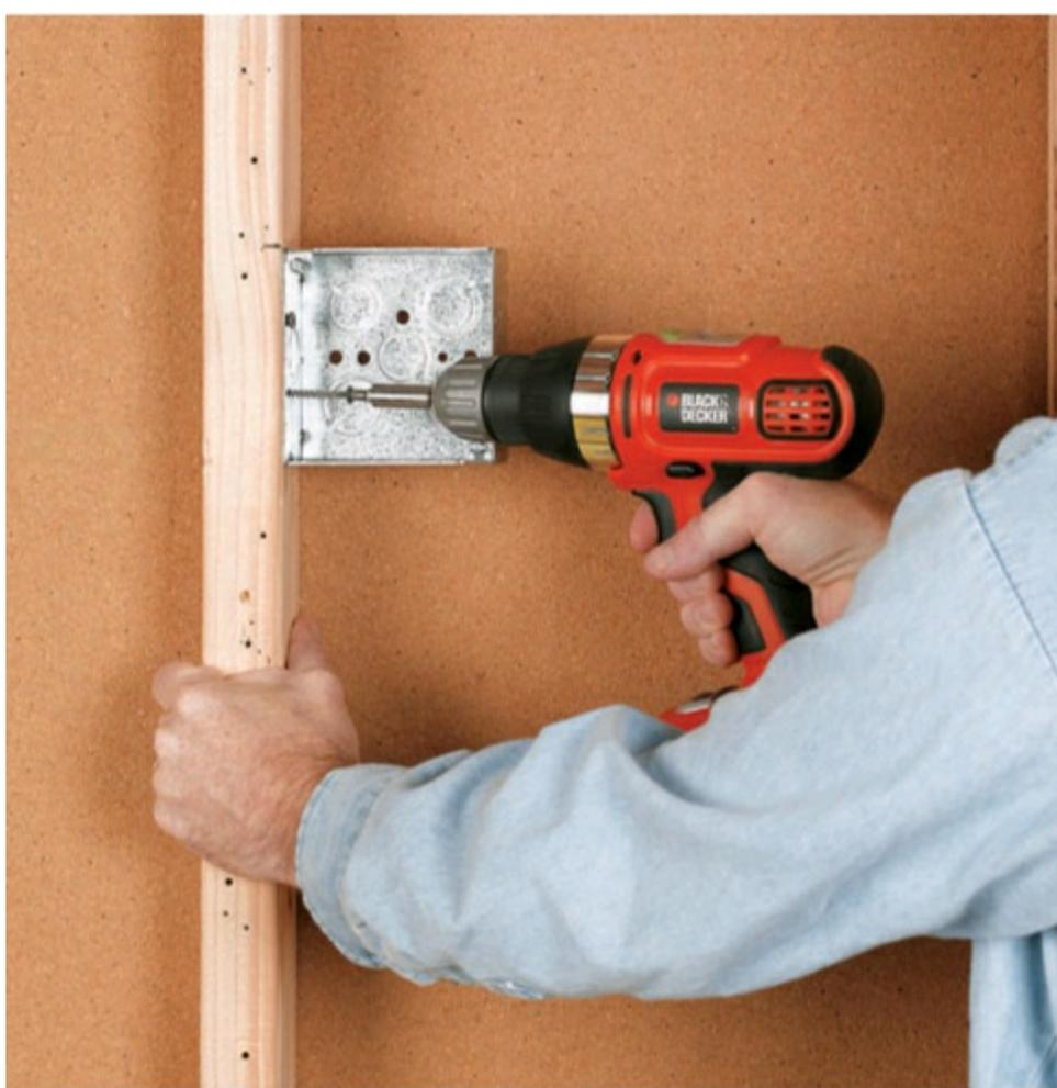
**3 Attach a junction box** for enclosing the DC disconnect, which is a heavy-duty switch, to a wall stud near the battery and charge controller location. Use a metal single-gang box with mounting flanges.
