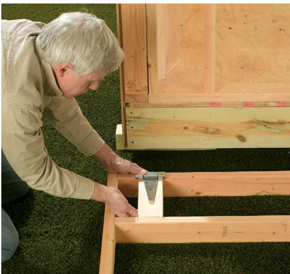
**11** **Frame the rear doors.** Make sure that the doors are 1/2" less than the height of the opening and 1/2" less (total) than the opening width. Frame openings for the vents, and add a hinge backer.
