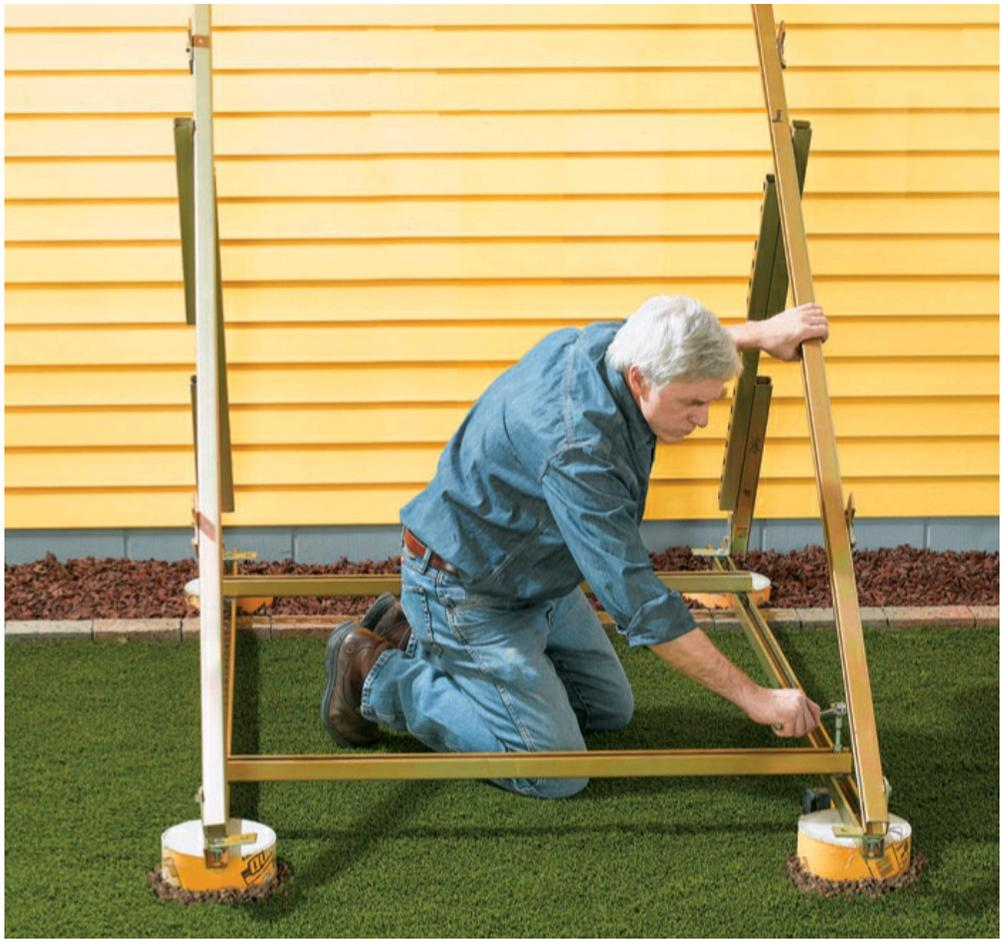
**5** Although the PV mount is stable, it needs to be securely anchored to the ground in case of high winds. For larger arrays like ours, add concrete footings at each corner.
