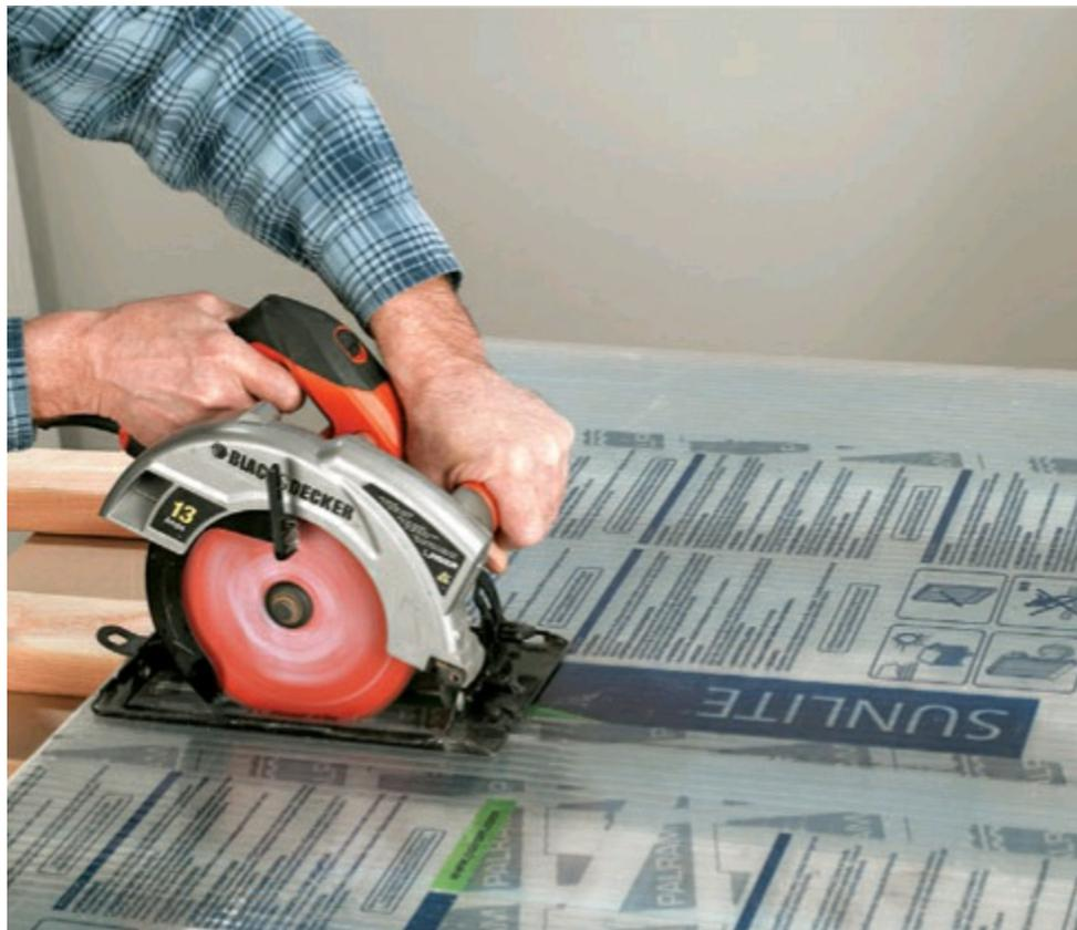
**10** Cut the **polycarbonate glazing** so that it matches the width of the box. Cut it long enough so it tucks under the overhang at the top and hangs over 1/2" at the bottom. Make sure to install it with the UV-protected side up (the side with the label).
