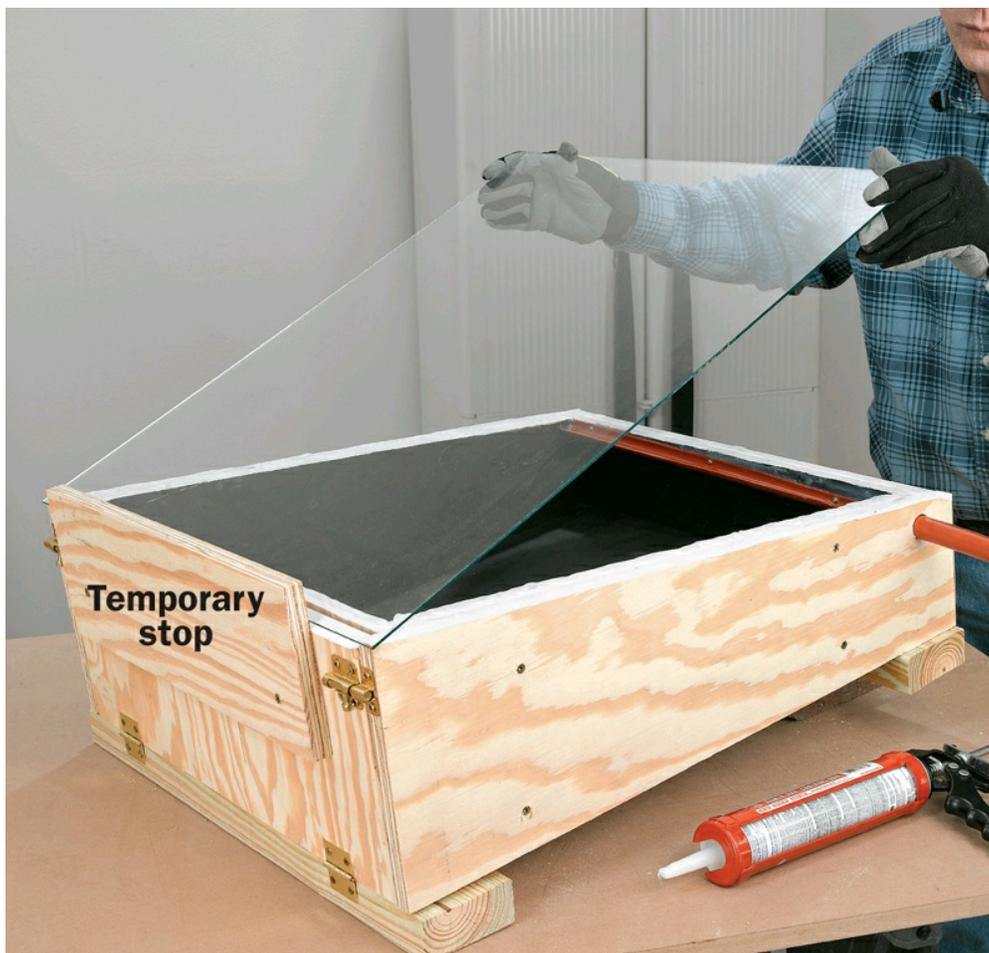
**12 Shim the box level** and tack a temporary stop to the top edge to make it easy to place the glass without smearing the caulk. Spread a generous bead of caulk on all the edges, then lay the glass in place. Tape it down around the edges with painter's tape, then let it set up overnight.
