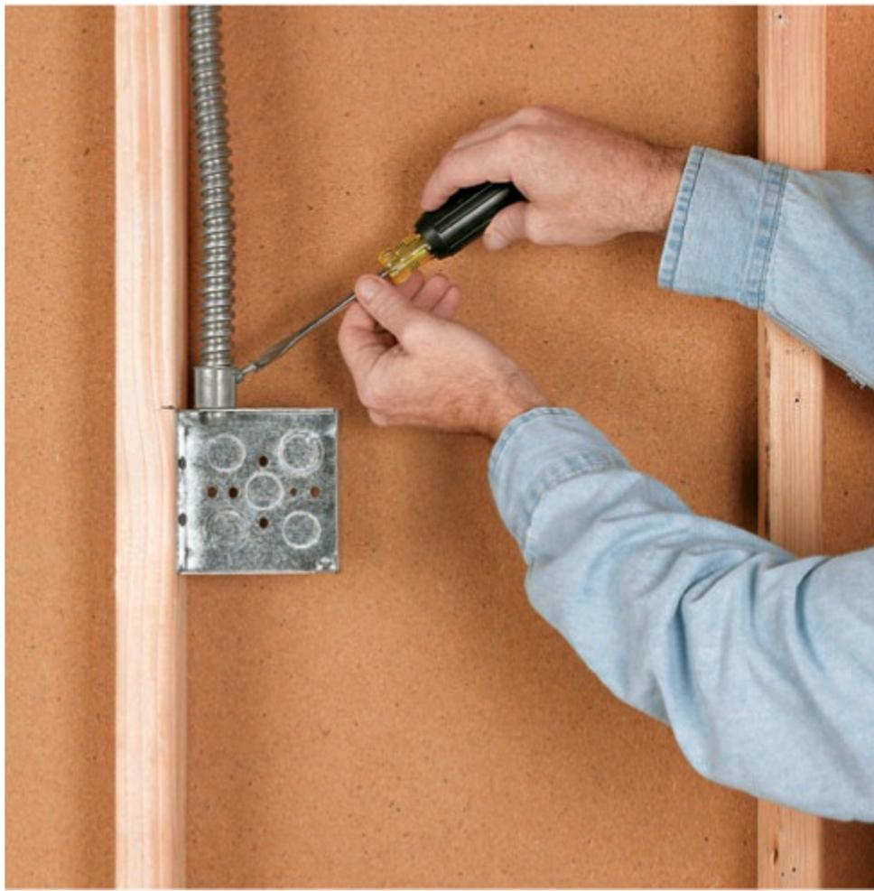
**4** Run flexible metal conduit from the entry point at the power source to the junction box for the DC disconnect box. Use hangers rated for flexible conduit.
