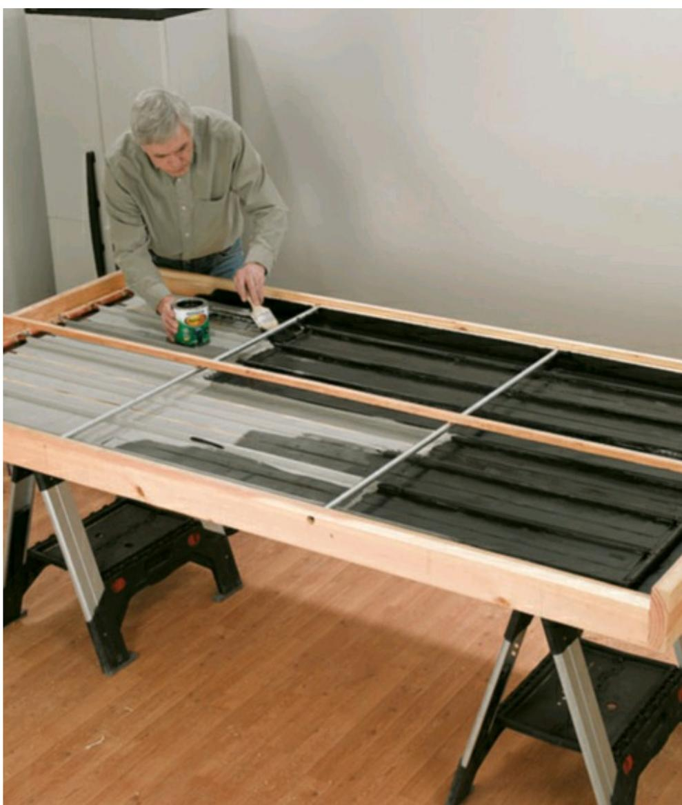
**14** Paint the entire inside of the collector with black, high-temperature paint.
