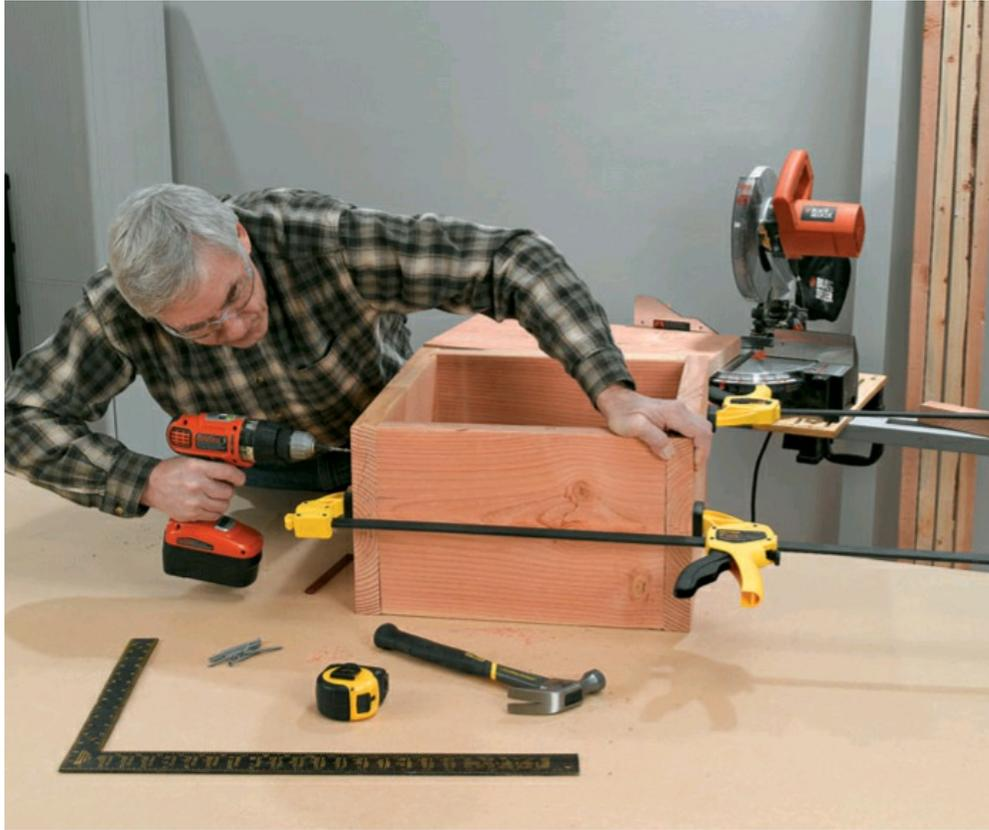
**1** Cut the four  $2 \times 12$  base pieces to length according to the cutting list. Arrange the base parts on a flat work surface and clamp them together in the correct orientation. Check with a carpenter's square and adjust the parts as needed. Then drill pilot holes and fasten the pieces together with 2-1/2" deck screws.
