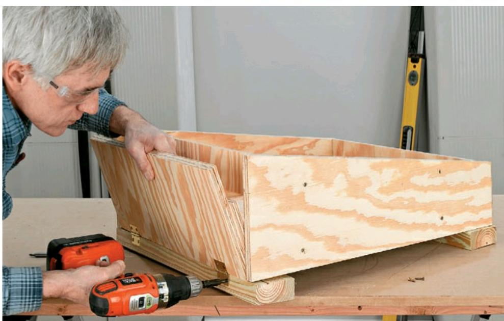
**5** Glue and screw the hinged door pieces together, aligning the bottom and side edges, then set the door in position and screw on the hinges. Add a pull or knob at the center.
