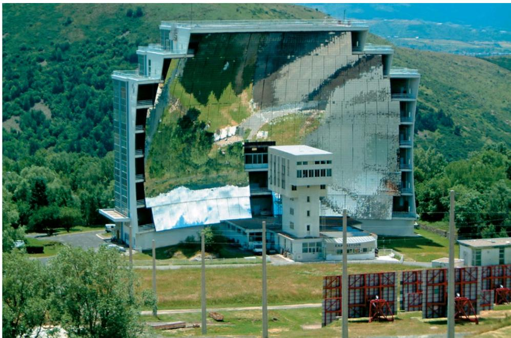
**This massive power plant** (above) and this small solar cooker (below) work on the same basic principle: Gather a large amount of light and focus it on a small area to make liquid boil. The power plant concentrates light from smaller mirrors on the hillside facing it, then focuses the light into a tight beam that can reach over 5000° F.
