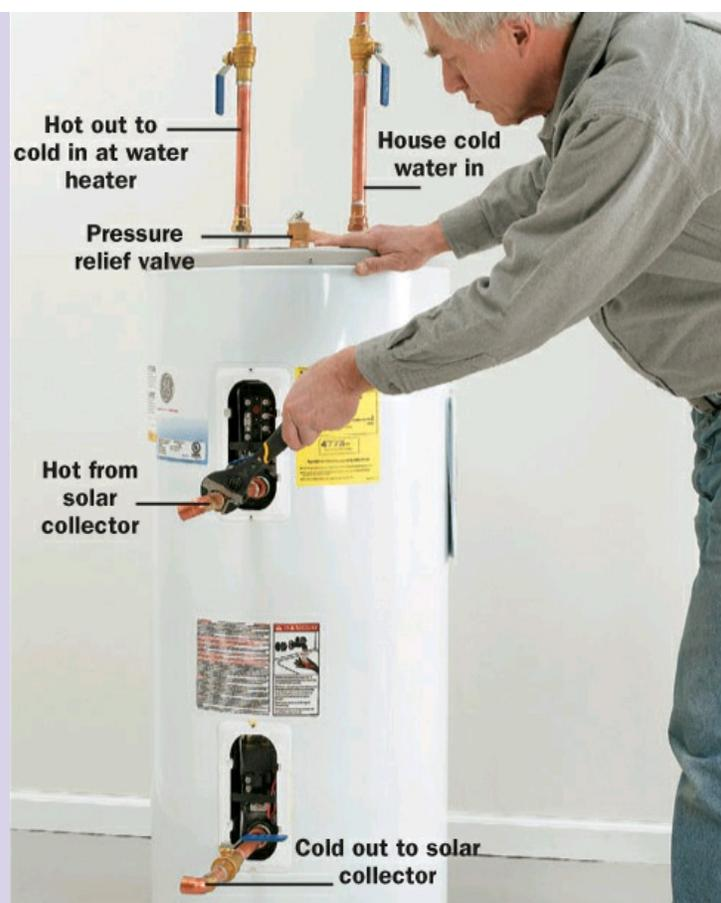
**Solder several inches of 3/4" pipe to 1 × 3/4" reducers** so you don't have to use the torch near the plastic and insulation in the water heater. After the pipes cool, wrap the fittings with teflon tape, then thread them into the water heater. Tighten with a wrench, then connect to the PEX lines coming from the solar collector. Connect the house cold water supply to the cold inlet at the top, then connect the hot output to the cold inlet at the main hot water heater.
