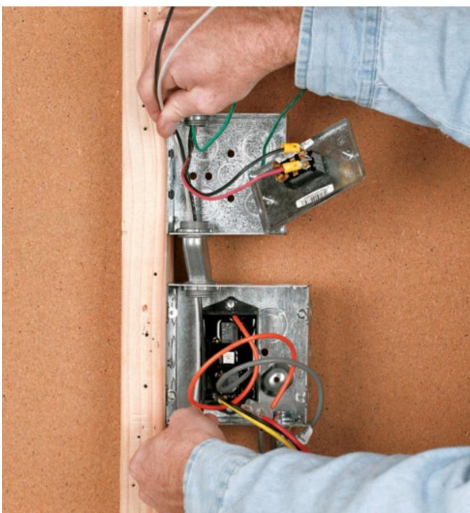
**7** **Install the charge controller** inside the double-gang box. Run flexible conduit with connectors and conductors from the disconnect box and to the charge controller box.
