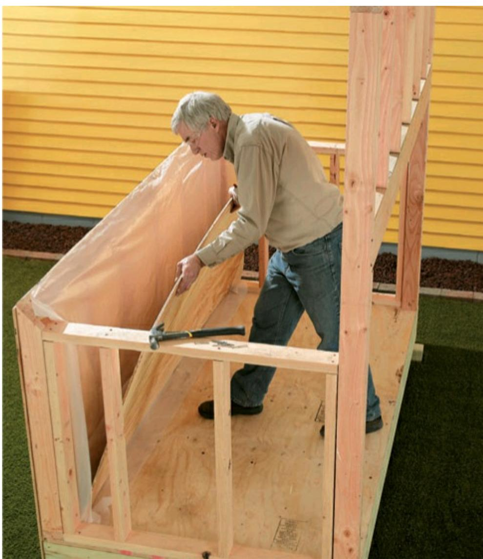
**7** Insulate the front wall, then add the vapor barrier and the 3/8" interior plywood siding. Leave the plywood 3/8 to 1/2" short of the top plate.
