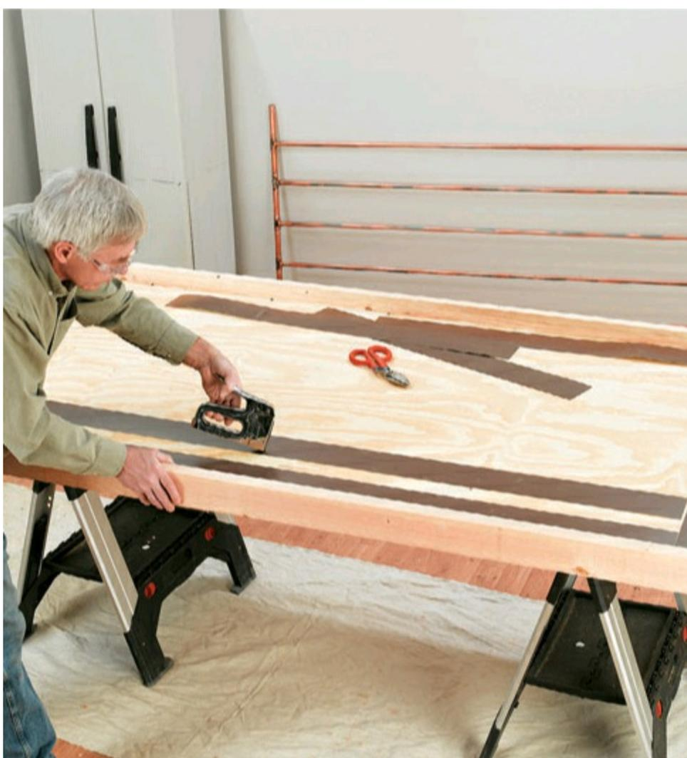
**9** Mark the manifold locations on the plywood, then cut 4"-wide pieces of aluminum flashing and staple them so they are centered under each length of copper. These will help transfer the heat to the copper pipes. Use stainless-steel staples.
