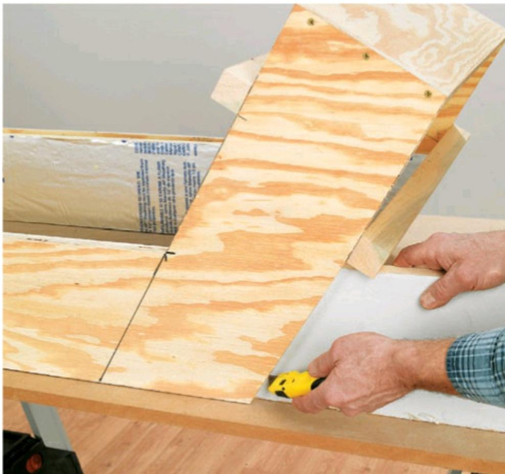
**4** Line the sides and ends with 1" polyisocyanurate insulation. Leave the foil side facing into the box and glue the insulation in place with construction adhesive. Wrap the exposed upper edges with aluminum foil tape to protect the insulation from UV rays. Cut the insulation 1/4" narrower than the plywood sides so that the bottom piece of 1/4" plywood will fit in between the sides.
