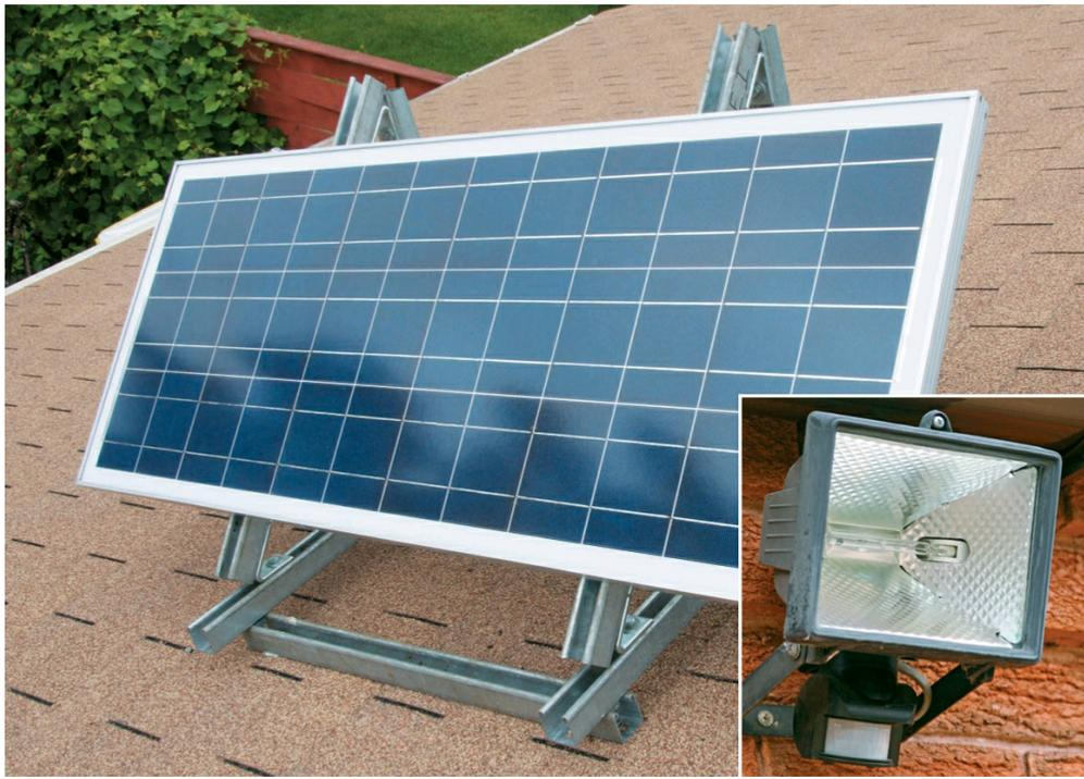
**This 60-watt solar panel** is mounted on a garage roof and powers a self-contained home security lighting system. Not only does this save energy costs, it keeps the security lights working even during power outages.
