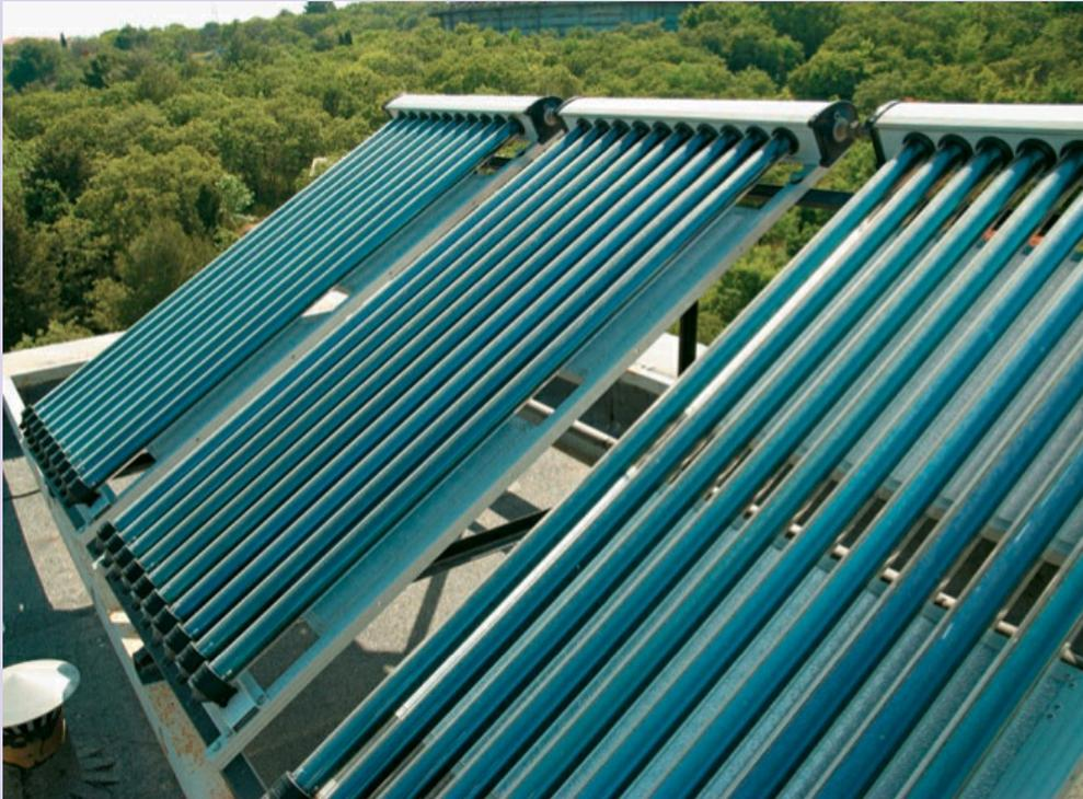
**Evacuated-tube collector:** This type of collector has to be purchased from a supplier, although homeowners can install it. Water pipes in this system, instead of running through an insulated box, are installed inside a round tube of insulated glass. The vacuum inside the insulated glass allows light through, but slows heat loss. Evacuated-tube collectors are more efficient than flat-plate collectors in partially sunny or cloudy conditions.
