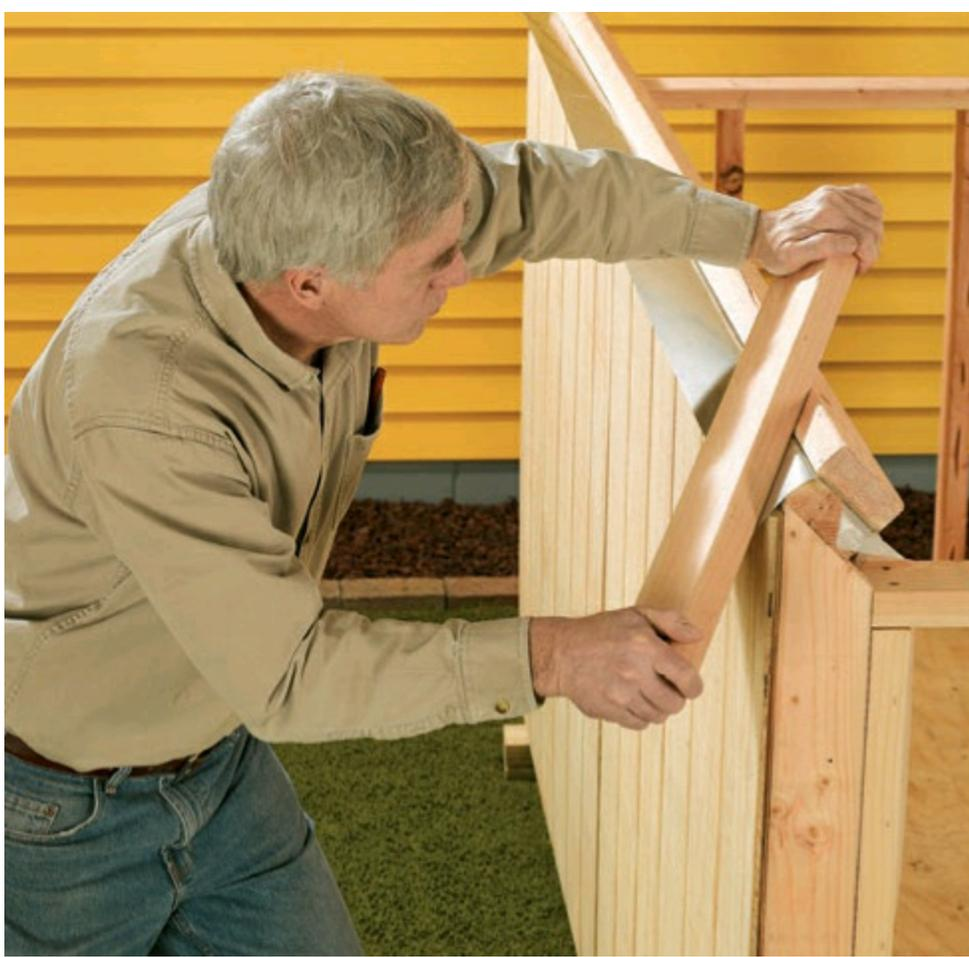
**8** Nail the coil stock to the top plate, leaving a 3" overhang on each side. Screw a 2 × 4 over the coil stock, matching the top plate position, then bend the coil stock over the edges and nail it in place. (Gutter repair tape or a strip of EPDM roofing can be used instead of coil stock.)
