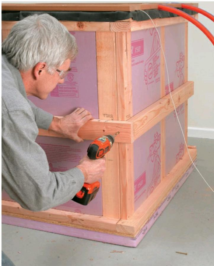
**14** Place 1-1/2" pieces of insulation on the sides, then install horizontal 2 × 4s around the center. If desired, you can add additional pieces of insulation above and below the 2 × 4s, then cover the sides with 1/4" plywood for a finished appearance.
