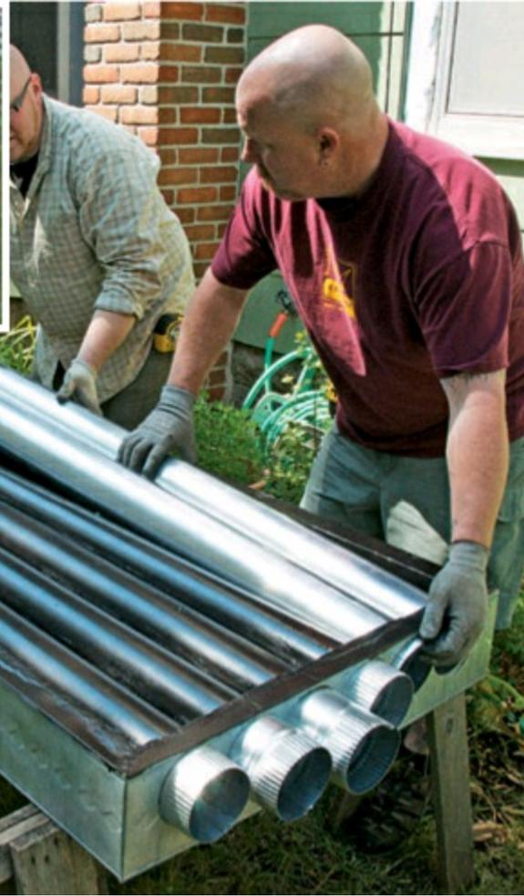
**10 Insert the ductwork.** Beginning at the inlet duct, guide 4" aluminum HVAC ductwork in a serpentine shape throughout the entire multi-panel installation, ending at the outlet duct. Join ends of adjoining duct sections with flexible duct connectors fashioned into a U shape and secured with metal screws and foil tape (inset). Paint each section of ductwork with black high-temperature paint once it is in place.
