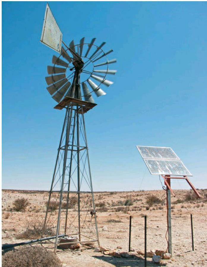
**Once powered by a windmill** that needed frequent maintenance, this deep well, which pumps water to a nearby stock tank, is now powered directly by solar panels. Instead of pumping on demand, the motor pumps water continuously when the sun is out and stores it in a large tank.
