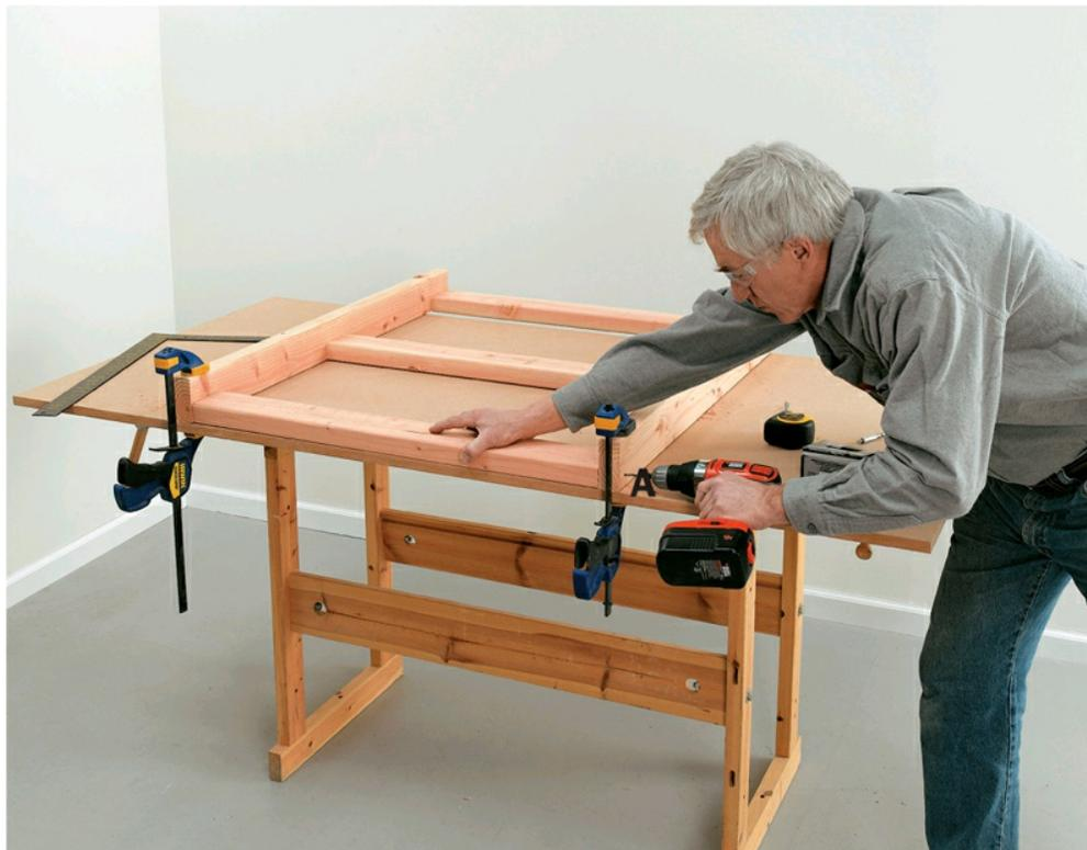
**1** Screw two of the 41" 2 × 4s to three vertical 2 × 4s, then fasten the 41"-wide piece of 1/2" plywood to the 2 × 4s with construction adhesive and 1-5/8" screws. Repeat for the opposite side. Align the bottom edge of the plywood with the bottom 2 × 4; the top edge will overhang 1-1/2".
