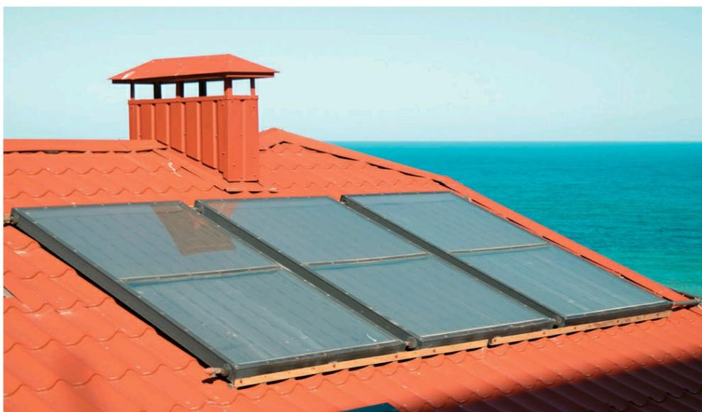
**Arrays of hot water collectors** are ganged together at the top and bottom. Cool water flows in at the lower right at one end of the array, and heated water flows out at the upper left. This system is controlled by a pump inside the house.
