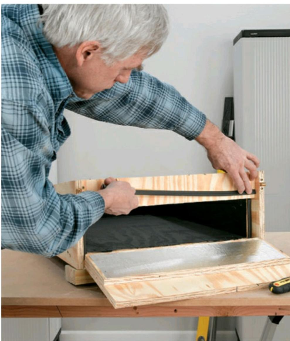
**7** Apply weatherseal around the edges of the hinged door to make the door airtight.
