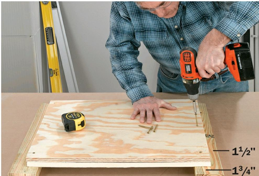
**2** Cut the insulation the same size as the plywood base, then screw both to the 2 × 4 supports with 2-1/2" screws.
