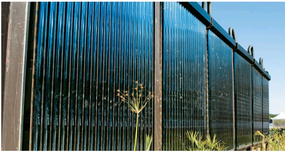
**The evacuated-tube hot water collectors** mounted to the side of this house in the desert collect abundant hot water for bathing and heat. Evacuated tubes are well-enough insulated that they can survive an occasional cold snap.
