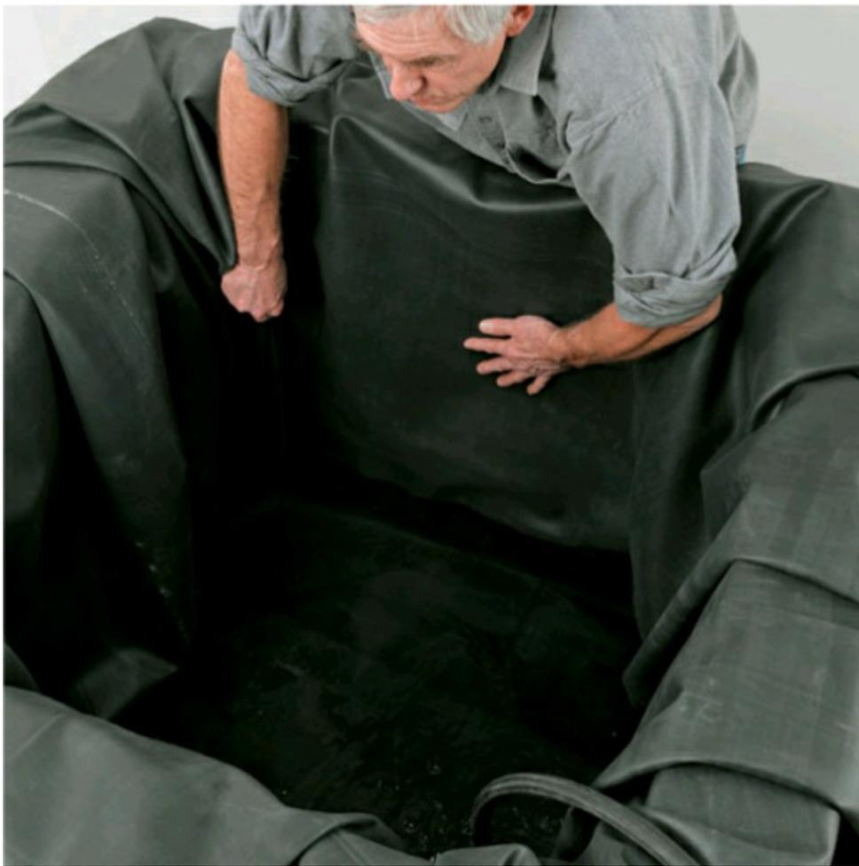
**8** Cut and set aside a 5 × 12-ft. piece of the EPDM for the top, then fold the remainder into the tank. Work it into the corners, leaving the rubber loose at the bottom so it doesn't stretch with the weight of the water. Add 6" of water to hold the rubber in place as you fold over the corners. Drape the excess over the sides.
