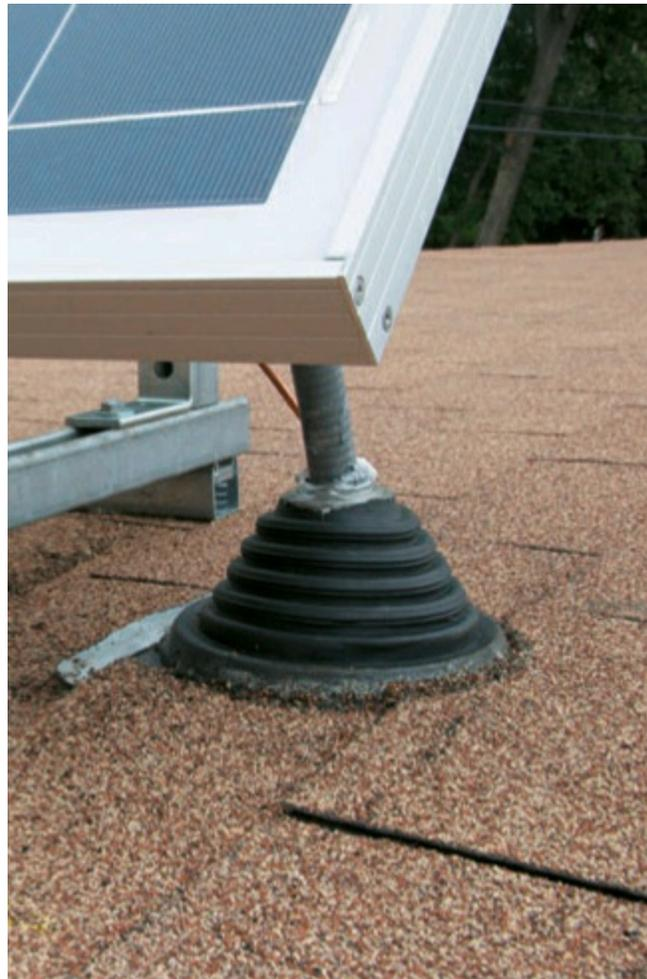
**An EPDM rubber boot seals** off the opening where the PVC conduit carrying the feed wires penetrates the roof.
