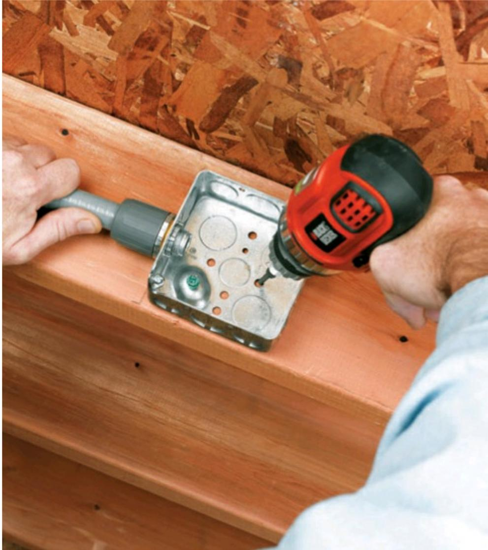
**1** **Mount a junction box** inside the building where the conduit and wiring enter from the power source. Secure the box to the conduit with appropriate connectors. Run two 14 gauge wires through the conduit and connect them to the positive and negative terminals on the panel.
