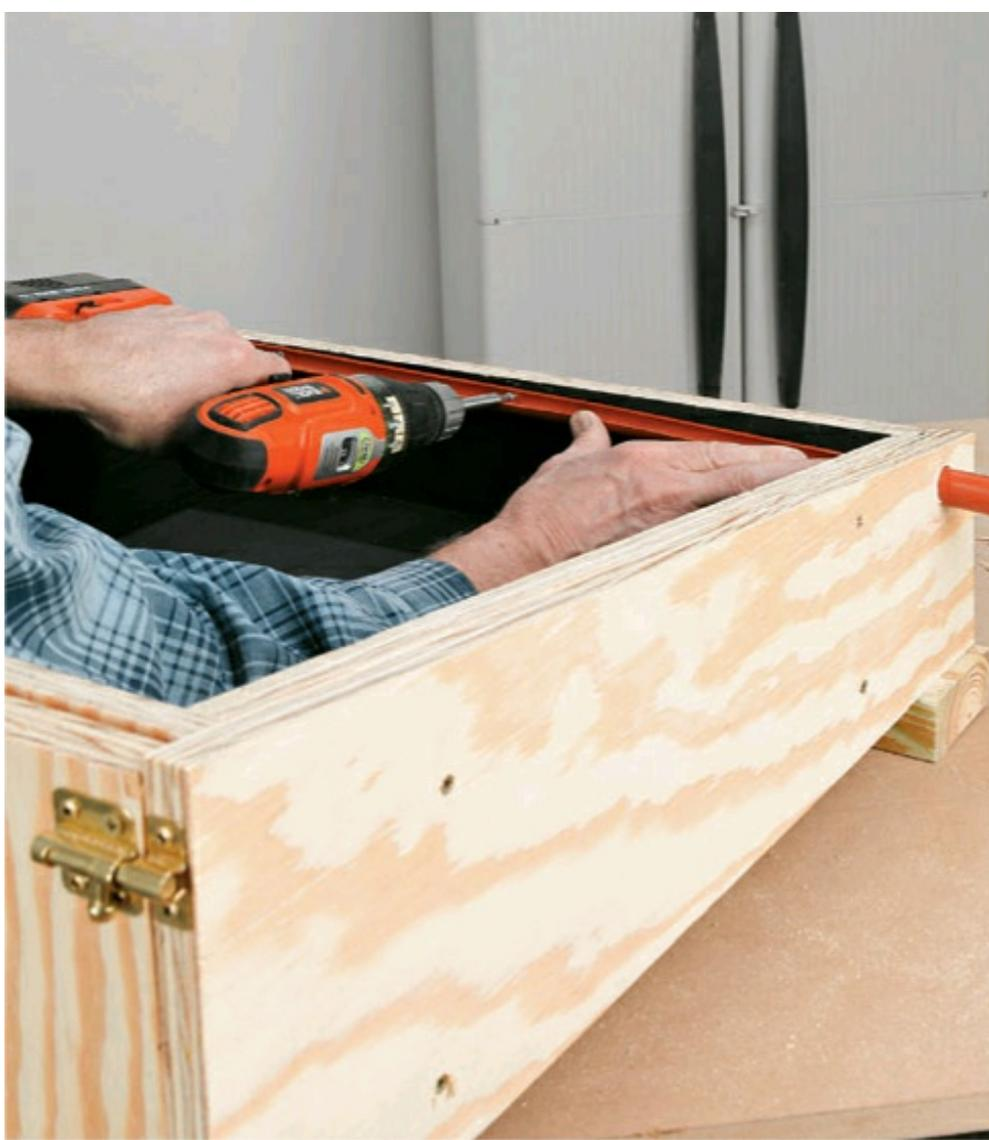
**10** Drill three 1/8" holes in the side of the PEX for screws, then insert the PEX through the hole. Butt it tight against the other side, then screw it in place, sloping it about 1/4".
