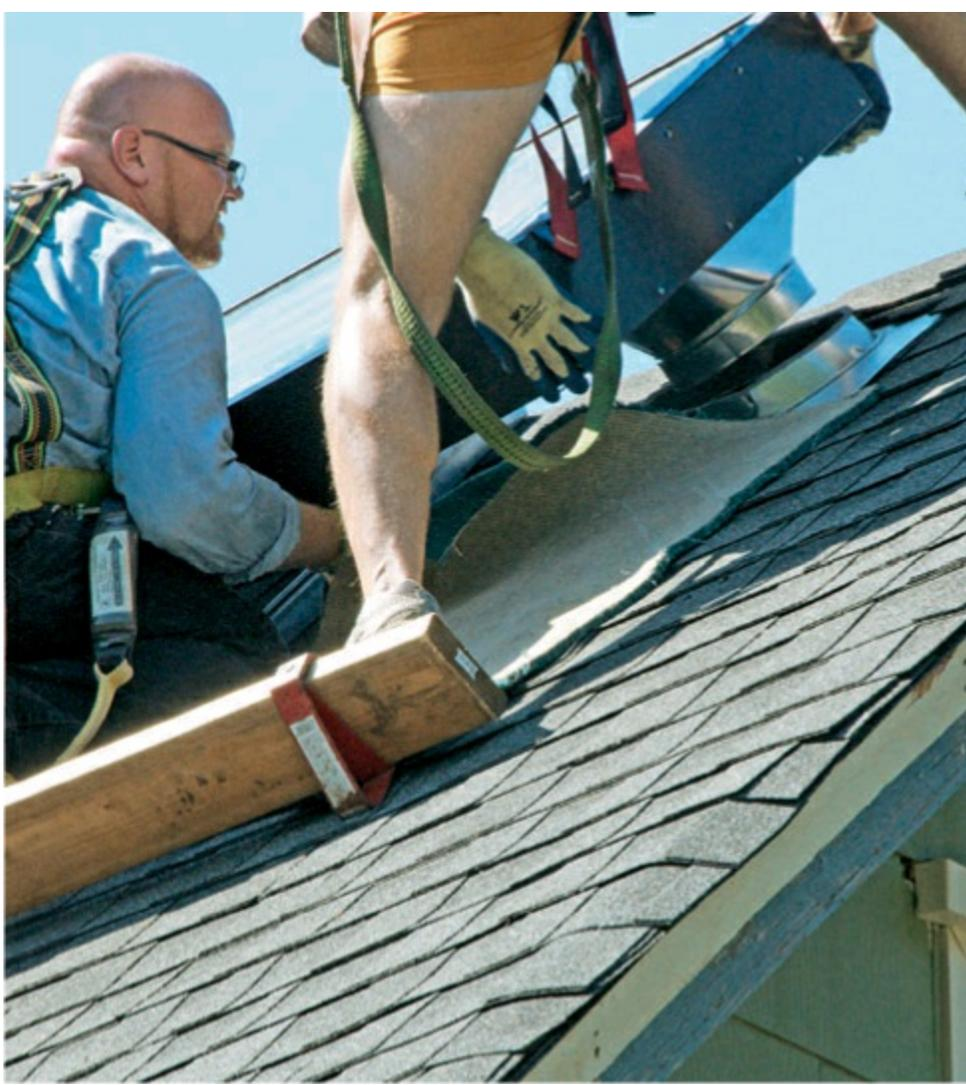
**18** Connect the inlet and outlet ducts on the panel(s) to the openings on the roof. Position the panels so the inlet and outlet openings match perfectly, and attach with a duct collar and silicone caulk.
