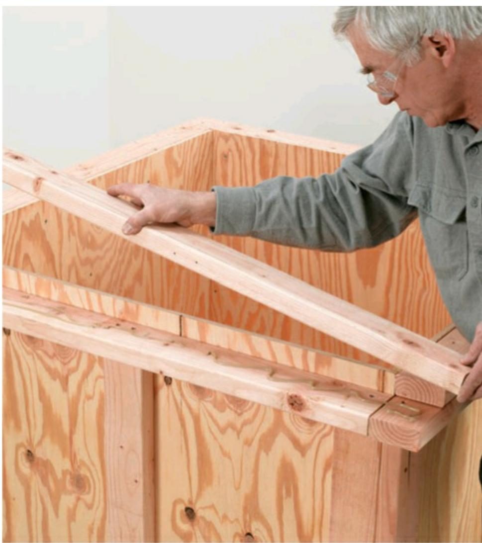
**6** Glue the 2" foam base to the plywood base with construction adhesive, then turn the box right-side up and add the second layer of 2 × 4s to the top, overlapping the corners for strength. Screw the plywood walls to the final layer of 2 × 4s.
