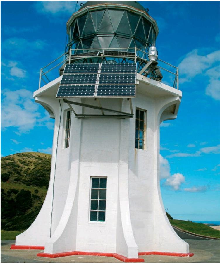
**An array of solar panels** and a bank of batteries replaced the noisy, smelly generator that formerly powered this remote lighthouse.
