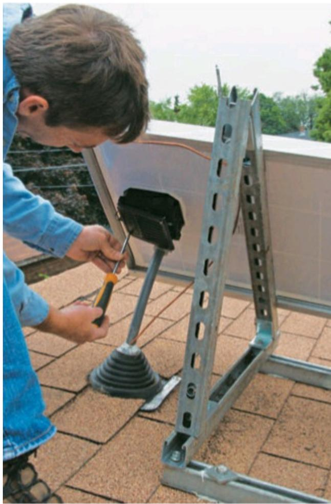
**Connections for the feed wires** that carry current from the collector are made inside an electrical box mounted on the back of the collector panel.
