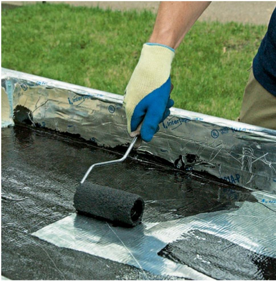
**9** Paint the entire box interior using black high-temperature paint and allow it to dry completely. A trim roller works well for this task.
