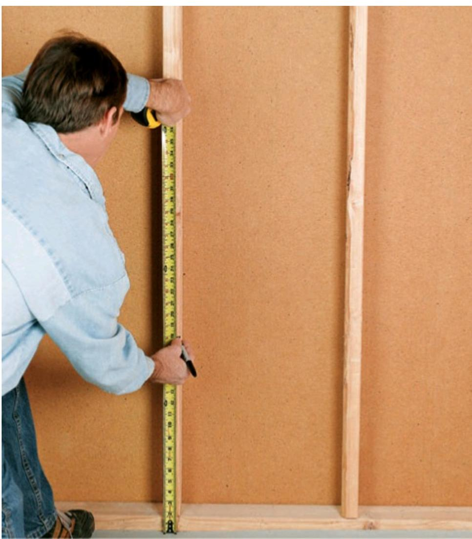
**2 Plan the system layout.** Determine the placement of the battery and then decide where you will position the charge controller and DC disconnect. The battery should be placed at least 18" off the ground in a well-ventilated area where it won't be agitated by everyday activity. Mark locations directly on the wall.
