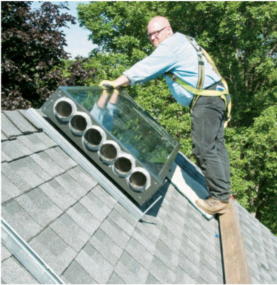
**20** Seal the **panel connections** with 1" foam gasket tape around each end of the panels where they connect. Place a bead of silicone caulk on top of the gasket tape and then attach 3"-wide flashing over the two panels at the joint. Attach flashing to the panel with galvanized sheet-metal screws with rubber gasket heads.
