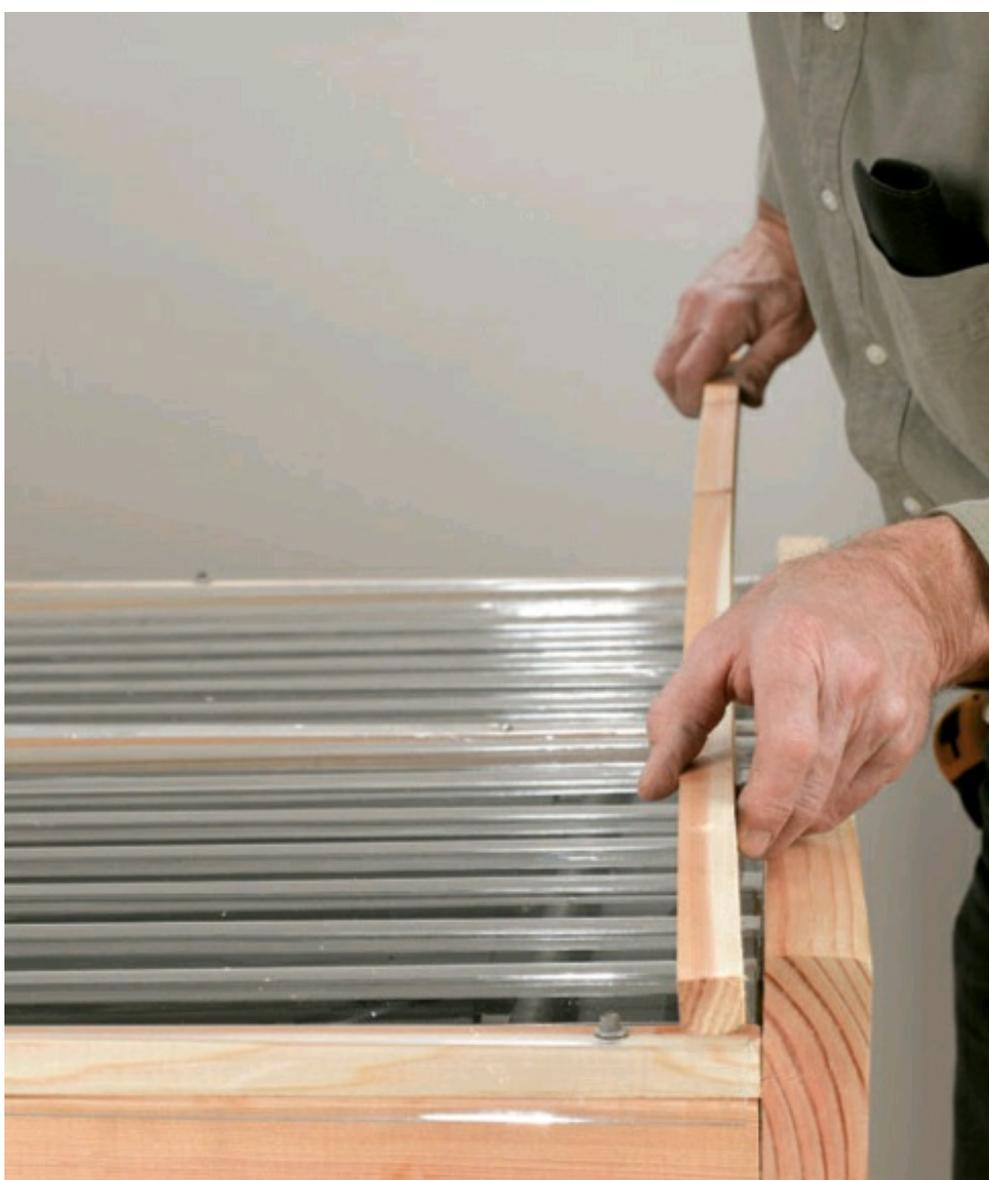
**16** Cover the ends of the glazing with 3/4" wood strips. Pre-drill and fasten the strips with 2-1/2" deck screws. Caulk the strip at the top against the 2 × 6 cap using paintable acrylic caulk.
