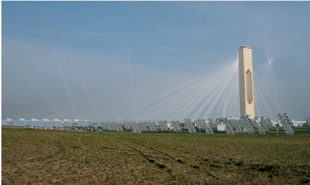
**The light from hundreds of solar reflector panels** is focused at the top of the tower, creating steam to power turbines that generate electricity for thousands of homes.
