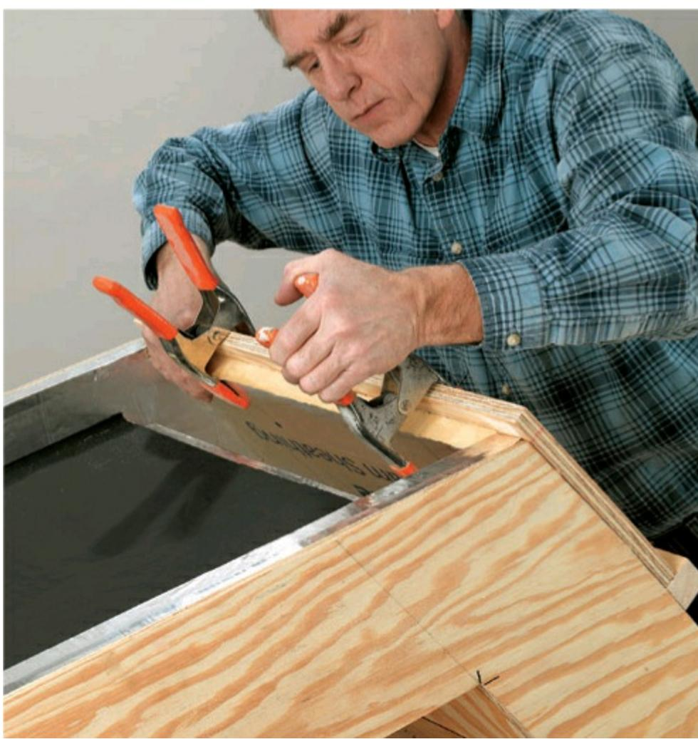
**9** Cut and install 1" insulation to fit the angled top, from the 2 × 2 to the outside corner. Caulk any gaps along the sides. Spread a bead of glue on the insulation, then cover it with 3/4" plywood screwed across the top, and extending from the 2 × 2 to 1" beyond the outside corner. Clamp the plywood and insulation until the glue sets.
