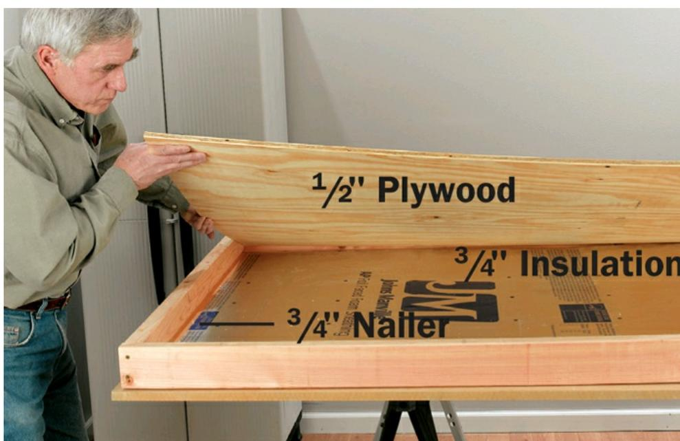
**4 Cut panels of 3/4"-thick closed-cell, foil-faced insulation** and fit them inside the frame between the 3/4" nailers, flush with the tops of the nailers. Cut a panel of 1/2" plywood to fit inside the frame over the insulation and the nailers and attach the plywood to the nailers, driving a 1-1/4" screw every 10 to 12" around the perimeter. Caulk the gap between the 1/2" plywood and the frame with clear, 100% silicone caulk.
