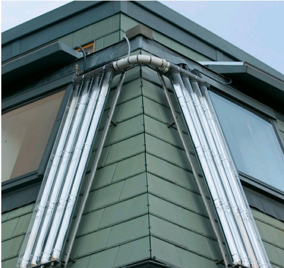
**An unusual roof style** and a NE/SW building orientation called for a creative mounting solution for this evacuated-tube solar hot water collector.
