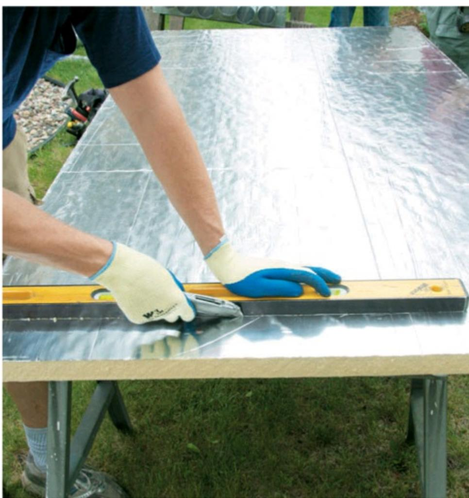
**4** Cut the foil-faced rigid foam insulation to match the interior dimensions of the box, using a drywall saw or a utility knife.
