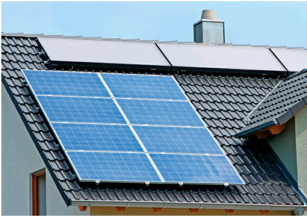
**Solar panels are combined** with solar hot water collectors (the panels along the ridge) to provide electricity, hot water and heat for this home.
