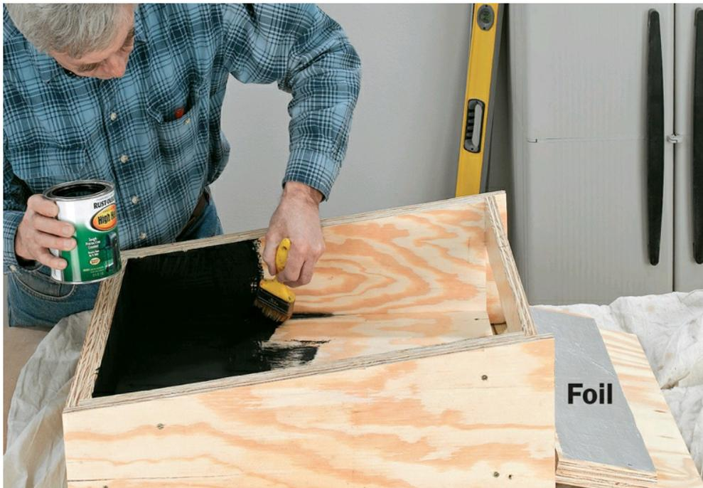
**6** Paint the inside of the box with black high-temperature paint. Cover the back and the door with reflective foil glued with contact cement. Let the paint dry for several days so that all the solvents evaporate off.
