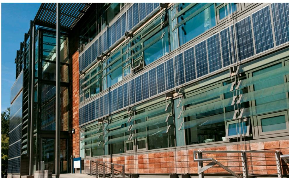
**PV panels are used** as an architectural element in this office building, along with the louvered glass and metal panels that shade the south-facing offices from the midday heat.
