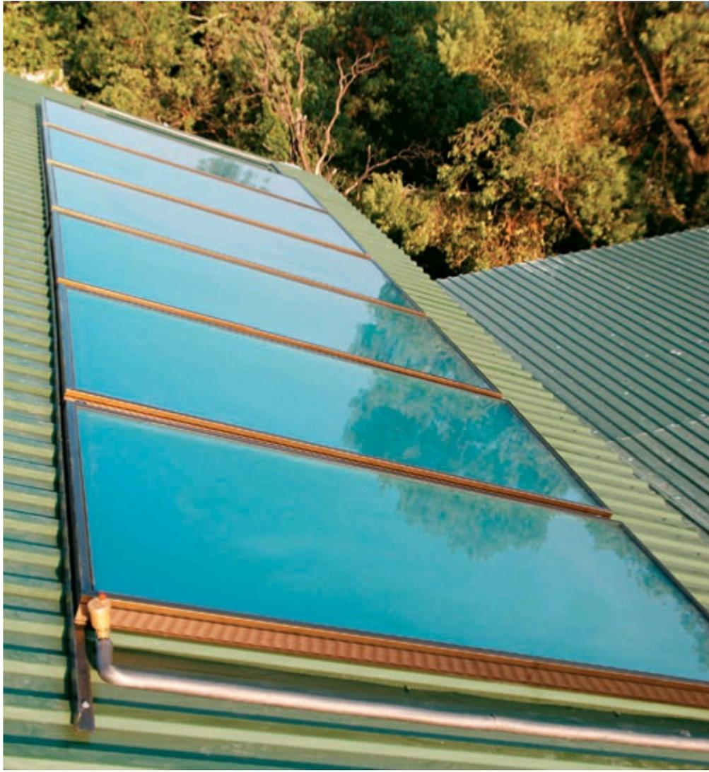
**Solar panels and collectors** can be fastened to corrugated metal roofs without expensive standoff systems, since rainwater just drains underneath.
