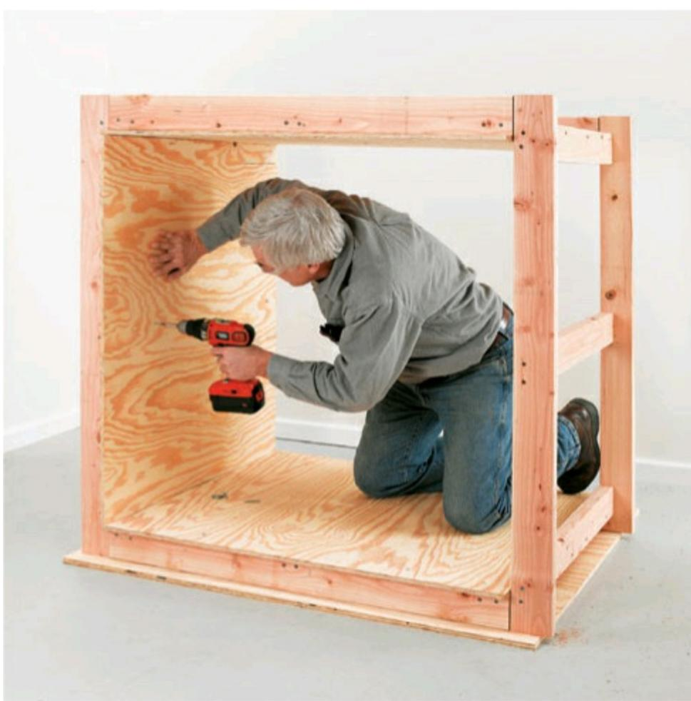
**4 Turn the box on its side.** Fasten the plywood sides in place on the long walls, taking care to align corners and edges. Check the box for square as you assemble it.
