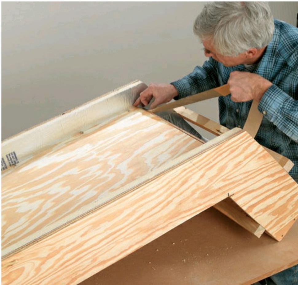
**6** Fasten 1/4" plywood to the top of the 1 × 3 to divide the incoming cool air from the hot air. Leave a 3" gap at the lower end of the plywood for air flow. Butt the two pieces of plywood together at the bend, then cover the small gap with a double layer of aluminum tape. Caulk the gaps at the end and at the corners of the insulation.
