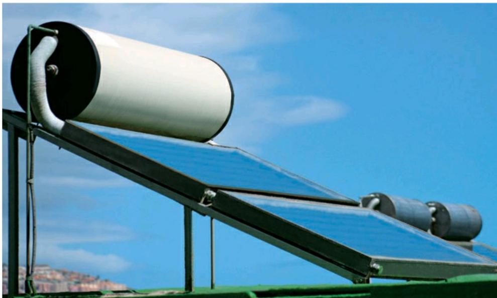
**In this thermosyphon hot water collector,** heated water rises into the storage tank at the top and then flows into the house as needed. This simple system is widely used in warmer parts of the world where freezing temperatures are not a problem.
