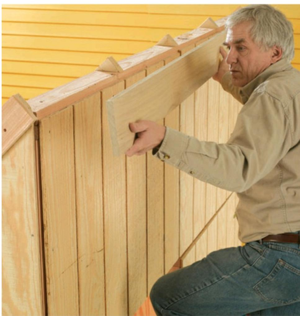
**18** Form the top of the kiln by extending the 1 × 4 diagonal trim to the edge of the framing, then join the two sides of the kiln with a 1 × 6 cap. Nail on triangular blocks for nailers and to help support the peak of the roof.
