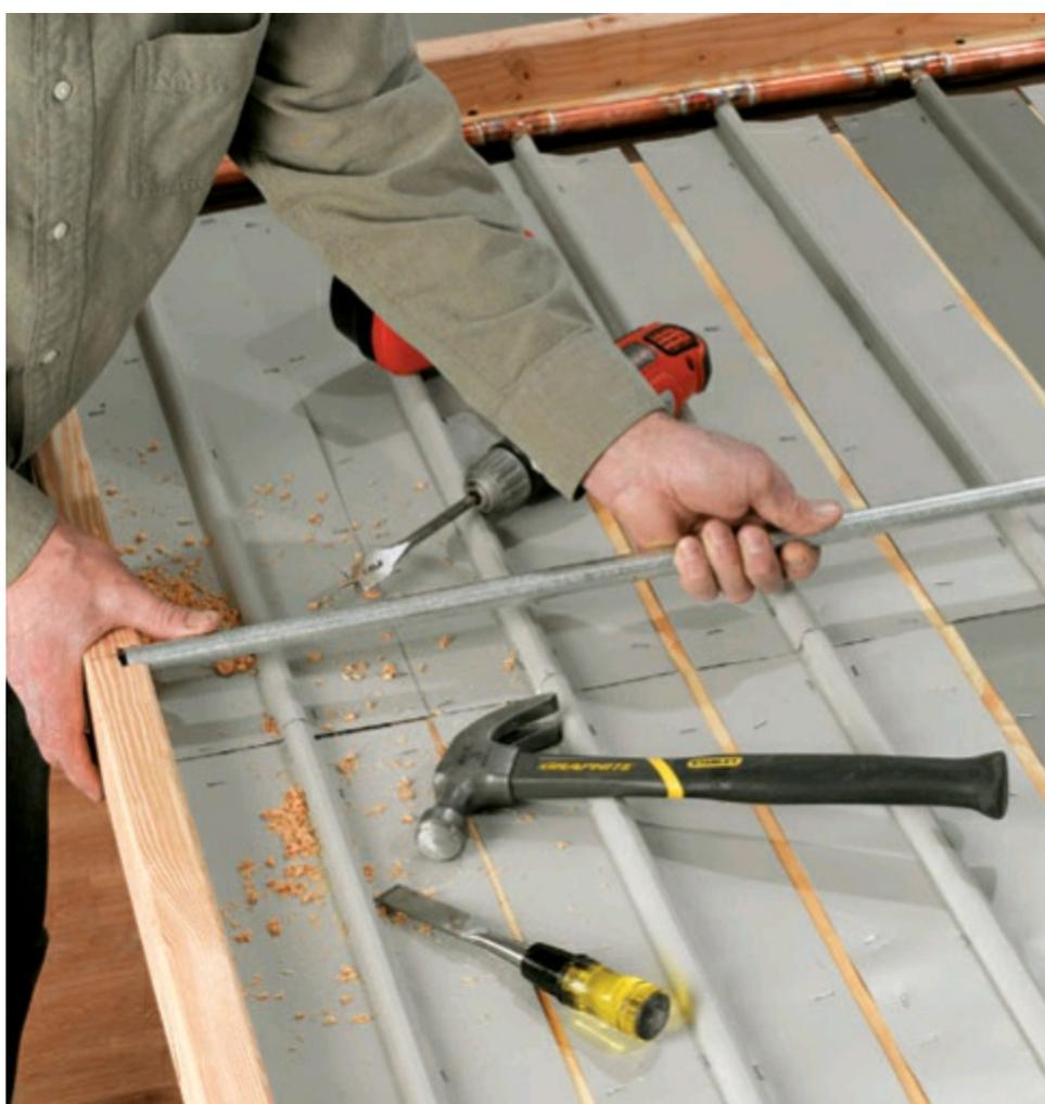
**12** Create cross-bar supports for the polycarbonate glazing by installing two lengths of 1/2" EMT conduit across the box. Drill 3/4" holes halfway through the 2 × 4 sides, centering the drill bit 3/8" down and drilling from the inside. Square the holes with a chisel, then place the conduit in the holes.
