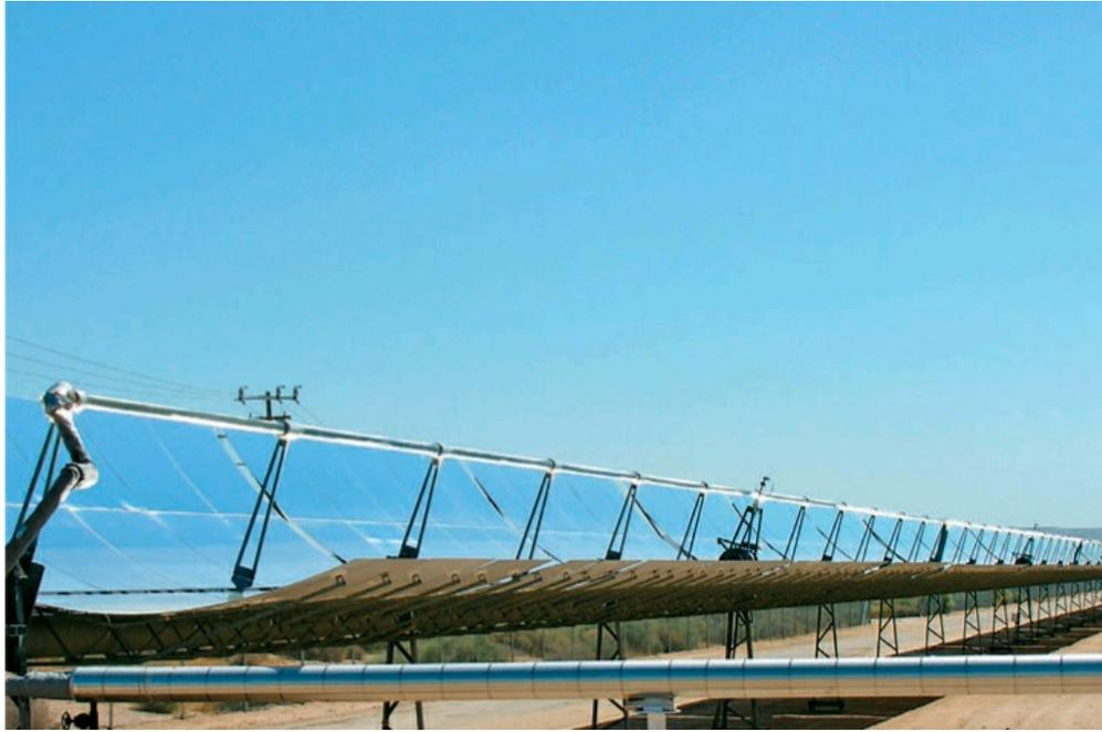
**This solar collector** uses parabolic reflectors to heat oil passing through a pipe to 750° F. This hot fluid is then used to boil water and generate steam, which powers turbines that create electricity. This power plant has been in operation since 1985.
