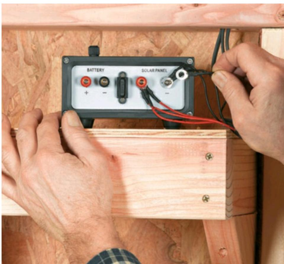
**8** **Connect the wires** from the PV panels to the solar terminals on the back of the regulator/charge controller. Secure the wires to the walls or roof framing members to keep them clear. **CAUTION:** The collector panels should be covered with a drop cloth or opaque material well before making these connections. Tape or clamp the drop cloth so it doesn't blow off.
