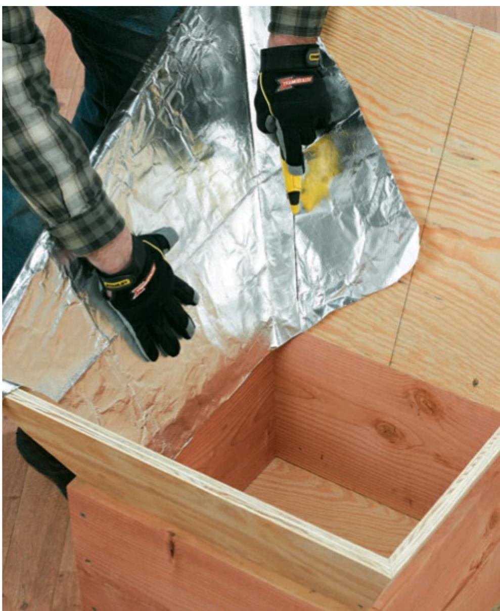
**10** Cut pieces of reflective sheeting to fit the sides of the reflector as well as the base. You can use heavy-duty aluminum foil, but for a sturdier option try solar foil (see Resources, [page 152](#)). The product seen here is essentially polyethylene tarp material with a reflective aluminum surface. Make sure to cut the pieces large enough so they overlap the edges and can be easily attached.
