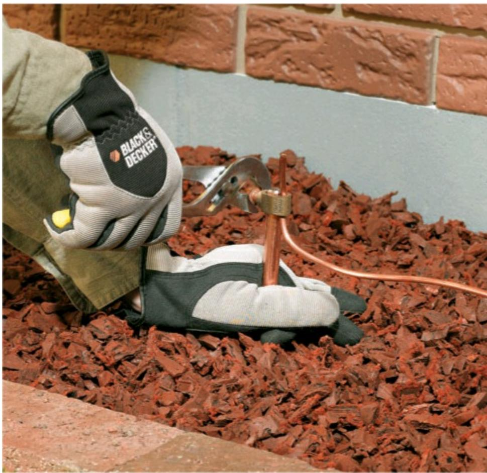
**10 Set up grounding protection.** Pound an 8-ft.-long, 1/2"-dia. ground rod into the ground outside the building, about 1 ft. from the wall on the opposite side of the charge controller. Leave about 2" of the rod sticking out of the ground. Attach a ground rod clamp to the top of the rod. Drill a 5/16" hole through the garage wall (underneath a shake or siding piece) and run the #6-gauge THWN wire to the ground rod. This ground will facilitate lightning protection.
