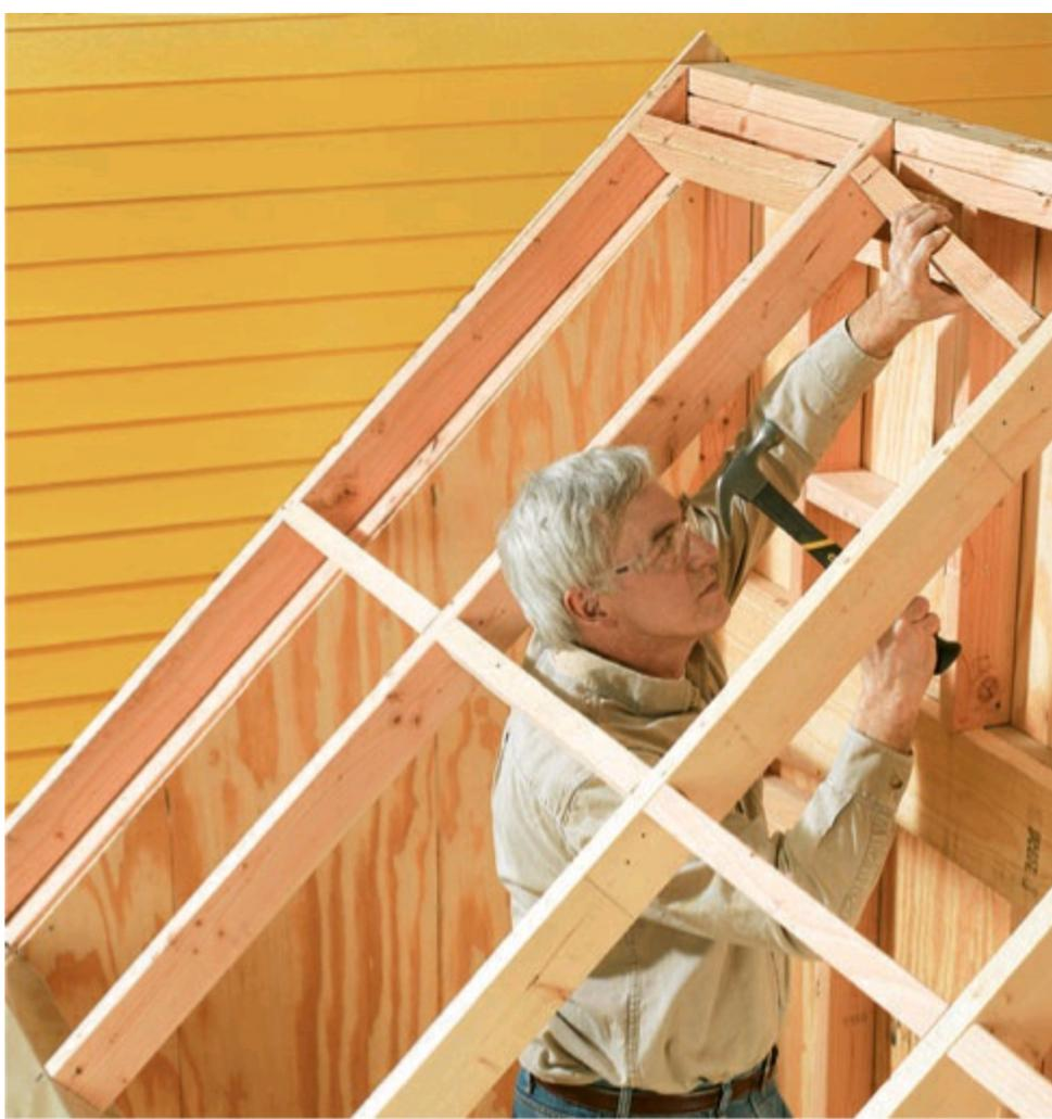
**15** Attach crosspieces between the rafters to stiffen and, support the glazing panels. Screw them in through the backs of the rafters at an angle.
