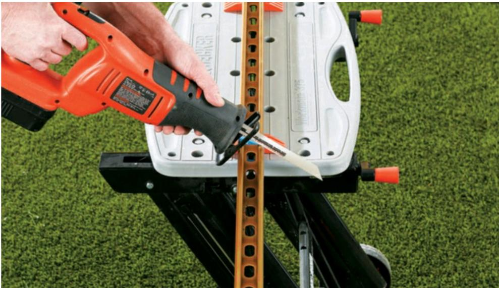
**2** Cut the pieces to length. Cut the cross supports to match the width of the solar collector or the length between mounting points on the PV panels.
