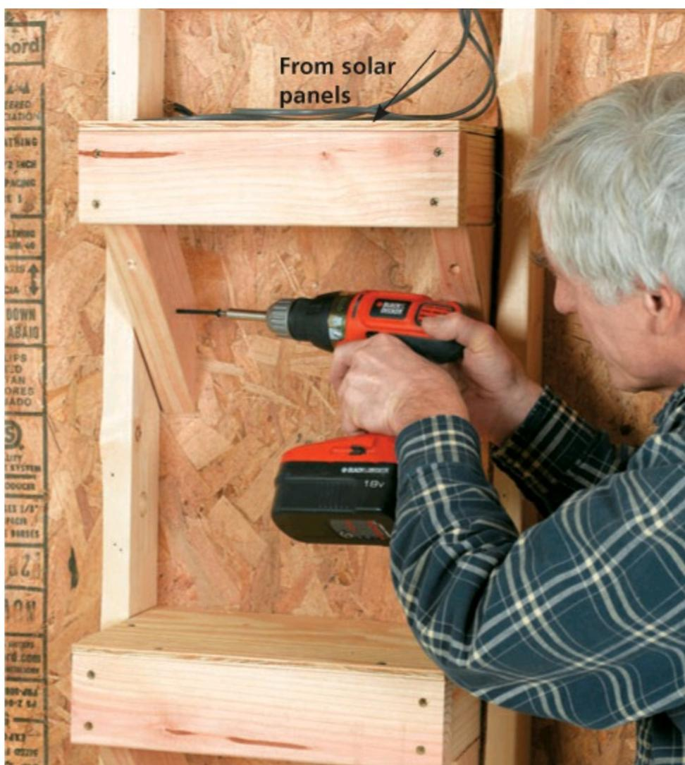
**7** Install two sturdy shelves inside the building to hold the regulator and the battery. The shelf should be easily reachable by an adult so the equipment can be turned on and off and plugged into the adapter easily. The battery shelf should be at least 18" off the ground.
