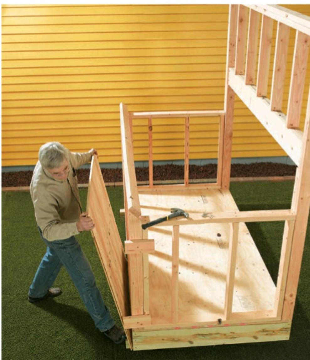
**6** Nail the exterior siding to the framing for the front wall. The top edge should be 1/2" lower than the top of the 2 × 4 framing to leave room for the glazing overhang. Nail temporary stops at the corner to help position the siding.
