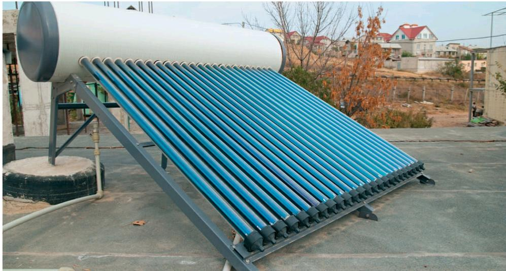
**This type of thermosyphon system** uses evacuated-tube hot water collectors and an attached storage tank at the top to provide hot water. It works well in both a tropical climate (top photo) and a cool northern climate.
