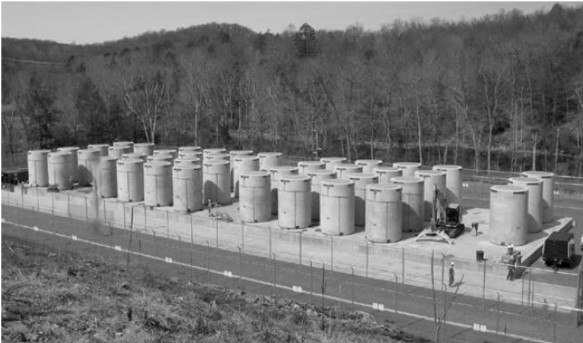
Figure 8.10 The 43 dry storage casks of the Yankee Rowe decommissioned nuclear facility. They contain 1019 spent fuel assemblies and sections of the reactor vessel
