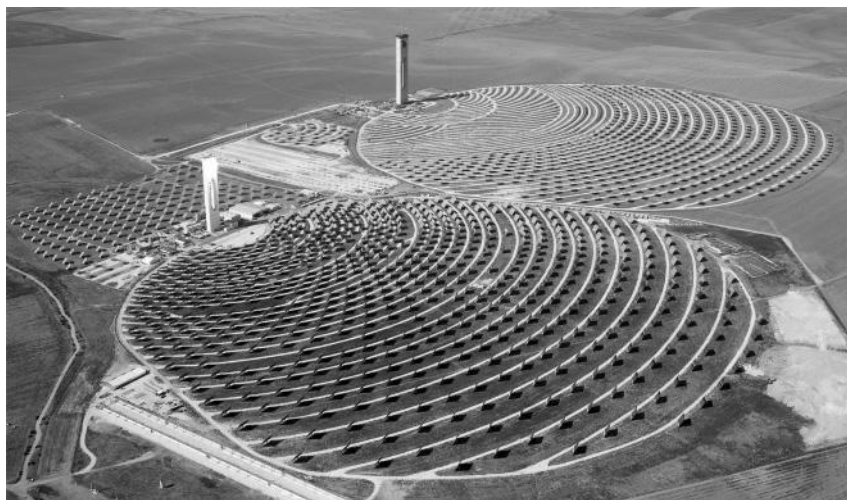
Figure 10.6 The PS10 and PS20 CSP solar tower facilities in Andalusia, southern Spain.
