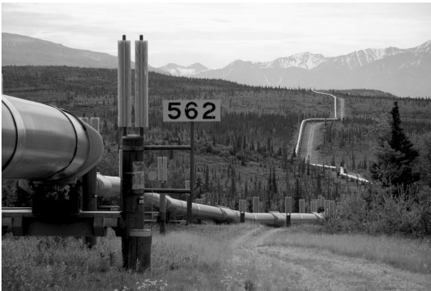
Figure 4.2 Trans-Alaska pipeline (photograph by Luca Galuzzi, www.galuzzi.it ).
