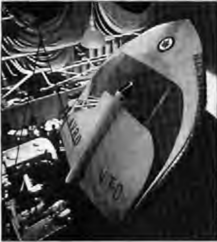
Above: A full-scale engineering mock-up of the Project Y Manta at Avro's factory in Malton, Ontario.
