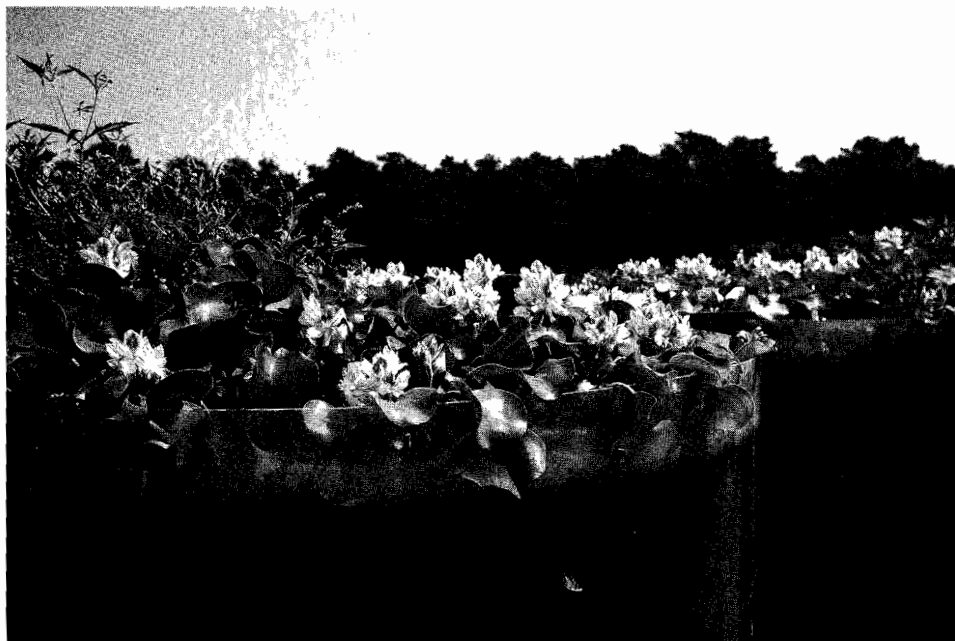
Rafted plants on the water surface of the Harwich Eco-Machine.
