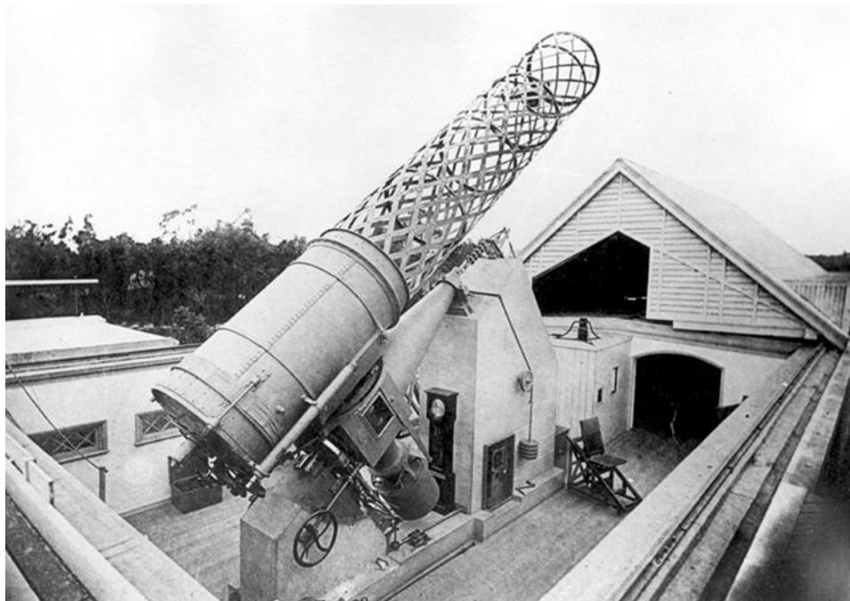
Figure 9.1. The Great Melbourne Telescope in its original incarnation. Crippled by poor design and maintenance, it had to wait decades before it made any important contributions to the science of astronomy.
