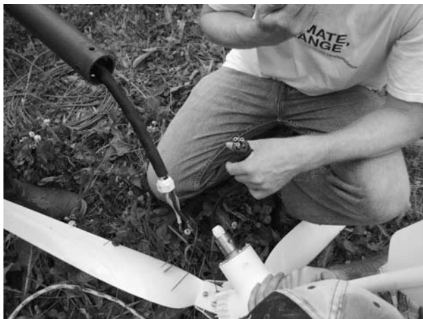
Figure 12-23 The turbine electrical connection and wire coming from the tower.
