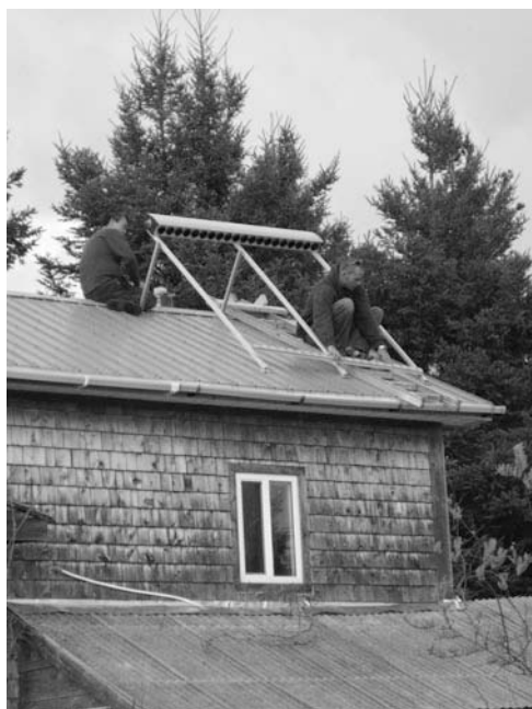
Figure 7-26 Supporting bracket for the evacuated tubes is attached to a roof-mounted frame.
