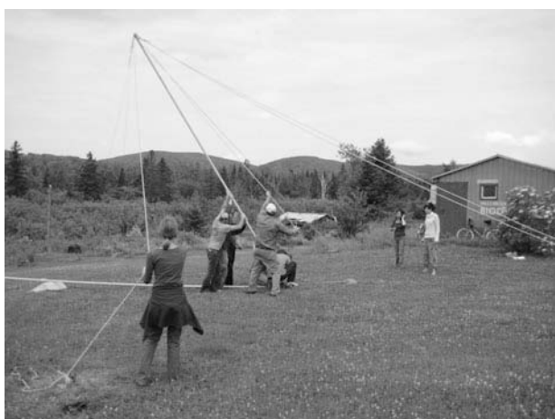
Figure 12-16 The gin pole is not actually that light, pull on the long ropes to help lift one end upright.
