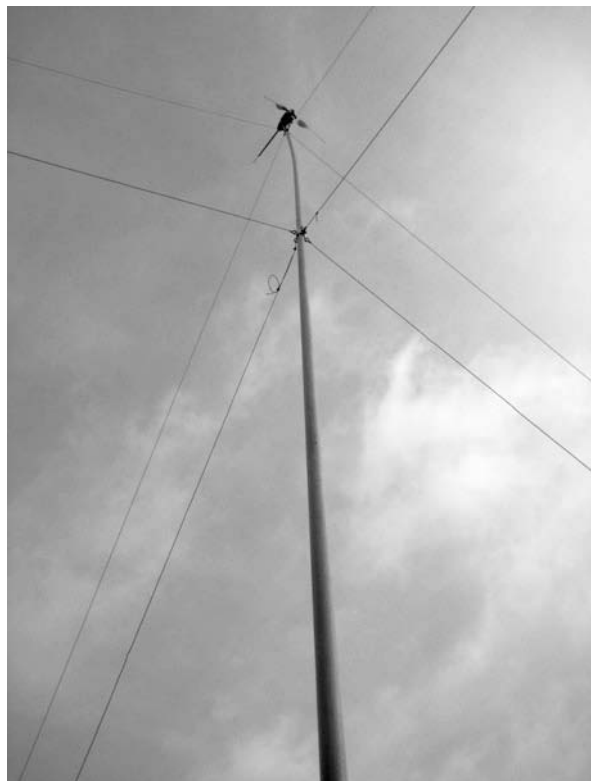
Figure 12-6 A thin tower with eight guy wires visible.
