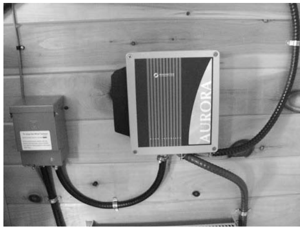
Figure 10-10 An Aurora grid-tied charge controller that is specific to the turbine shown in Figure 10-11 is connected to a net-metered system in New Brunswick, Canada.
