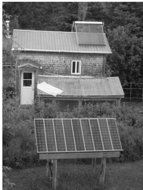
Figure 7-21 An affordable evacuated tube solar thermal collector mounted on the roof of a house in New Brunswick, and a solar electric panel on a frame on the ground in front of it. The solar thermal system is by far the more affordable option.
