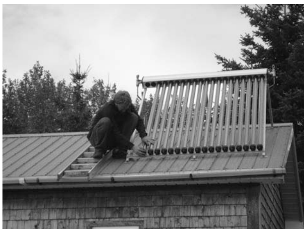
Figure 7-35 Attach the mount to the bottom of the evacuated tube.
