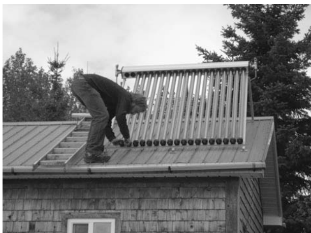
Figure 7-36 Insert mounting bolts and tighten.
