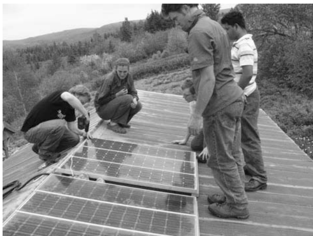
Figure 11-48 Fasten every corner into a solid part of the roof, so the wind doesn't pick them up.
