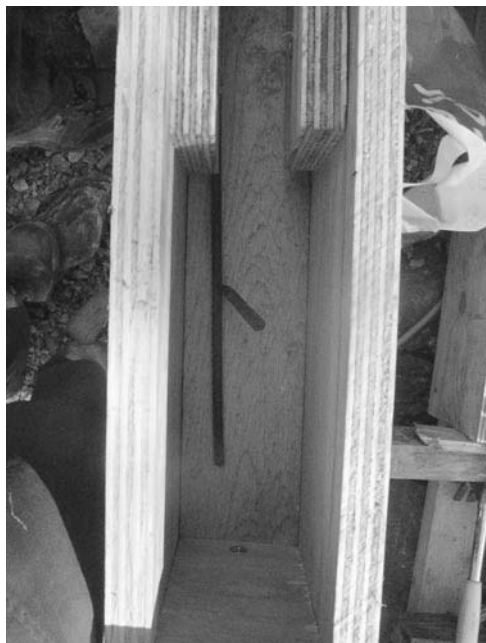
Figure 15-5 A simple wooden form can be used to create a thermally massive earth wall to store heat and cold and reduce energy costs.
