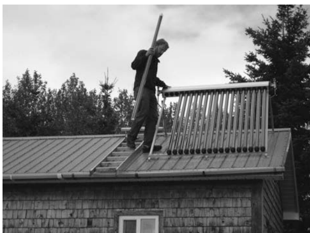
Figure 7-30 Correctly orient the tube so the thin end (where the fluid emerges) will fit up into the heat exchanger.
