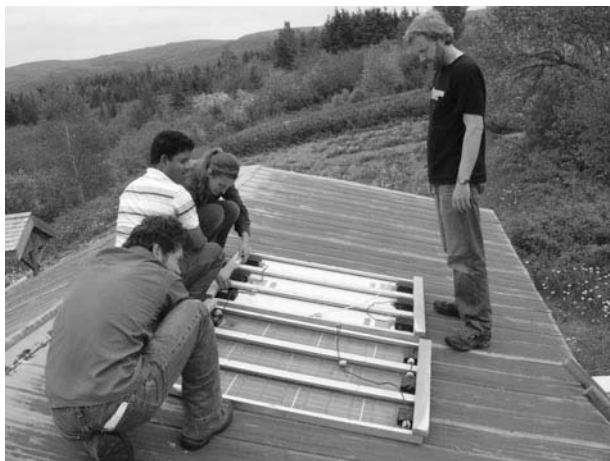
Figure 11-36 Lay out the panels so that the electrical connections are accessible.
