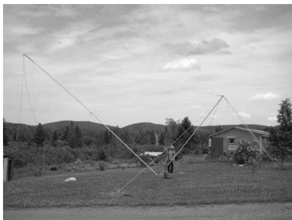
Figure 12-19 With the ropes attached, the gin pole is used to raise the tower.
