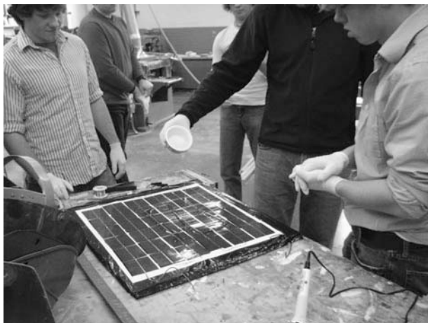
Figure 11-20 Pouring silicon onto the wired module.
