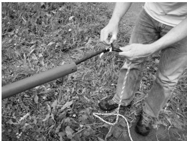
Figure 12-22 Attaching the wire to a guide rope.
