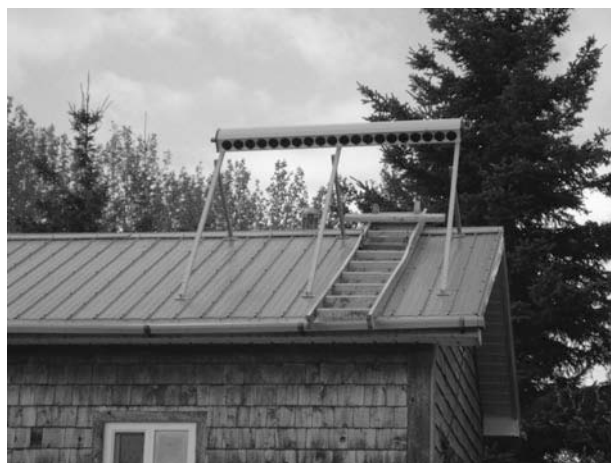
Figure 7-23 Parts of an evacuated thermal collector frame mounted on a roof of a house, not quite ready for the tubes to be installed.
