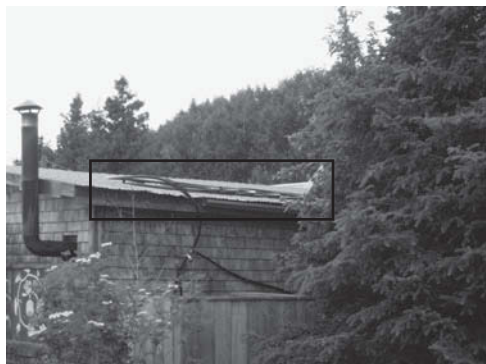
Figure 7-8 A low-cost batch water heater that holds enough water in the coils of black plastic tubing on the roof to provide one or two outdoor showers at the end of a hot day. Photo taken at the Falls Brook Centre, Canada.
