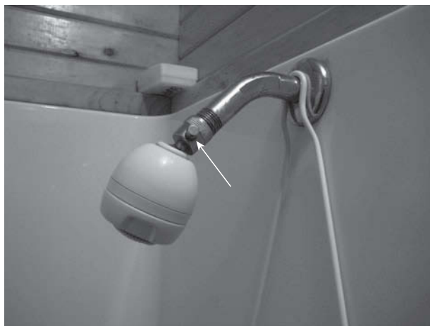
Figure 6-10 A low-flow showerhead installed. The on-off control is arrowed.
