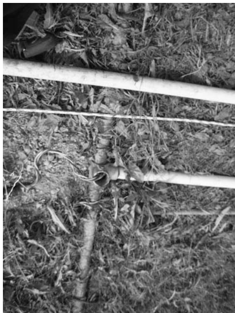
Figure 12-9 The hinge line (vertical tube) held in place by a U-shaped rebar. The mast (down) forms a T going off to the right. The gin pole lies, detached, horizontally across the photo, just below the second U-shaped bracket. The electrical connection wires are visible where the gin pole and tower meet in the center of the image.
