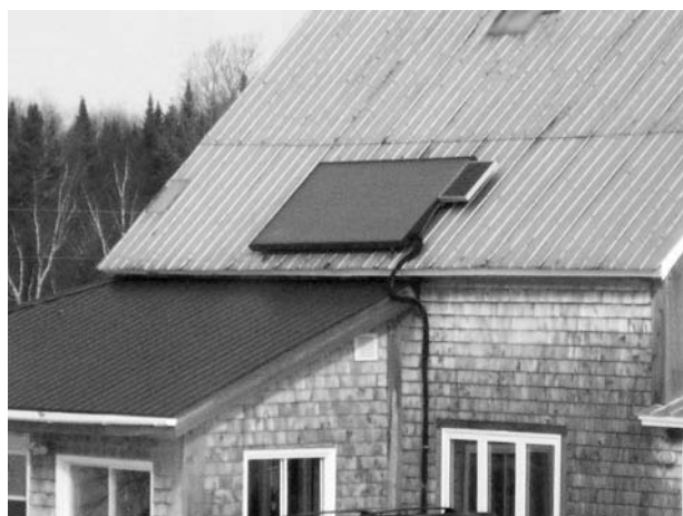
Figure 7-10 Professionally installed solar hot water system in New Brunswick. The small electric panel to the right on the large thermal panel powers a pump which circulates fluid through the collector and into the tank inside. The flat-plate collector is similar to the ones built in the upcoming project.
