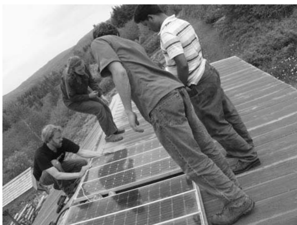
Figure 11-47 On flat roof installation, your panels are not going to have that many forces acting on them, but they shouldn't move around.
