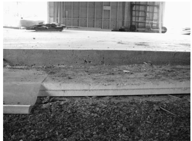
Figure 3-13 Thermally massive concrete flooring being installed on top of a layer of insulation in a geothermal (earth as a source of heat) building, described more later in the book.
