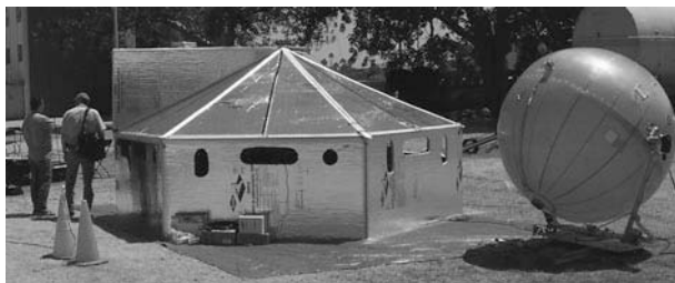
Figure 15-12 The hexayurt—an open-source environmentally responsive building technology that costs little to build and can be constructed quickly.
