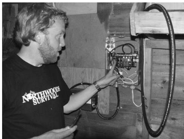
Figure 10-14 The door of the fuse box of the above system, open while attaching the solar electric panels from Chapter 11. Brent Crowhurst from the Falls Brook Centre is pictured.
