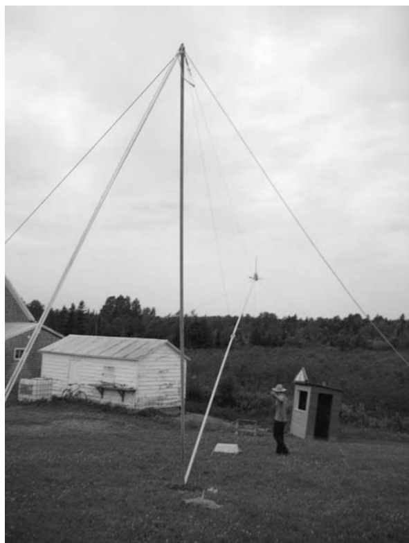
Figure 12-7 Lowering a tower with a removable gin pole.
