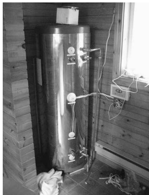
Figure 7-38 Solar hot water tank, before plumbing from the thermal collector is installed.
