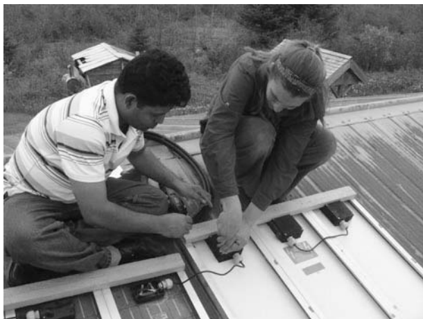
Figure 11-37 Connect the two modules together.
