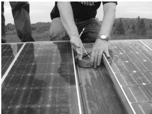
Figure 11-41 Securing the junction box.
