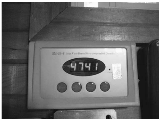
Figure 7-20 Temperature sensors in the tank feed data to this computer, which then turns circulation on only when the sun is shining, and turns on the electric heater only when needed.
