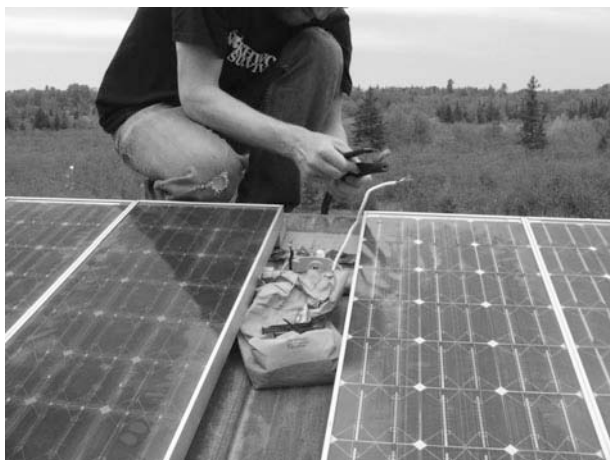
Figure 11-42 Strip the end of the cable that will carry the electricity to the battery or charge controller.
