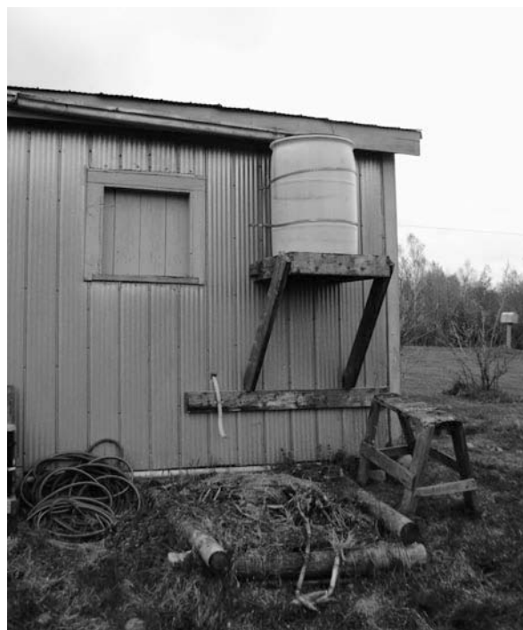
Figure 6-11 A rainwater collection barrel mounted on the back of a workshop at the Falls Brook Centre, New Brunswick. The soak below the barrel catches the oily particles from the biodiesel workshop's gray water waste.
