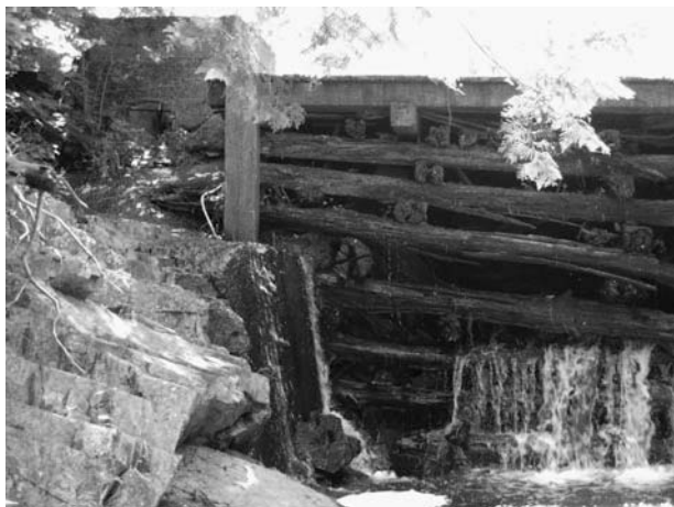
Figure 8-1 An old dam outside Florenceville, New Brunswick, which once powered a sawmill using a large water wheel. The wheel was fed through the chute, barely visible in the top left corner of the photograph.
