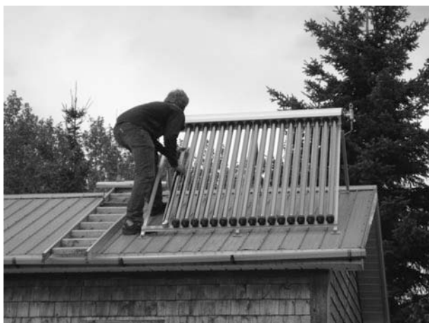
Figure 7-33 Grasp the tube firmly and slide straight up into place.
