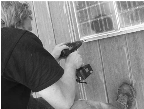
Figure 11-46 Drilling this close to the panel isn't really advisable, but is sometimes necessary. Be careful.
