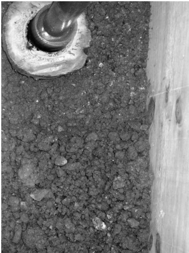
Figure 15-8 Ramming earth into a wooden framework to create the earth wall shown in Figure 15-7.
