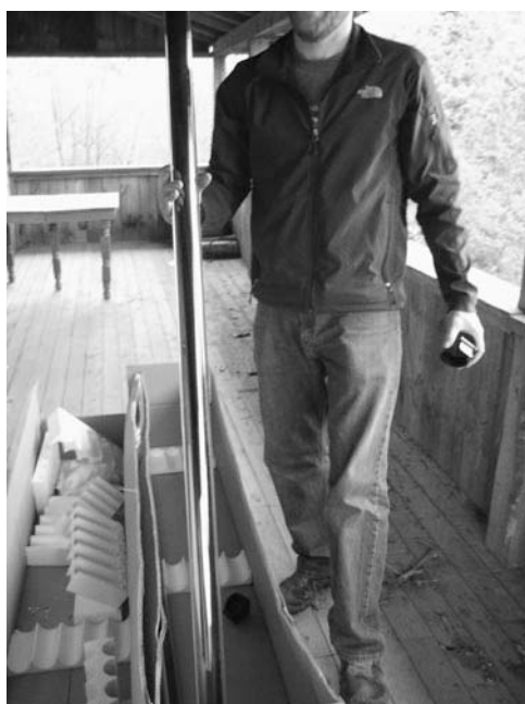
Figure 7-28 Gently lift the evacuated tube from the box.
