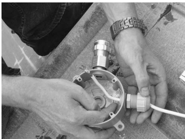
Figure 11-40 Feed the wires from the panels into the junction box.
