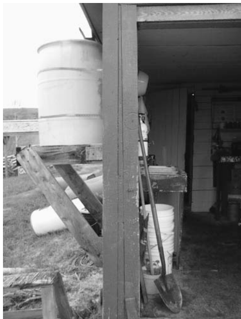
Figure 6-12 View of the rainwater barrel (left) outside and sink (right) inside the workshop. The bottom of the barrel is only slightly above the sink tap, but provides more than enough pressure for washing up.
