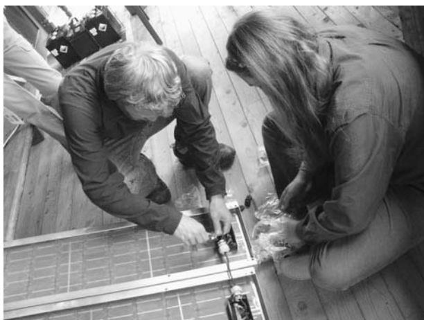
Figure 11-30 Tightening the weatherproof covers onto the second connection.
