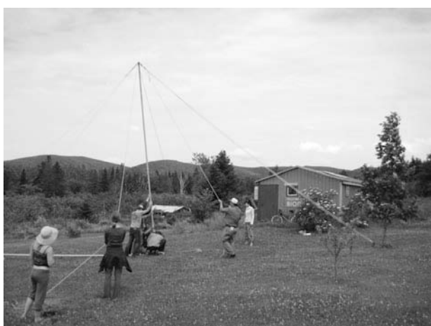
Figure 12-17 In this position, it is important to make sure the electrical cable is not pinched, which can require lifting the pole straight up.
