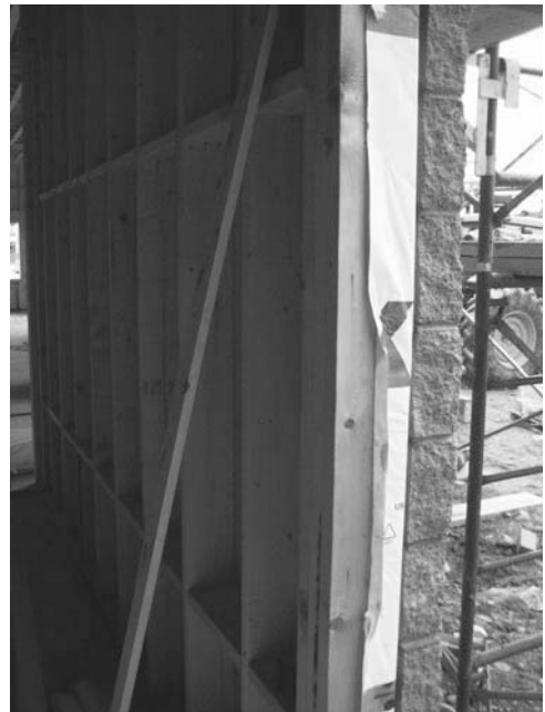
Figure 3-17 Cavities left for the insulation along the inside are visible, along with the thermally massive outside wall. Heat radiating from the thermally massive floor (see Figure 3-13) will be trapped by the insulation, and any heat getting through will first have to heat the brick wall before escaping.
