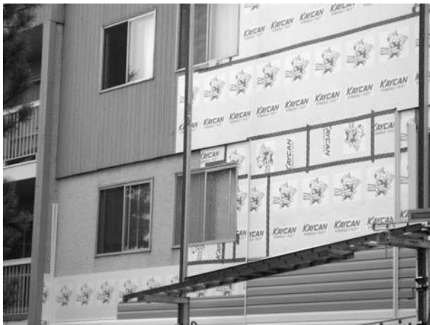
Figure 3-16 Insulation and siding being retrofitted over a top of a layer of heavyweight material, on an apartment structure that is constantly heated and occupied.
