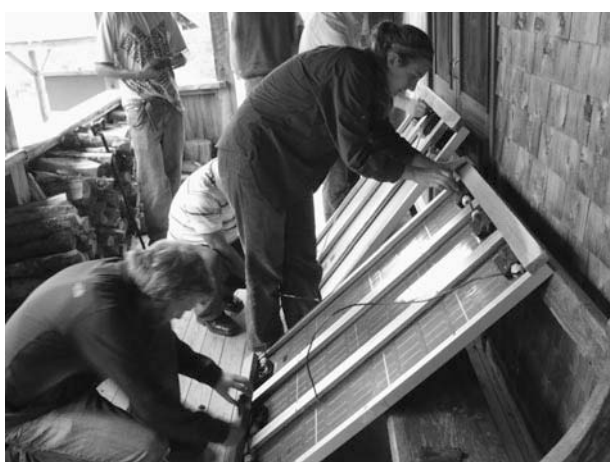
Figure 11-32 The wooden frames holding the three modules together are being installed.
