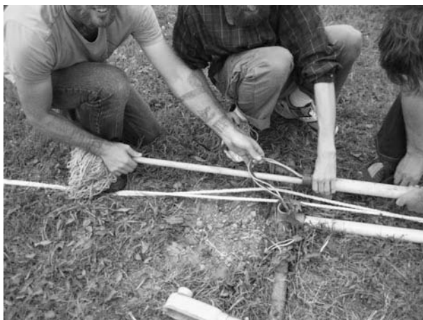
Figure 12-21 Using a special tool to gently push the electric wire up the tower.
