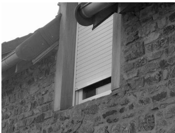
Figure 3-9 Roll down shutters can be automated to close at certain times.
