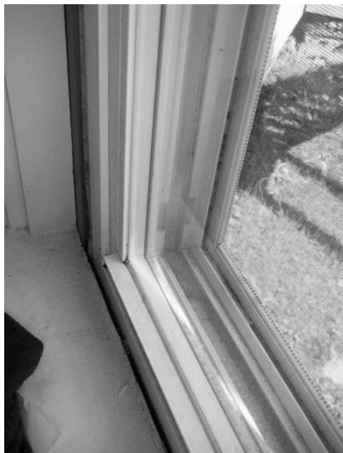
Figure 3-11 Newer-style airtight double-pane windows.
