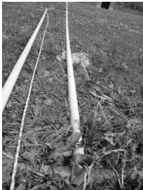
Figure 12-13 The gin pole (left), mast (center), and wire stuffing tool (right), with the hinge line and electrical connections visible at the bottom.
