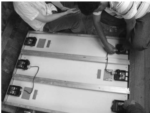
Figure 11-31 Securing wires on a second set of three modules to be installed.
