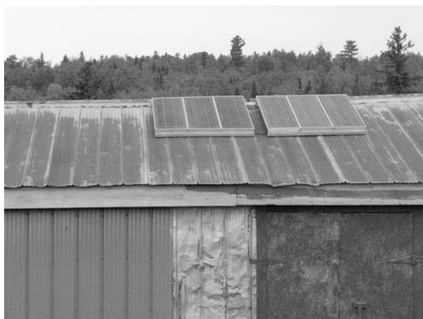
Figure 11-54 The mounted PV modules, producing clean electricity!
