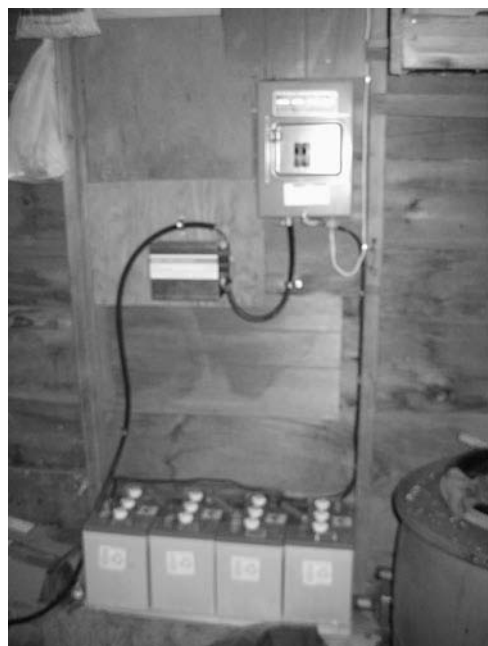
Figure 10-13 Flooded lead-acid batteries on the floor of this educational setup at the Falls Brook Centre, New Brunswick. The small charge controller and fuse box are mounted on the wall above.
