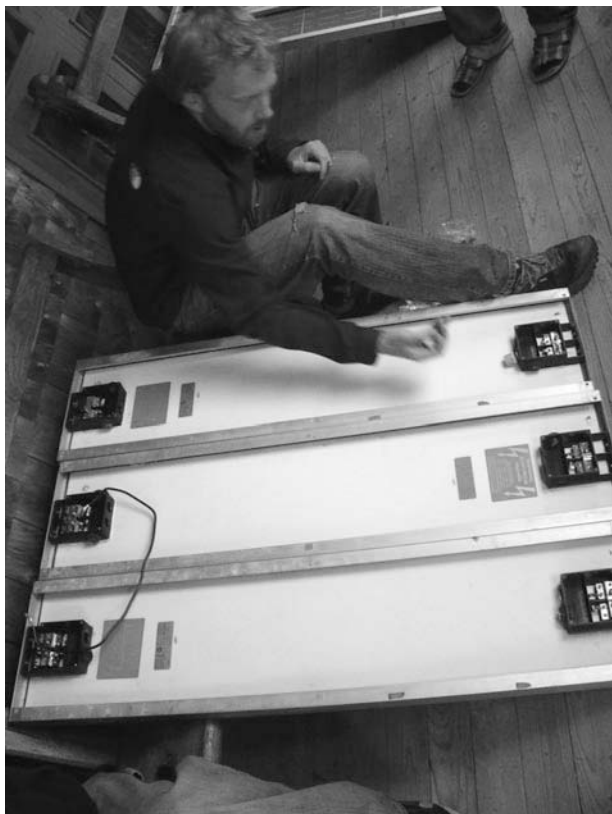
Figure 11-29 Three modules set alongside one another; the first cable wiring them together is in place.
