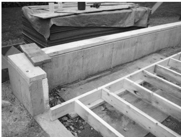
Figure 15-1 A heavy concrete foundation beneath a lightweight wooden wall construction is a common building technique. If well-insulated, this method of construction can produce buildings that are efficient.
