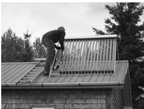
Figure 7-32 Slide the evacuated tube into the mounted heat exchanger.
