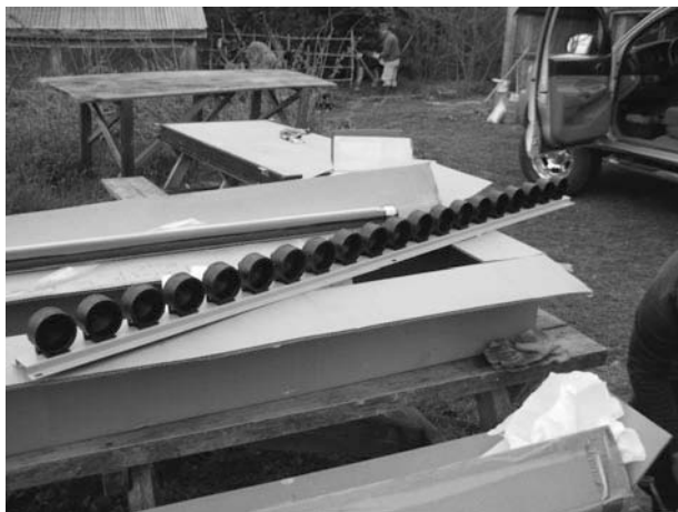
Figure 7-27 Lower support member of the evacuated tubes, ready to be lifted onto the roof.
