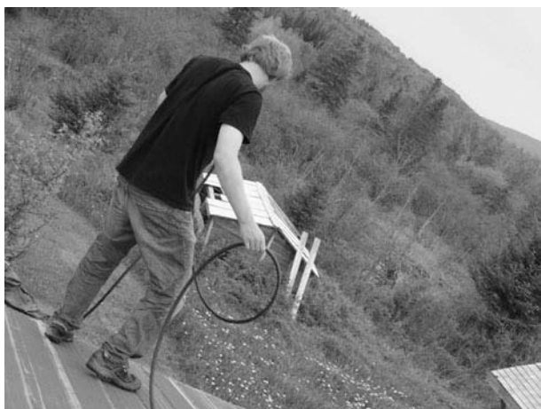
Figure 11-52 The cable should be fed out of the way, but on the shortest path possible to avoid losses.
