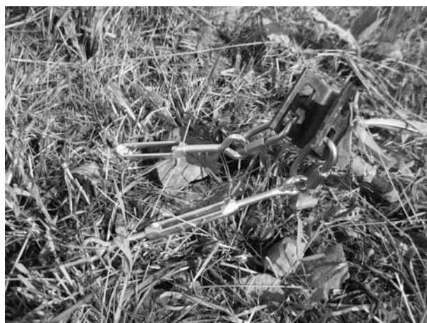
Figure 12-8 The rubble holding the anchor underground and the steel connection point with turnbuckles.
