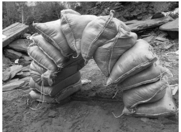
Figure 15-10 A sandbag arch. Note how there is one central bag, directly in the middle, which forms an almost triangular shape. This is called the locking bag, because it locks the arch into a sturdy form.
