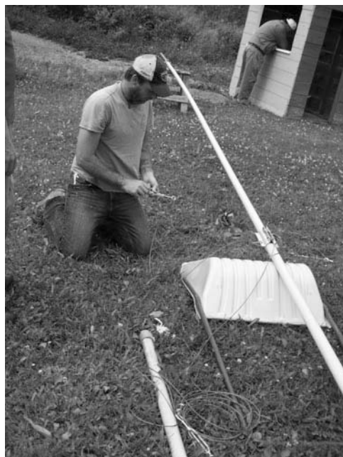
Figure 12-10 With the tower laid out, start by attaching cables.
