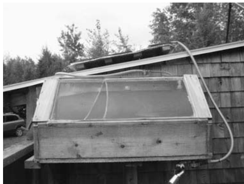
Figure 7-7 A batch solar hot water heater, with a metal tank inside an insulated box functioning much like a solar cooker, feeding an outdoor shower (the cracked glass is about to be replaced).
