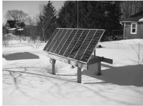
Figure 11-1 Frame-mounted solar electric modules at the Falls Brook Centre, Knowlesville, New Brunswick.
