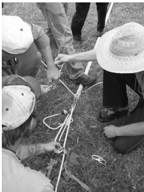
Figure 12-27 Moving the cable from the gin pole to the lift anchor.
