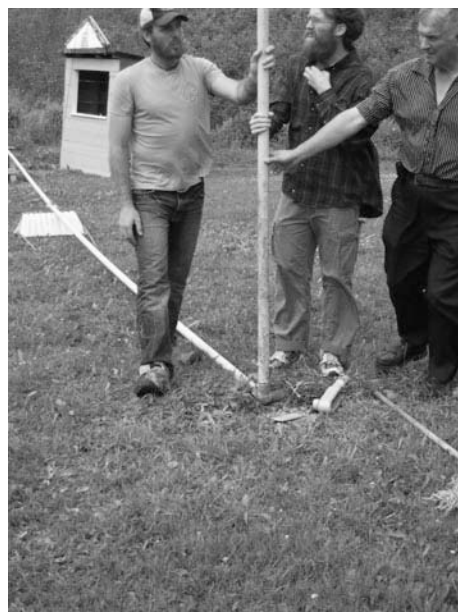
Figure 12-18 The gin pole installed.
