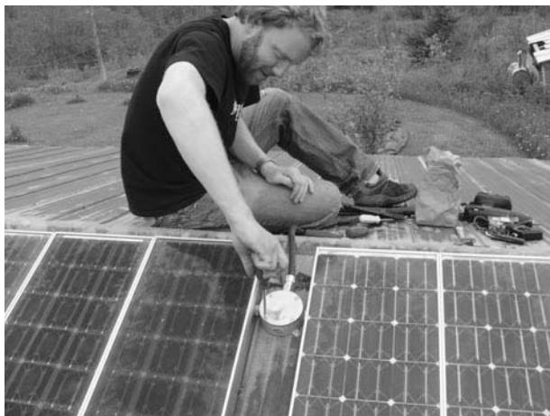
Figure 11-51 Rain is bad for electronics. Fasten the junction box cover tightly.
