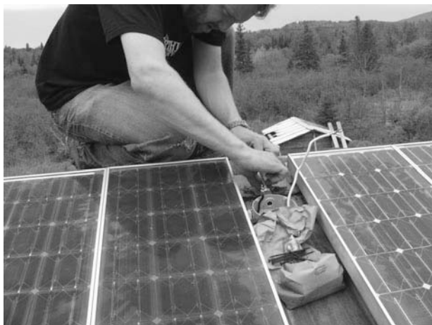
Figure 11-43 Feed the thick cable into the junction box.
