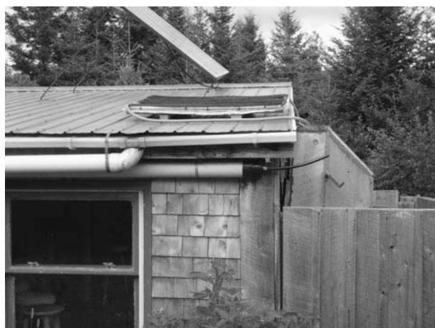
Figure 7-24 The homebuilt solar thermal panel from the previous project. It has been simply mounted in a more permanent place on a roof as a supplementary heater for a shower.
