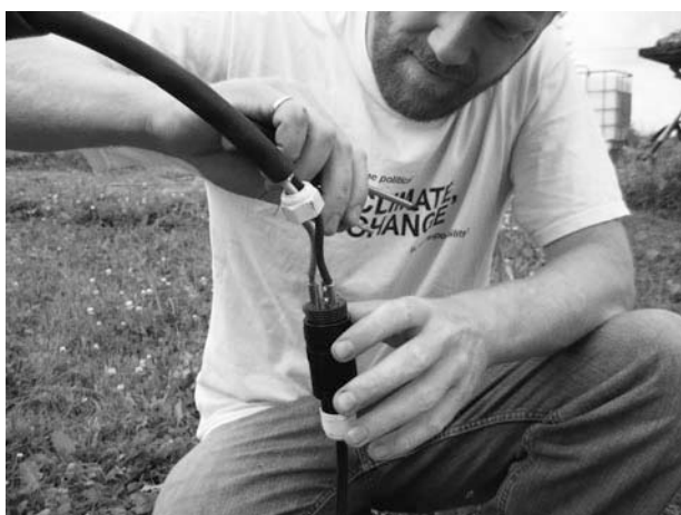
Figure 12-24 Connecting the turbine to the wire feeding down the tower.
