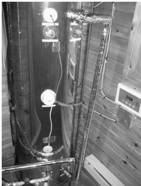
Figure 7-19 An individual family-sized solar-electric hot water heater; installed. The electric element is midway up the tank, fed by electric cables from the right.
