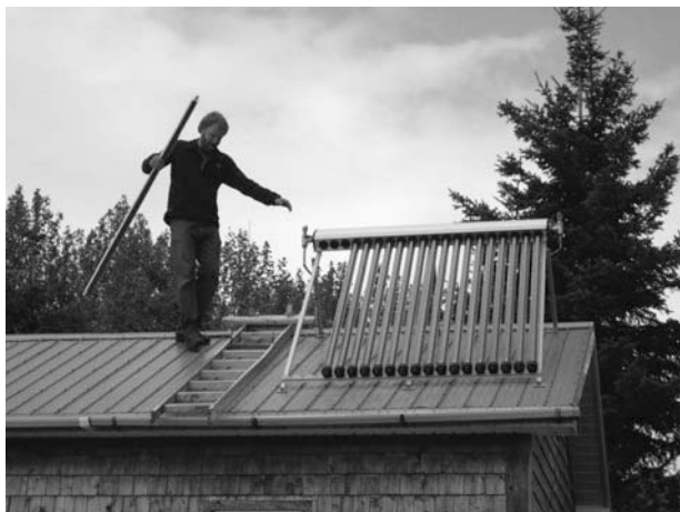
Figure 7-29 Carry the evacuated tube onto the roof, holding it away from sharp objects that could shatter the glass.
