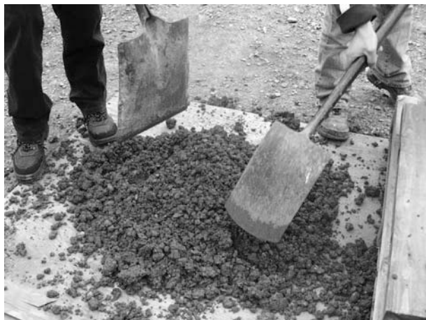
Figure 15-4 Mixing earth on a cardboard plank.
