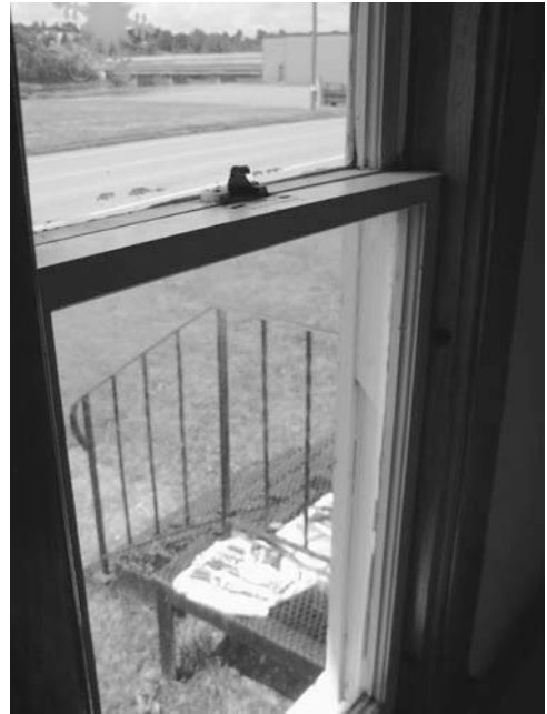
Figure 3-1 Old single-pane windows with many gaps around the edges visible. Keep reading for both long- and short-term improvements if they look familiar to you.
