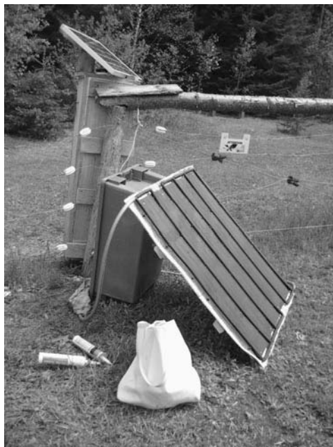
Figure 7-16 The homemade solar collector in action! It has been painted black and has some (reclaimed hot water tank) insulation behind it. The tank is kept (out of the sun) in the container doubling as a stand, and the pump is powered by the solar panel mounted on the fence behind.
