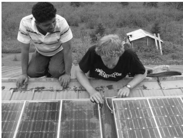
Figure 11-38 Easy for wires to get into inconvenient places, so make sure the important ones are accessible.
