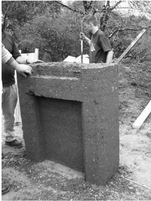
Figure 15-7 A rammed earth wall built as an educational experience by students at the Centre for Alternative Technology, in Machynlleth, Wales.
