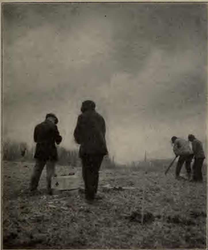
SHATTERING SUBSOILS WITH FARM POWDER
