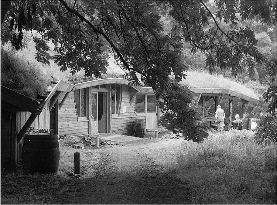
*While roofs shelter building occupants, they rarely have a beneficial effect on local outdoor climate. Vegetated roofs, however, can absorb airborne toxins, redress oxygen, ion and humidity balances. Even more importantly, they reduce flood risk by spreading rainwater discharge over a day instead of minutes.*
